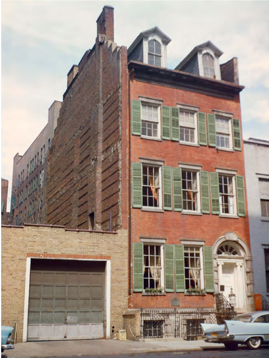
1960'S LOT LINE WALL CONDITION
