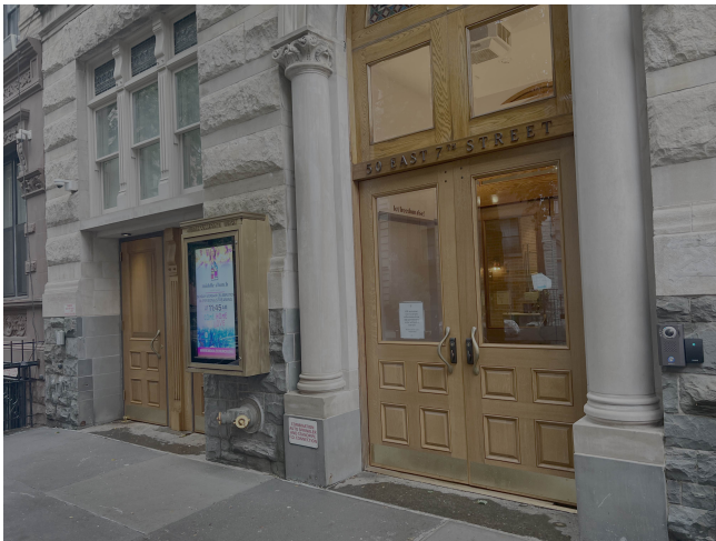
EXISTING ENTRYWAY @ 50 E 7TH ST (NO WORK)
