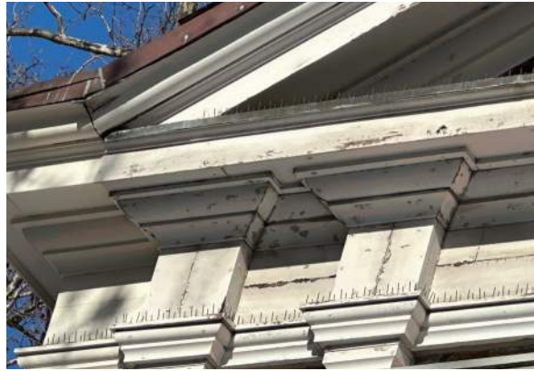
A13-1 - FINISH REPAIR WORK AT WOOD CORNICES AND PEDIMENTS ON NORTH AND SOUTH SIDE OF SANCTUARY
