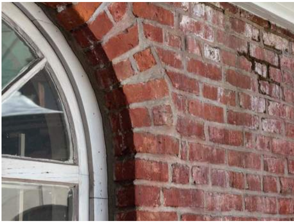
A10-1 - REPAIR CRACKED BRICK MASONRY AT PARISH HALL FACADES
