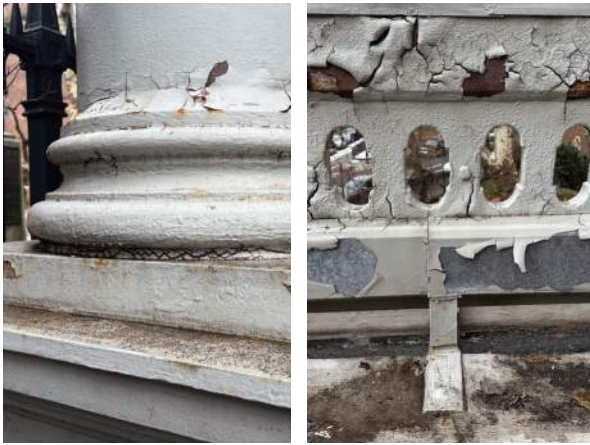
A12-1 - REPAIR AND REFINISH CAST IRON PORTICO
