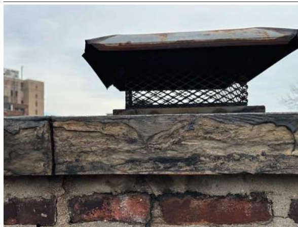
A15-3 - INSTALL WEATHER-RESISTANT CHIMNEY CAPS
