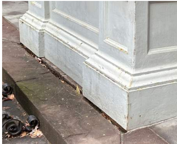
A17-2 - RESET DISPLACED CURBS AT PORTICO
