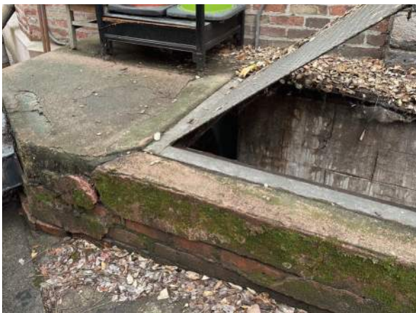
A17-1 - REPLACE AREAWAY VAULT DOORS AND CURB
