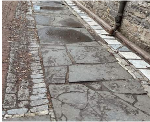
A53 - REPAIR SITE PAVING TO PARISH HALL
