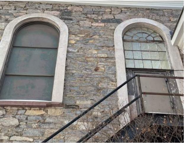
An exterior stair was added for egress from the second floor ballet studio. An original window was modified to accommodate for the door.
