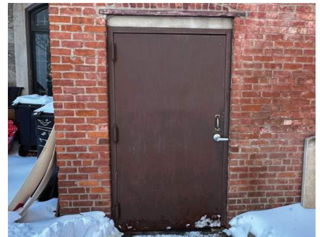
The Parish Hall first floor exit door is mismatched to the historic character of the building, and has deteriorated.
