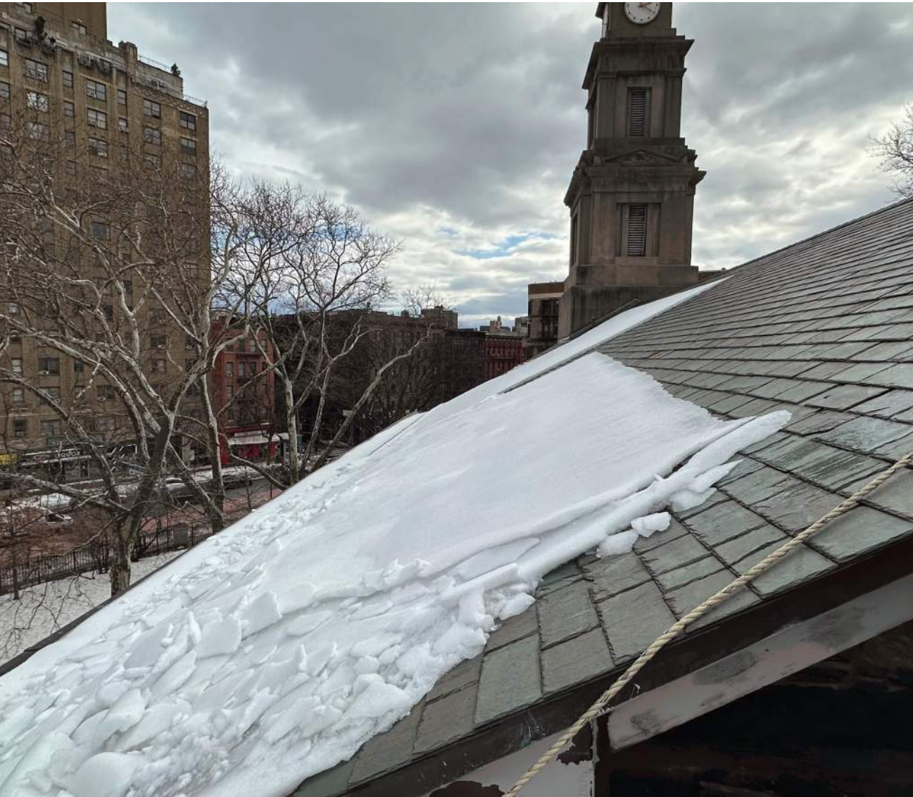
The slate roof of the church is in fair condition, and active leaks were not observed in the attic below. The Church has attic stock tiles and completes repairs periodically as needed.
