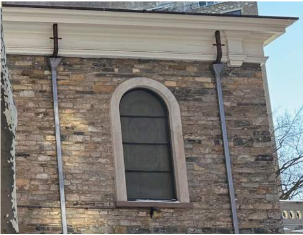
Copper downspouts were replaced with the gutter restoration project in 2023. External leaders extend to drainage boots below but are frequently stolen.
