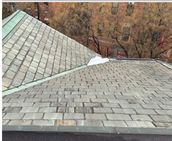
A34 - REPLACE SLATE ROOFS
