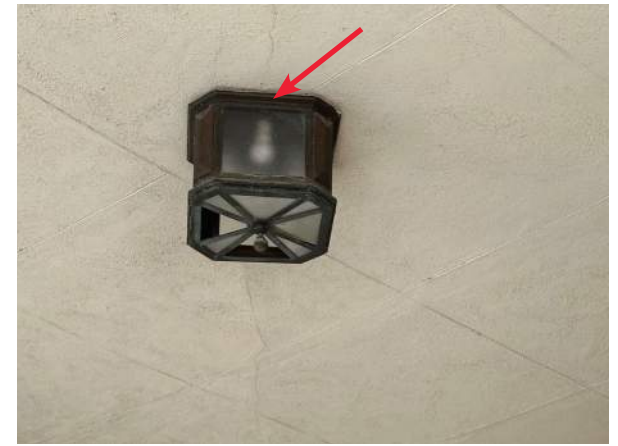
A11-2 - REPAIR CRACKS AT PORTICO CEILING STUCCO
