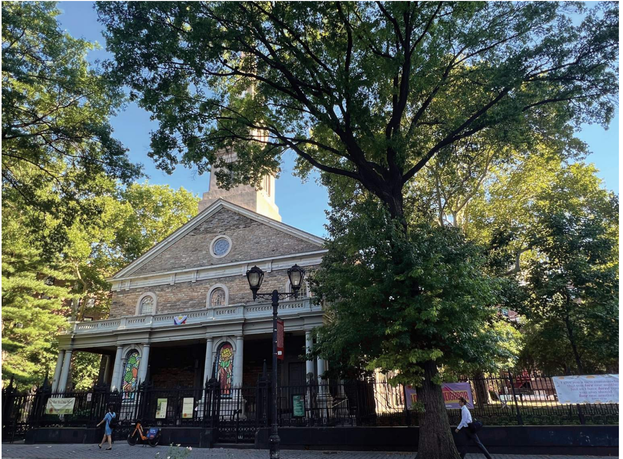
ST. MARK'S CHURCH IN-THE-BOWERY | 75-42 CONTINUING MAINTENANCE AGREEMENT
