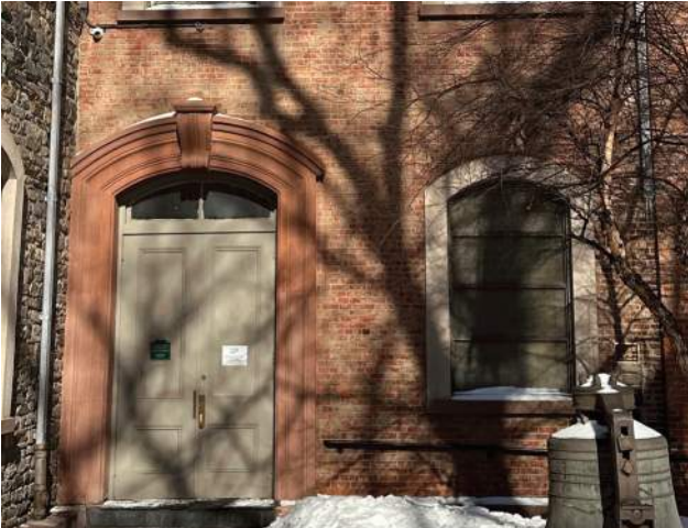
The Parish Hall south facade hosts its main entry door from the yard, a stained glass window and operable windows at the Second Floor.
