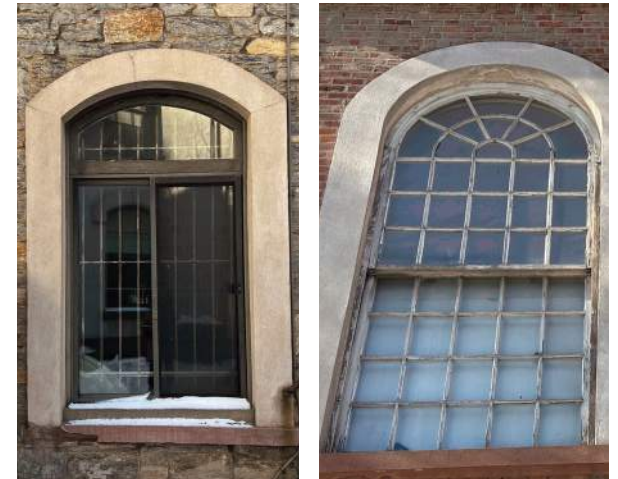
A16-1 - REPAIR DETERIORATED WINDOWS
