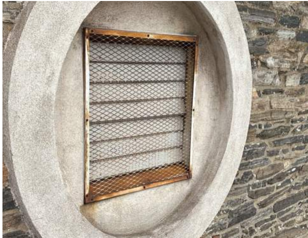
The Church attic vent louver at the north pediment does not reliably resist weather, has a rusted frame, and is mismatched to the style of other church louvers.
