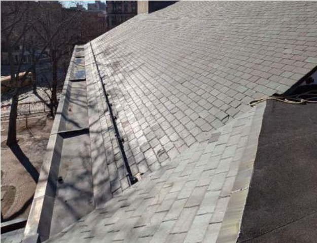
Gutters were installed in 2023 and are in excellent condition. Drains were reported to be blocked with debris in past years, and should be cleaned bi-annually.
