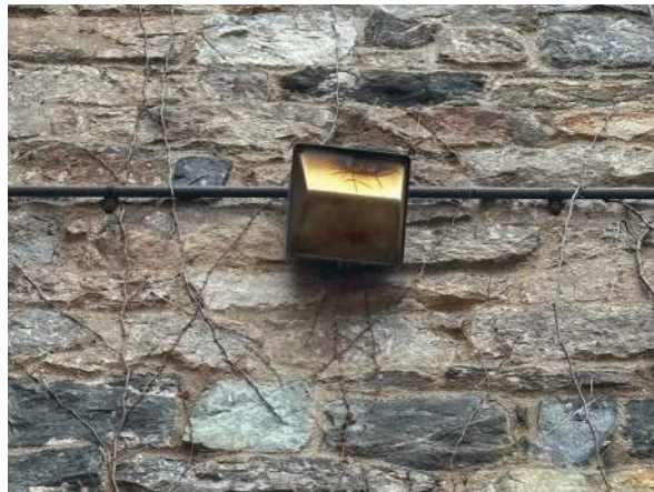
A54 - REMOVE NON-FUNCTIONING LIGHTING AND CONDUIT
