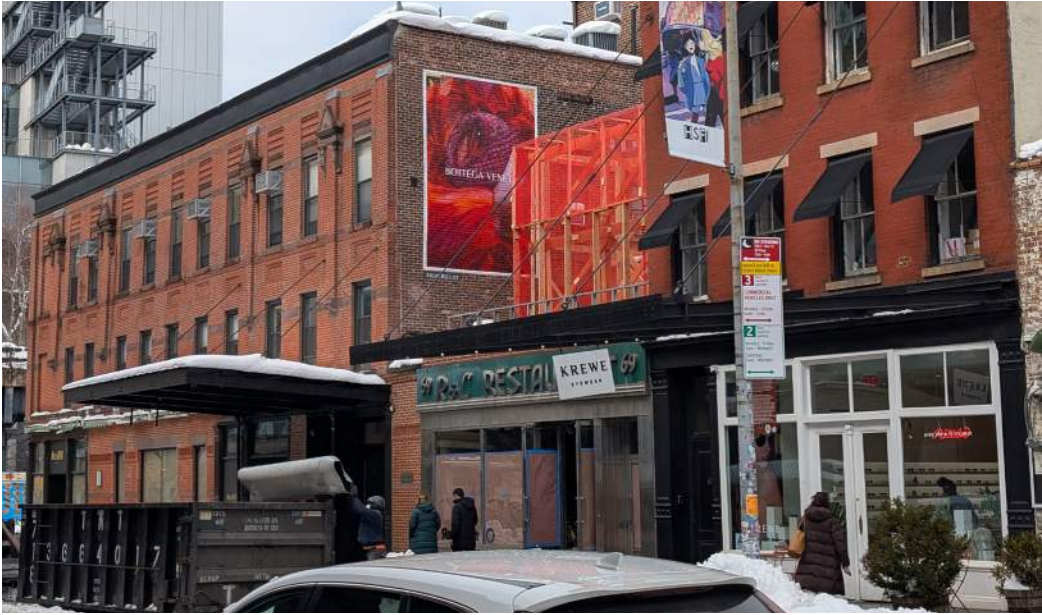
2 | MOCKUP FROM THE EAST
