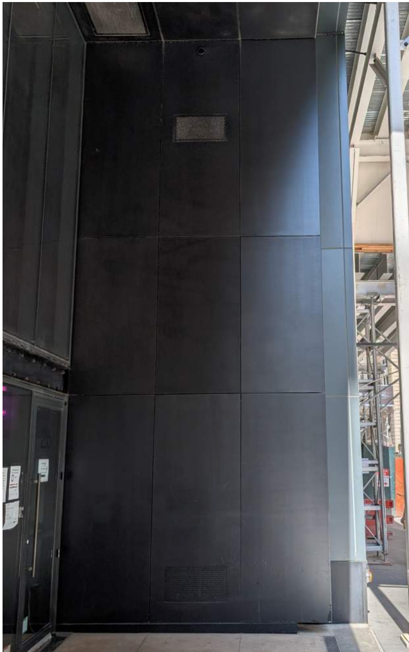
EXAMPLES OF DARK GRAY MOTTLED METAL PANEL RAINSCREEN FACADE WITH 1/8" GAP BETWEEN PANELS
