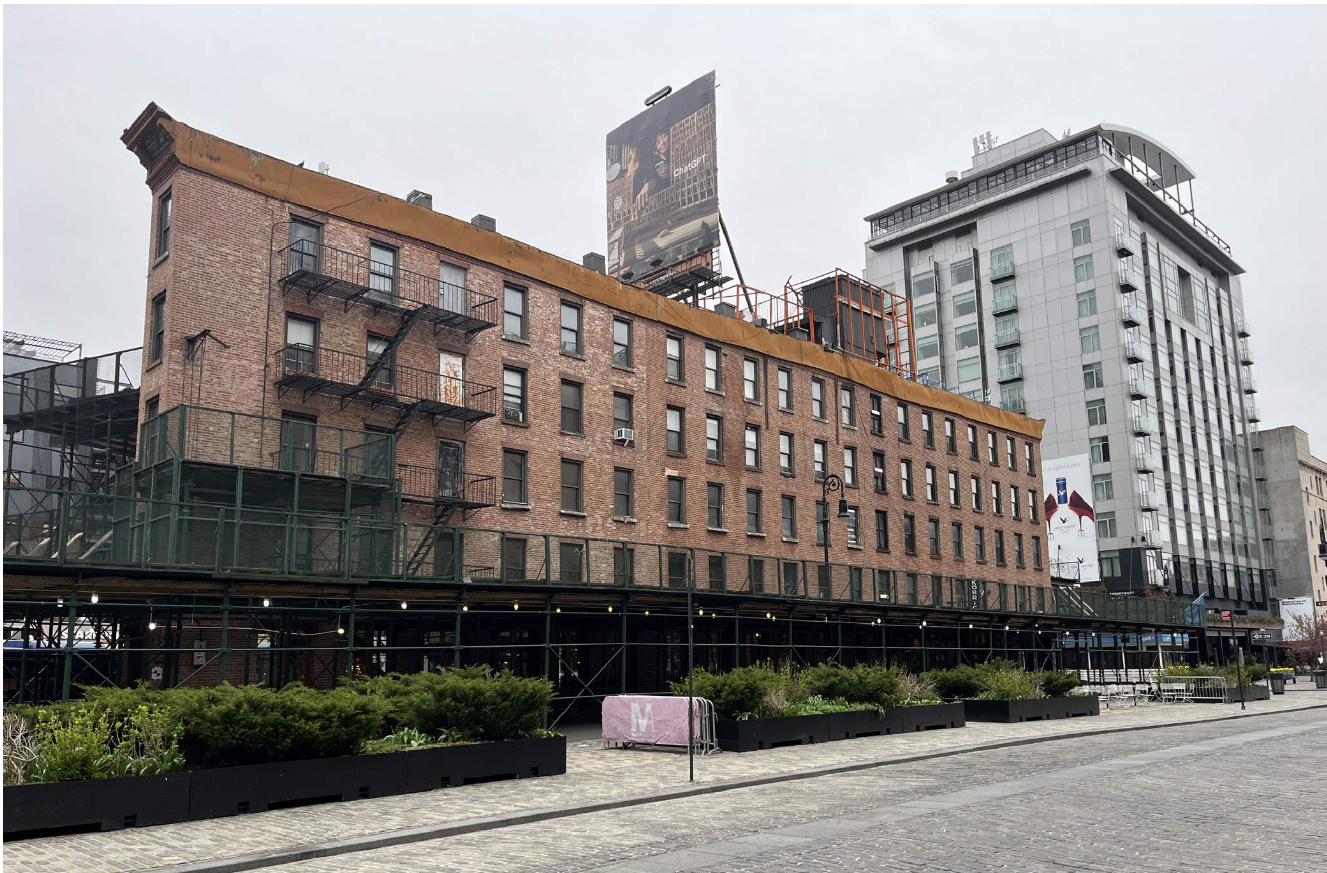
VIEW ON NINTH AVE LOOKING SOUTH
