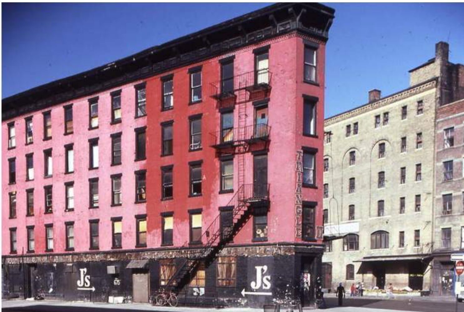
HUDSON STREET ca. 1990 (Village Preservation)
