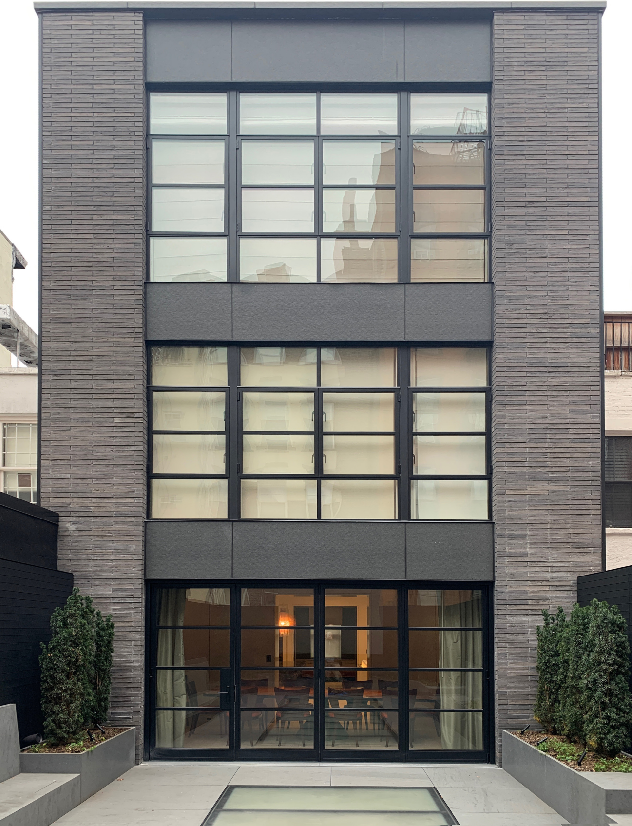
46 MACDOUGAL ST REAR FACADE
