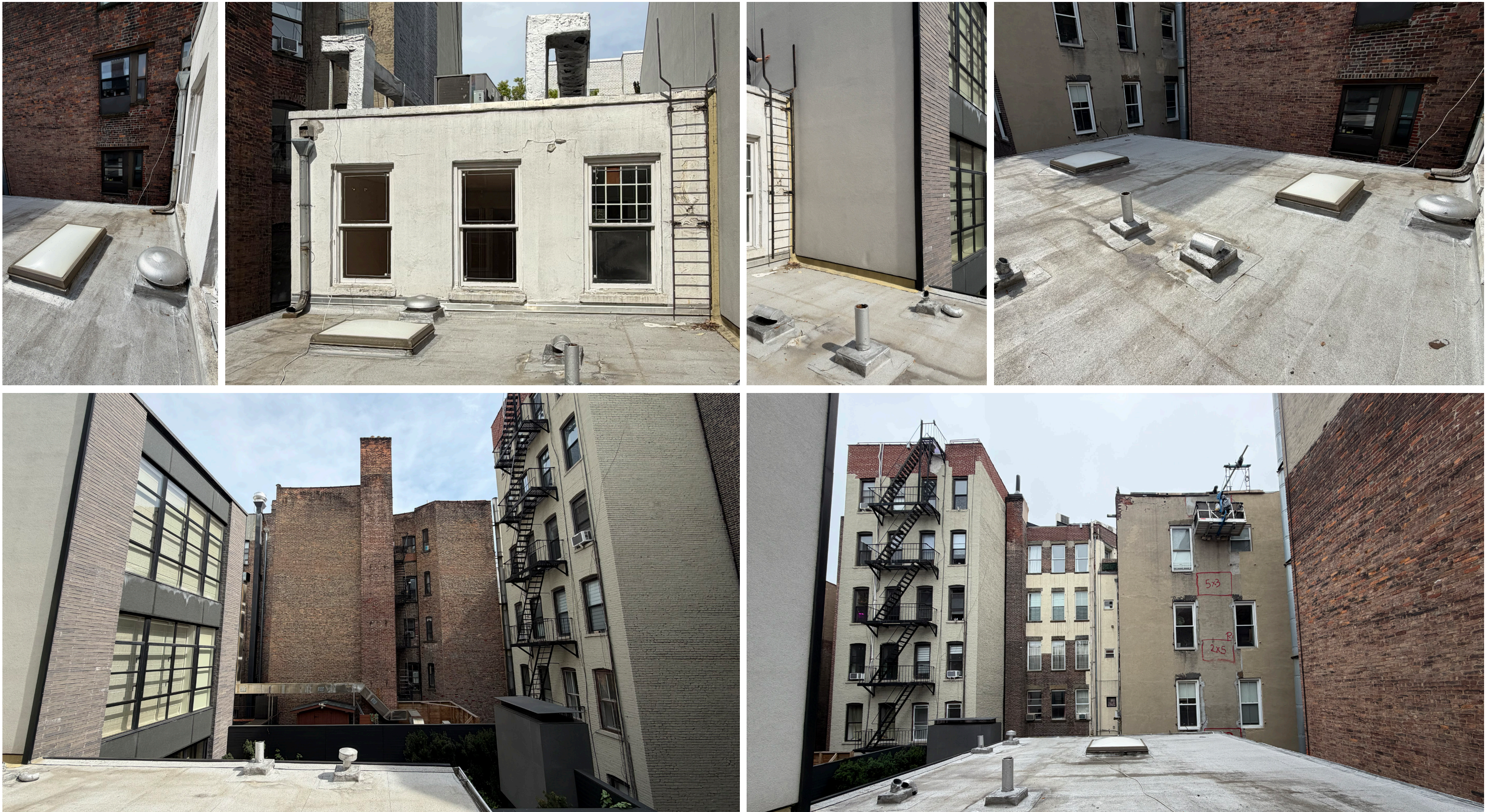
PHOTOS STANDING ON 3RD FL REAR TERRACE
