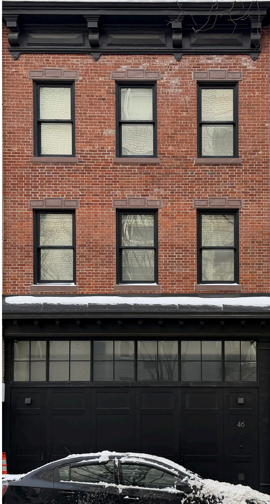
46 MACDOUGAL ST FRONT FACADE
