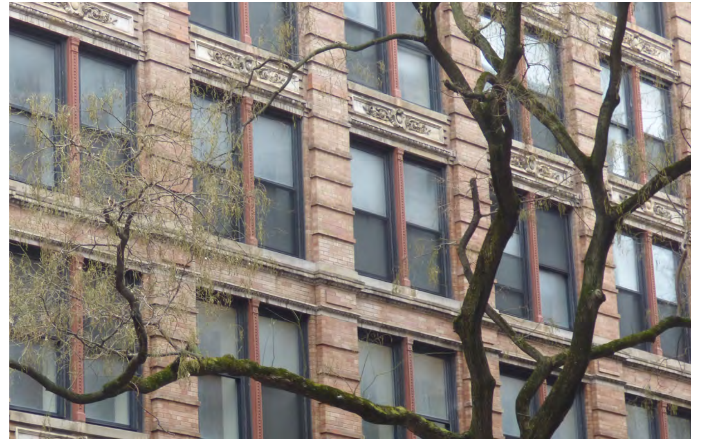
Window Details, Mott Street facade
