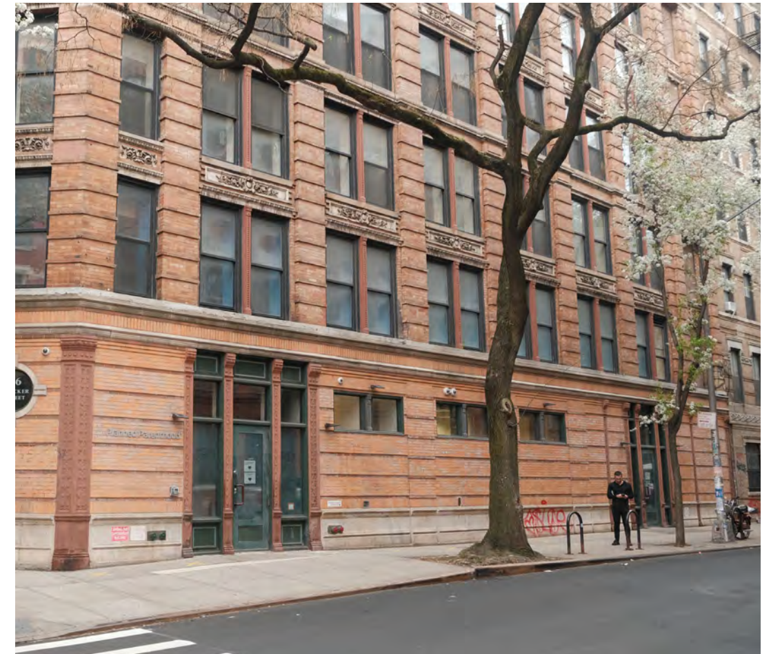
Mott Street Elevation, facing southeast
