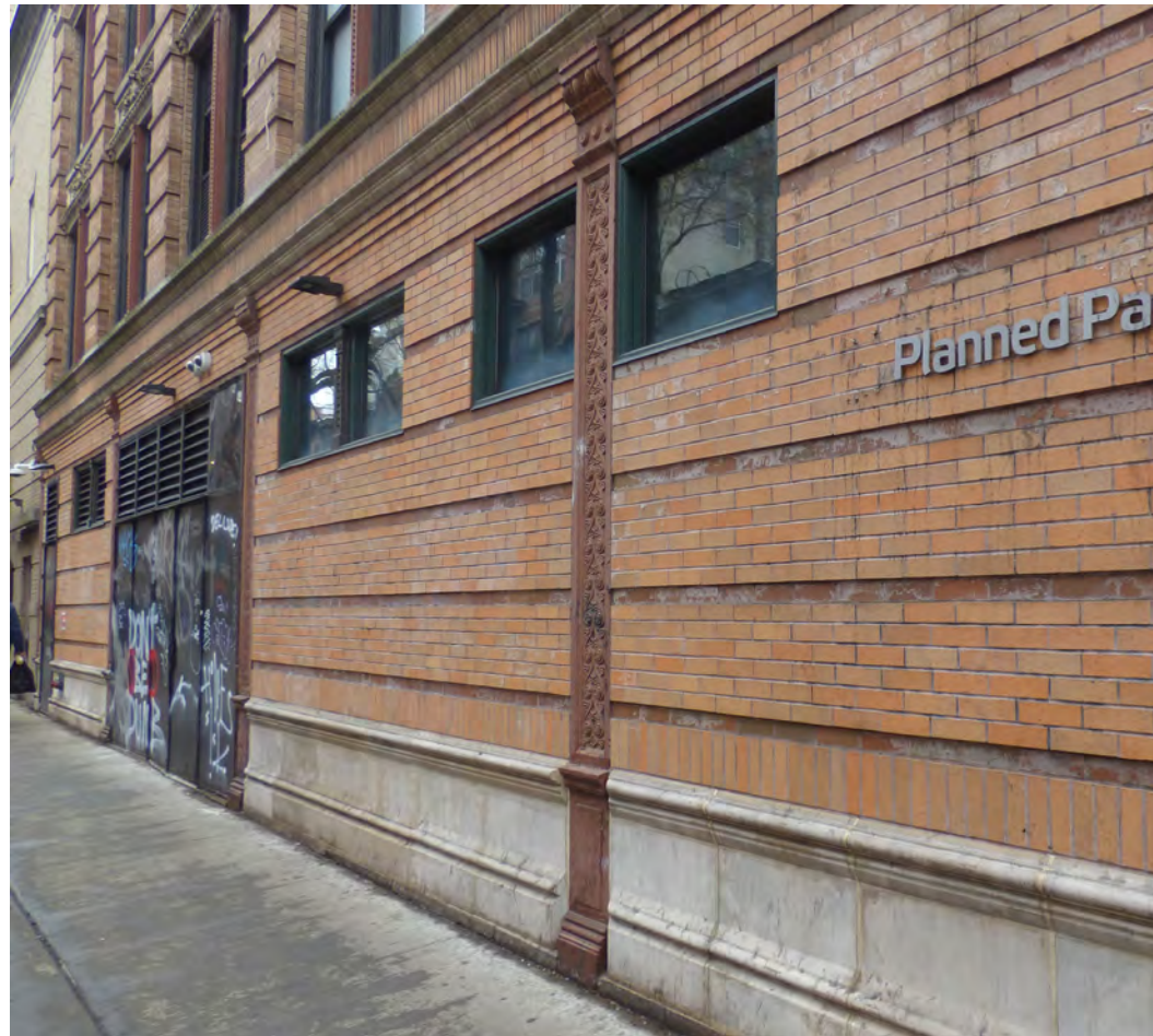
Bleecker Elevation, facing east
