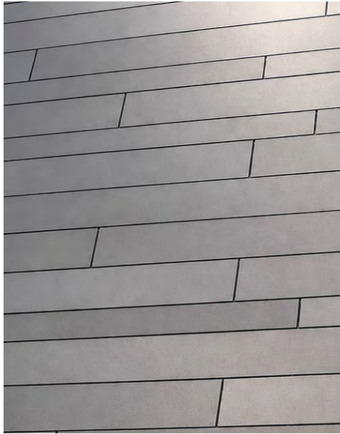
Proposed Bulkhead Cladding Zinc Flat Panel & Reveal Cladding Color Pre-Weathered Zinc Panels
