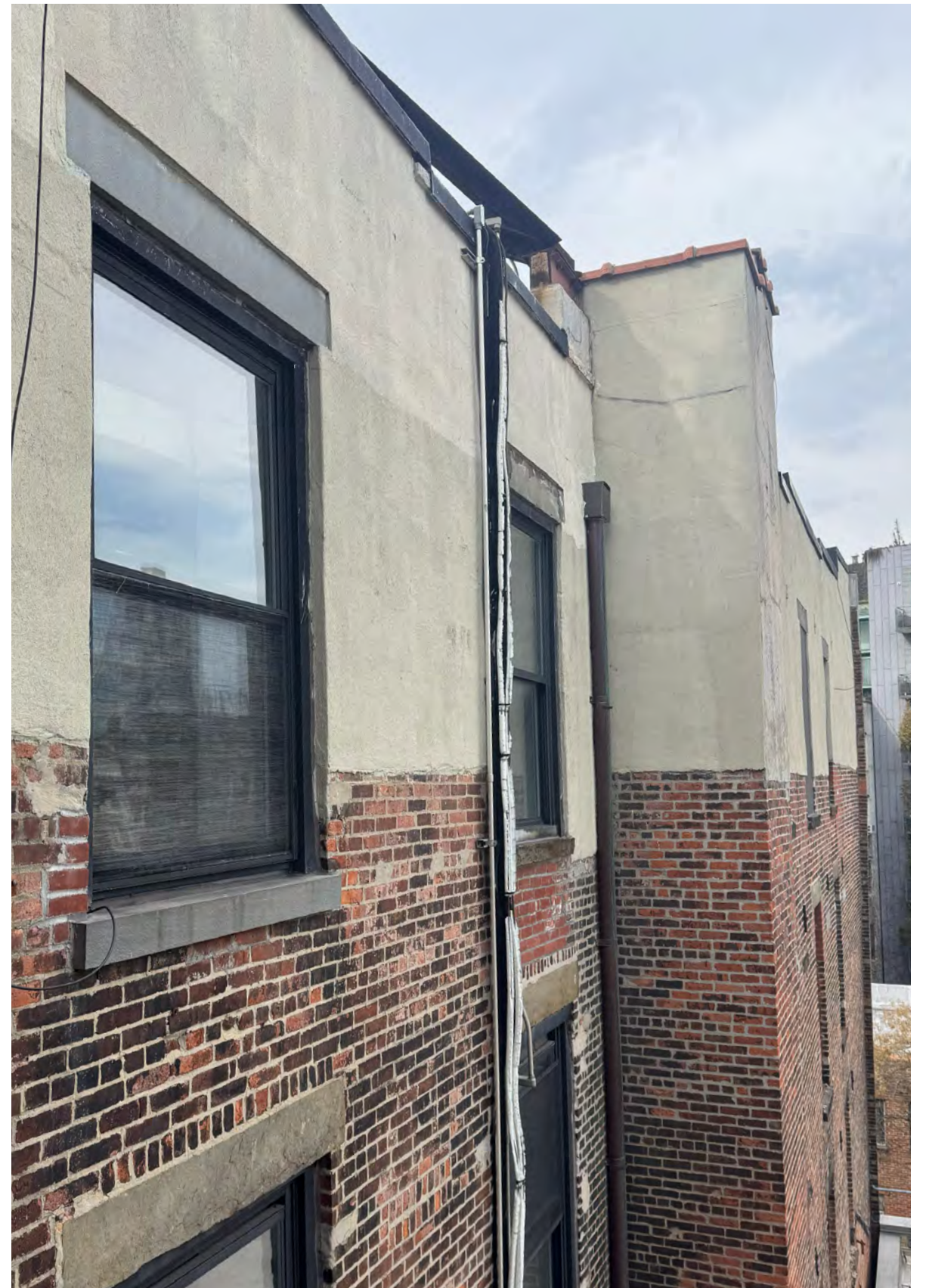
Upper Floor of East Side Elevation
