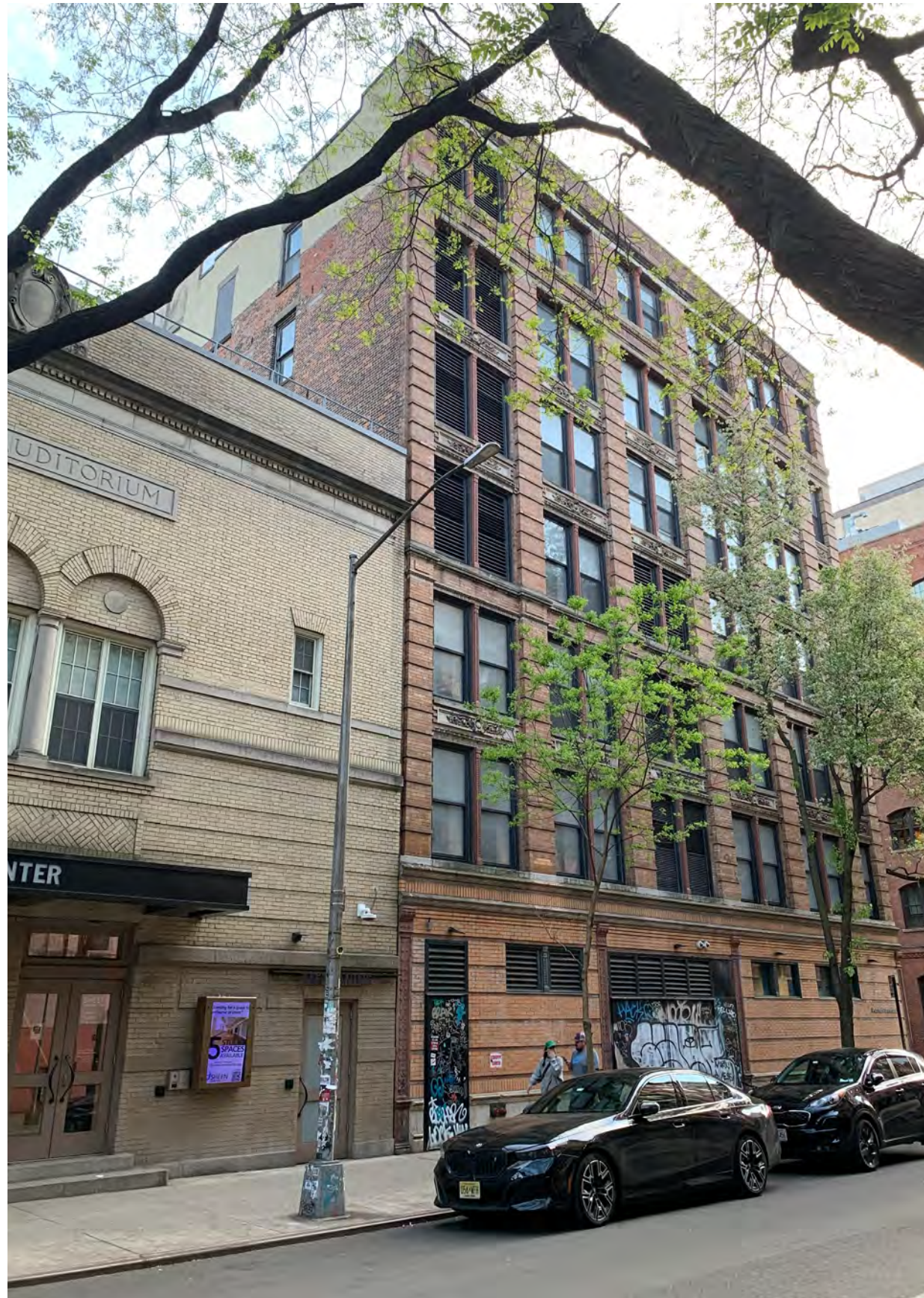
Blecker Street Facade, Facing South, 2026
