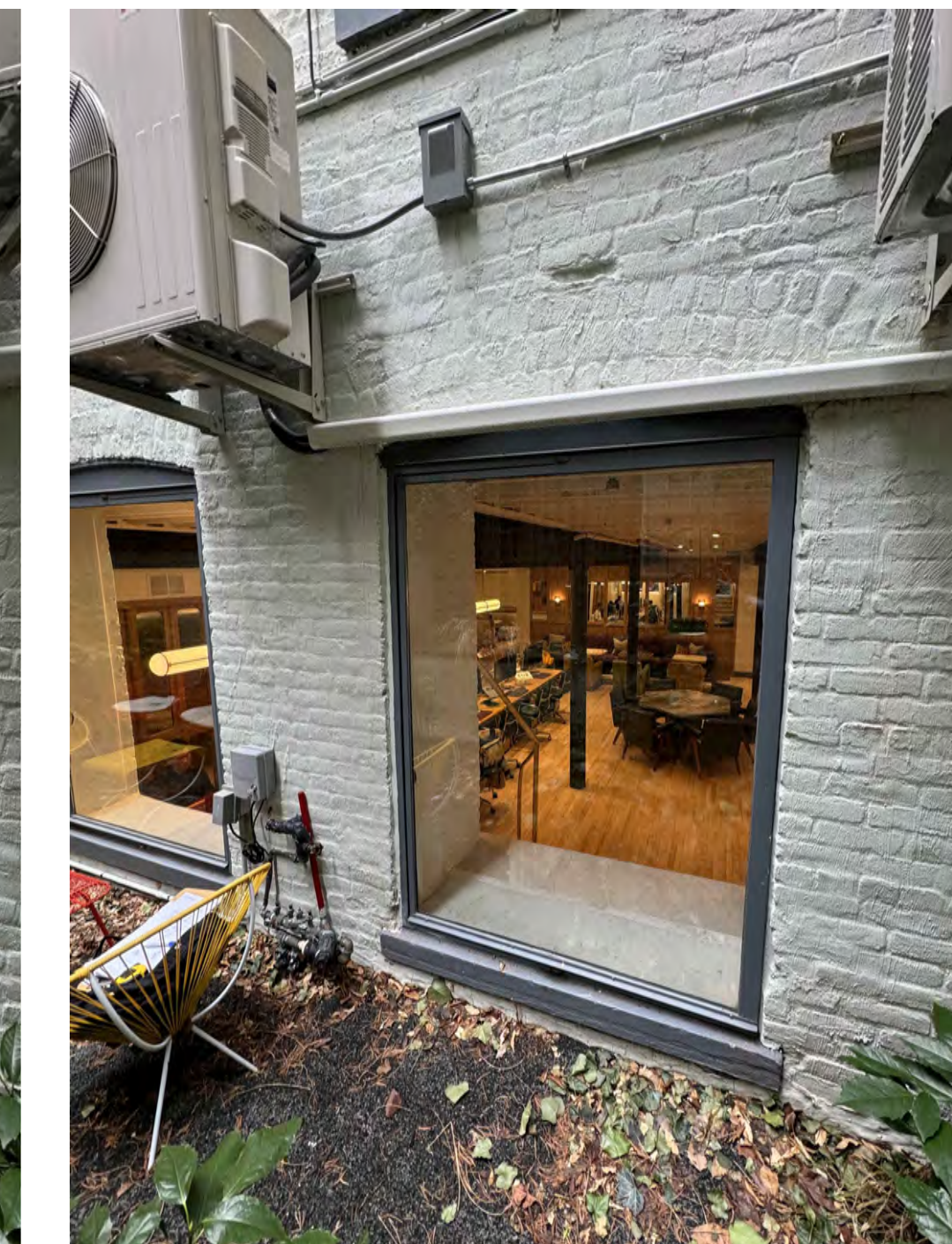
8 EX. CELLAR WINDOW-W 9 F
