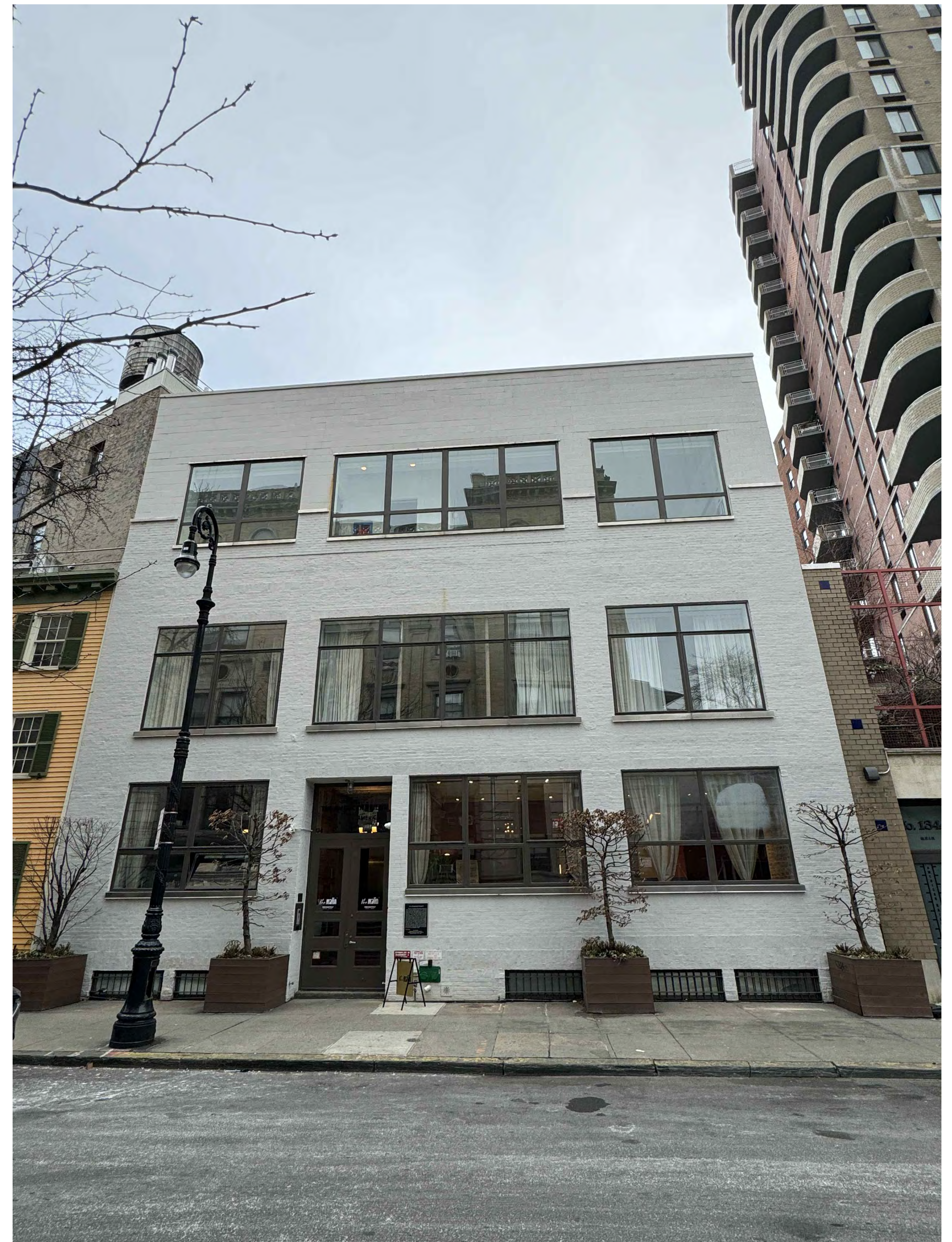
Existing Conditions - Front Facade
