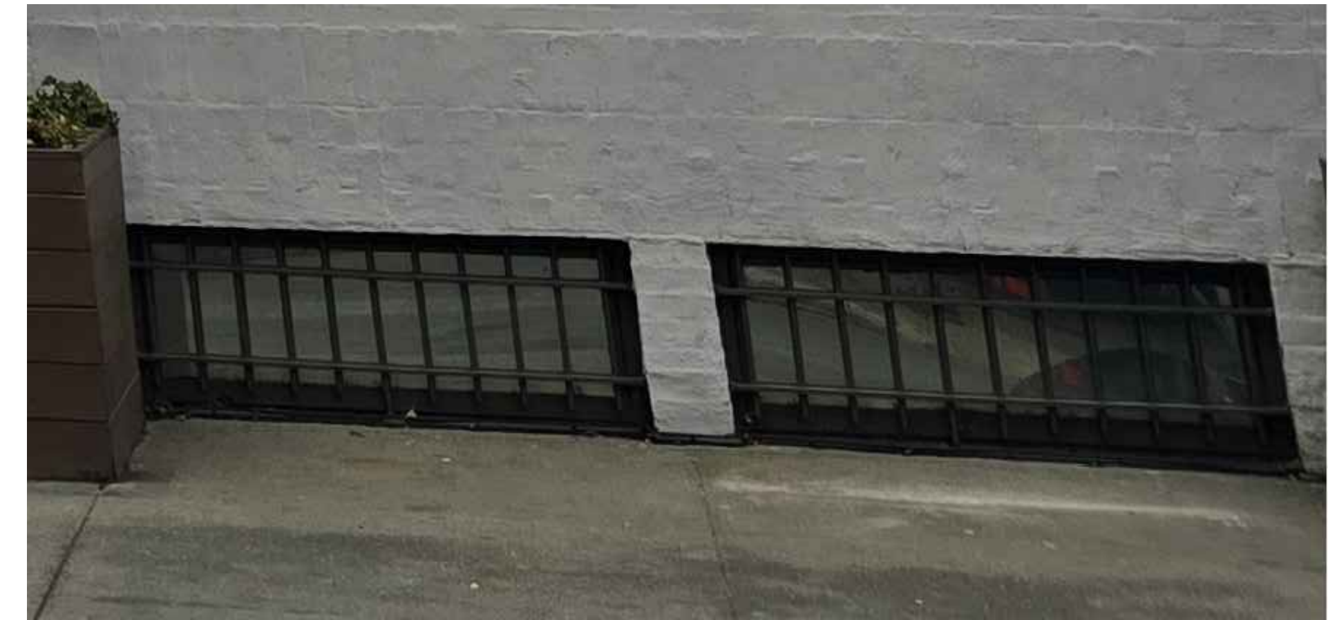
3 EXISTING CELLAR WINDOW-W 1 B (A)
