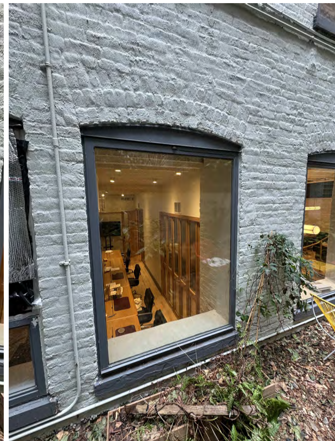
5 EX. CELLAR WINDOW-W 9 F
