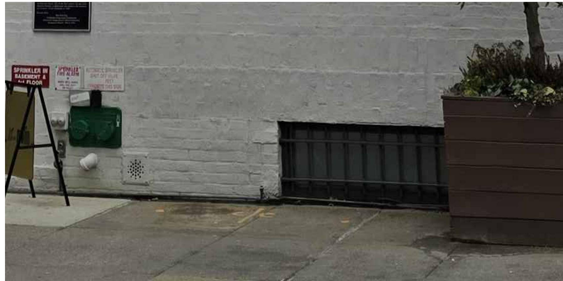
2 EXISTING CELLAR WINDOW- W 1 B (A)
