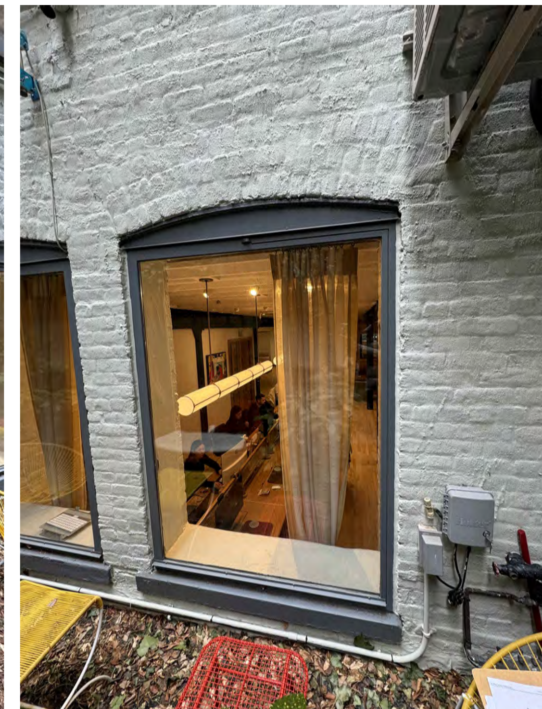
6 EX. CELLAR WINDOW-W 9 F
