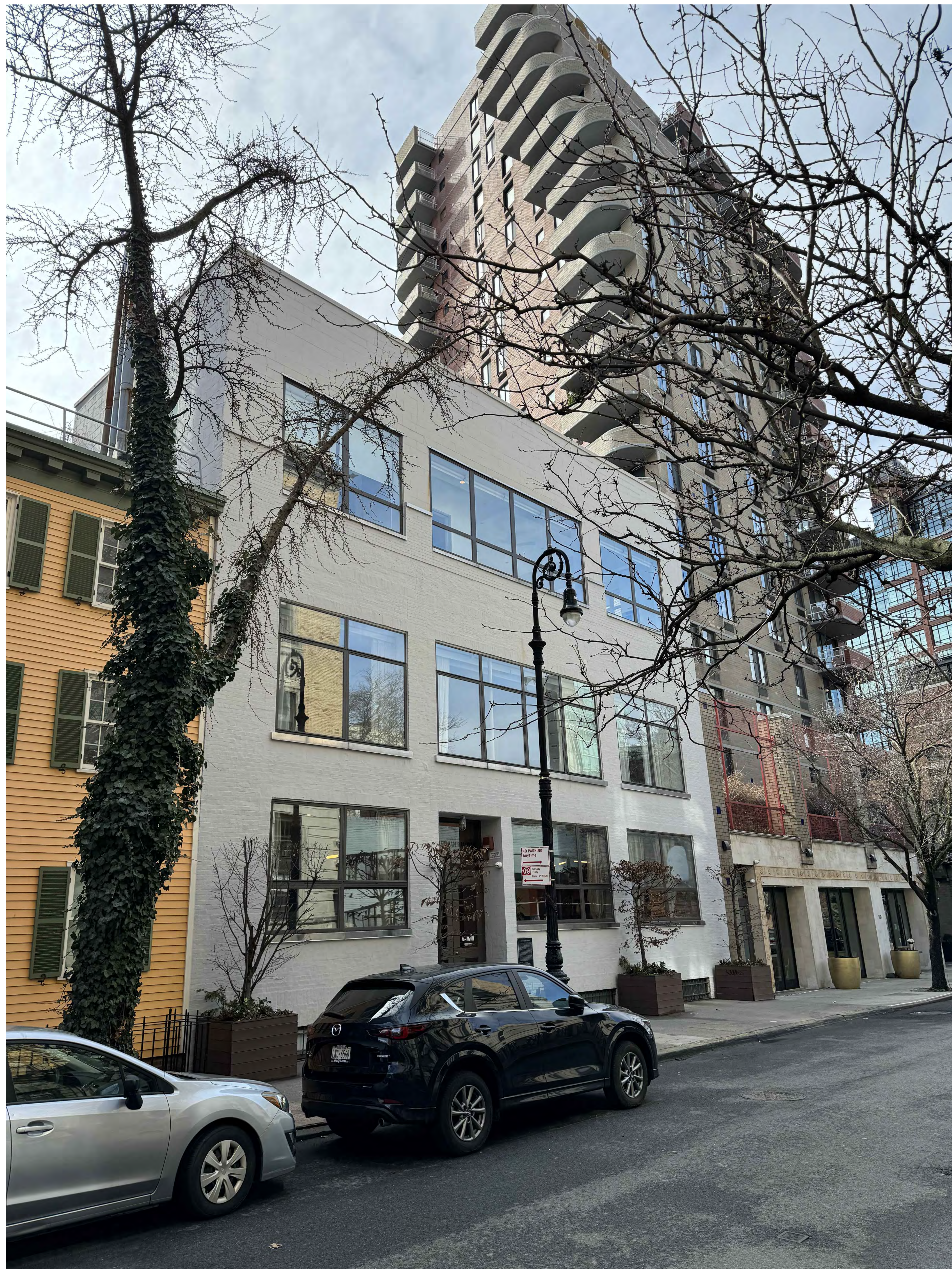
Existing Conditions - Front Facade
