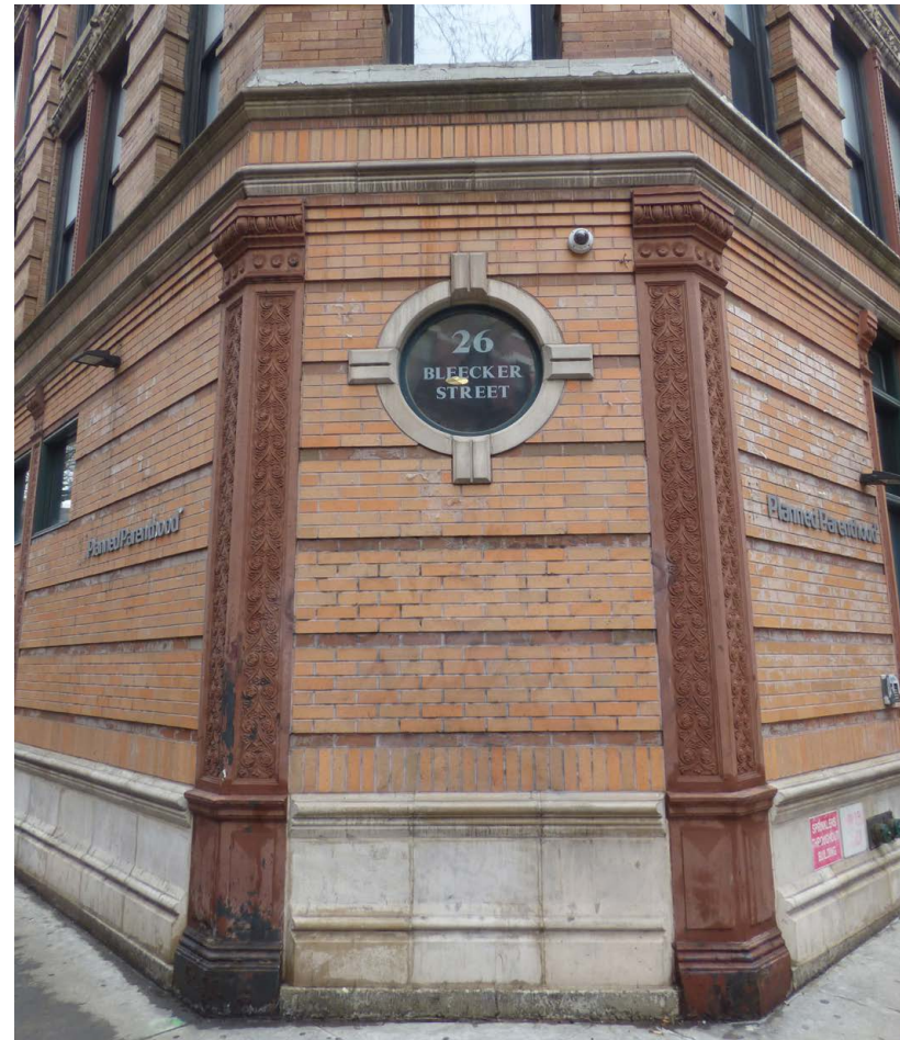
Historic Entry on northwest corner
