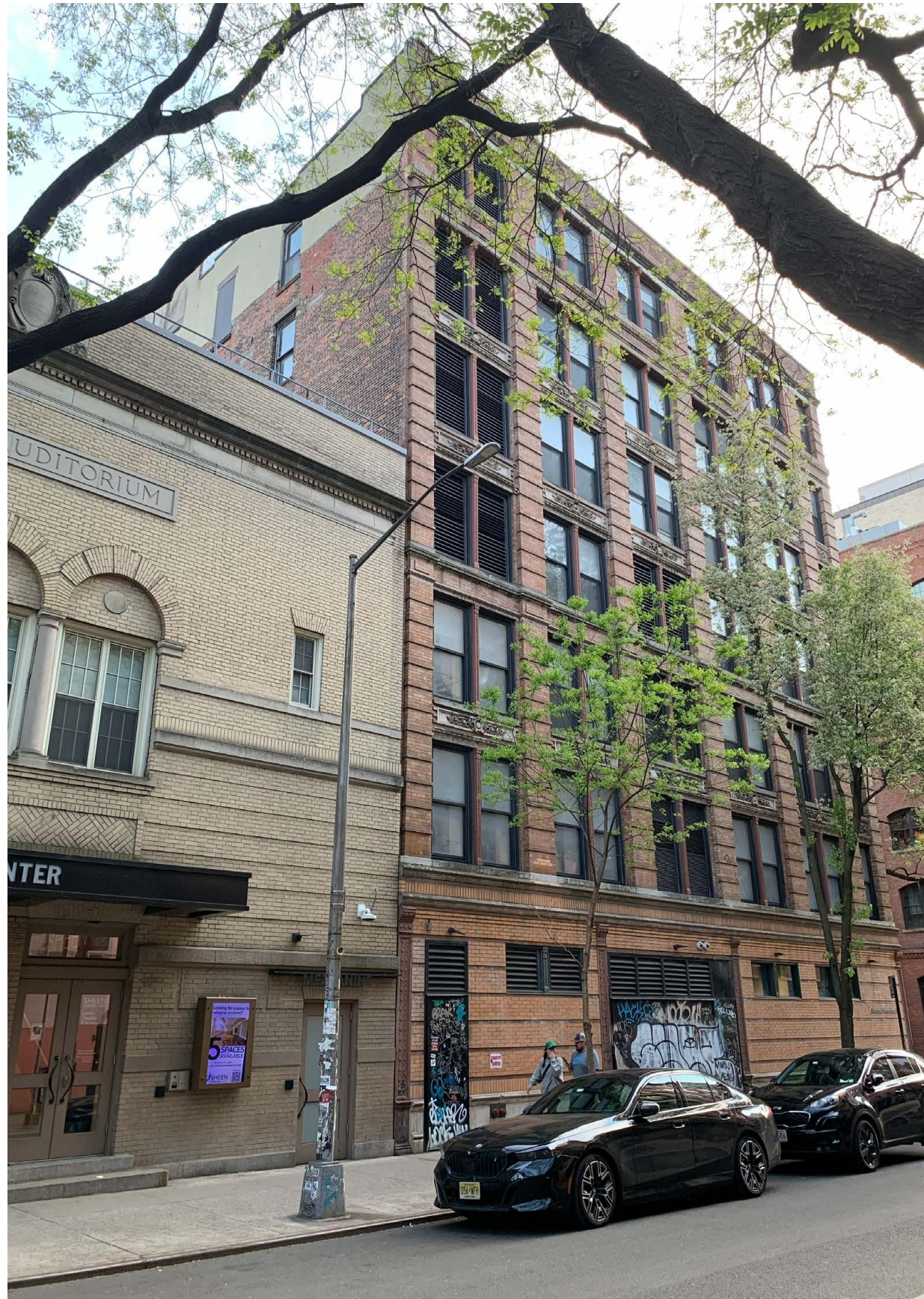
Blecker Street Facade, Facing South, 2026
