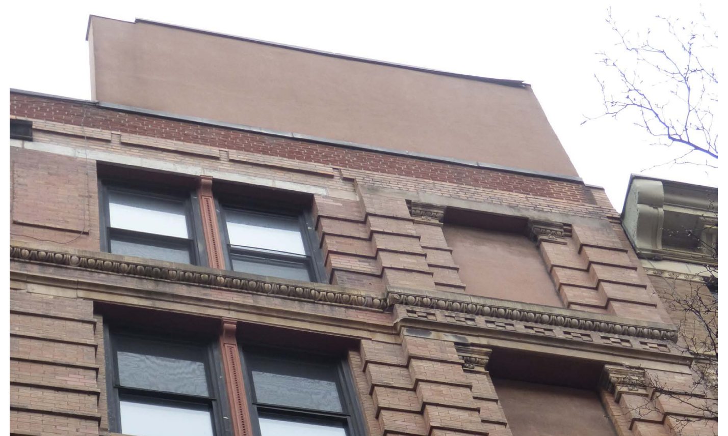
Blind Windows and Existing Elevator Bulkhead, Mott Street Elevation
