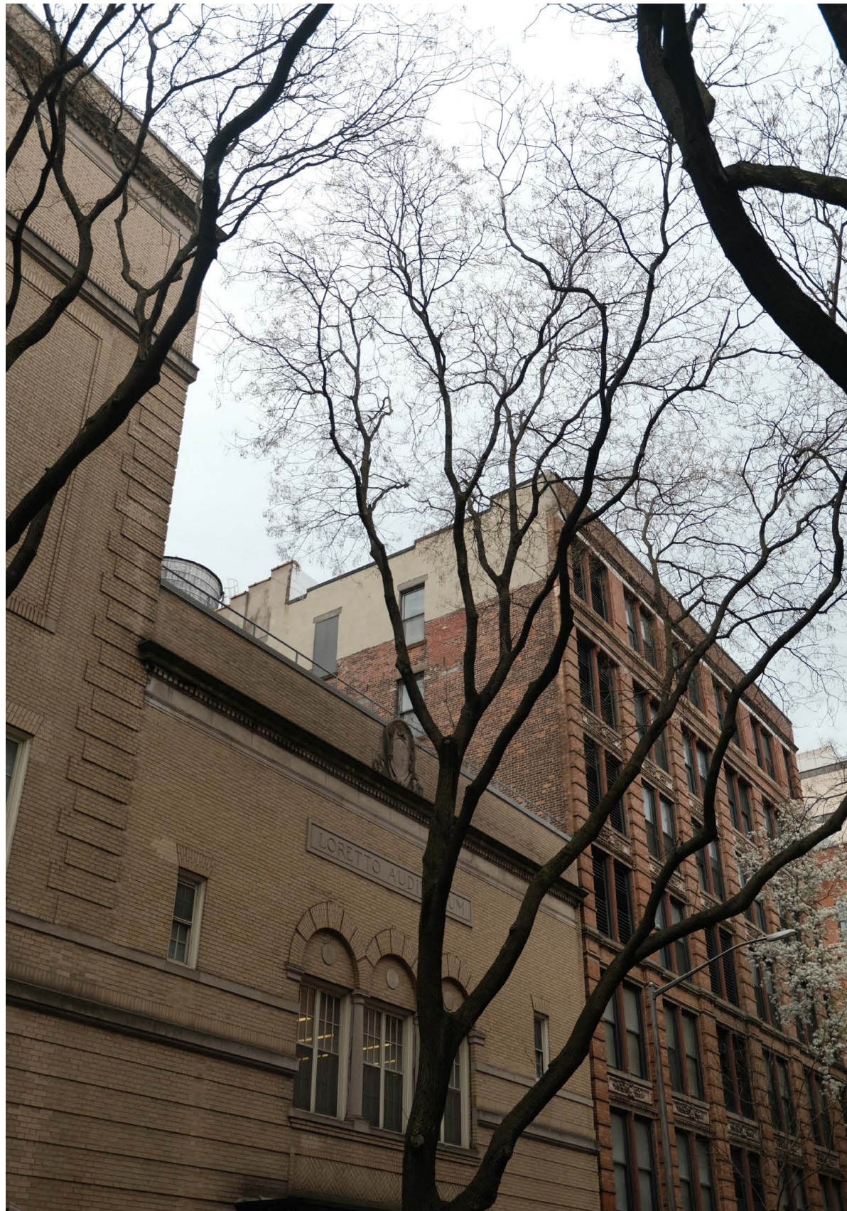
From Blecker Street, East Side Elevation
