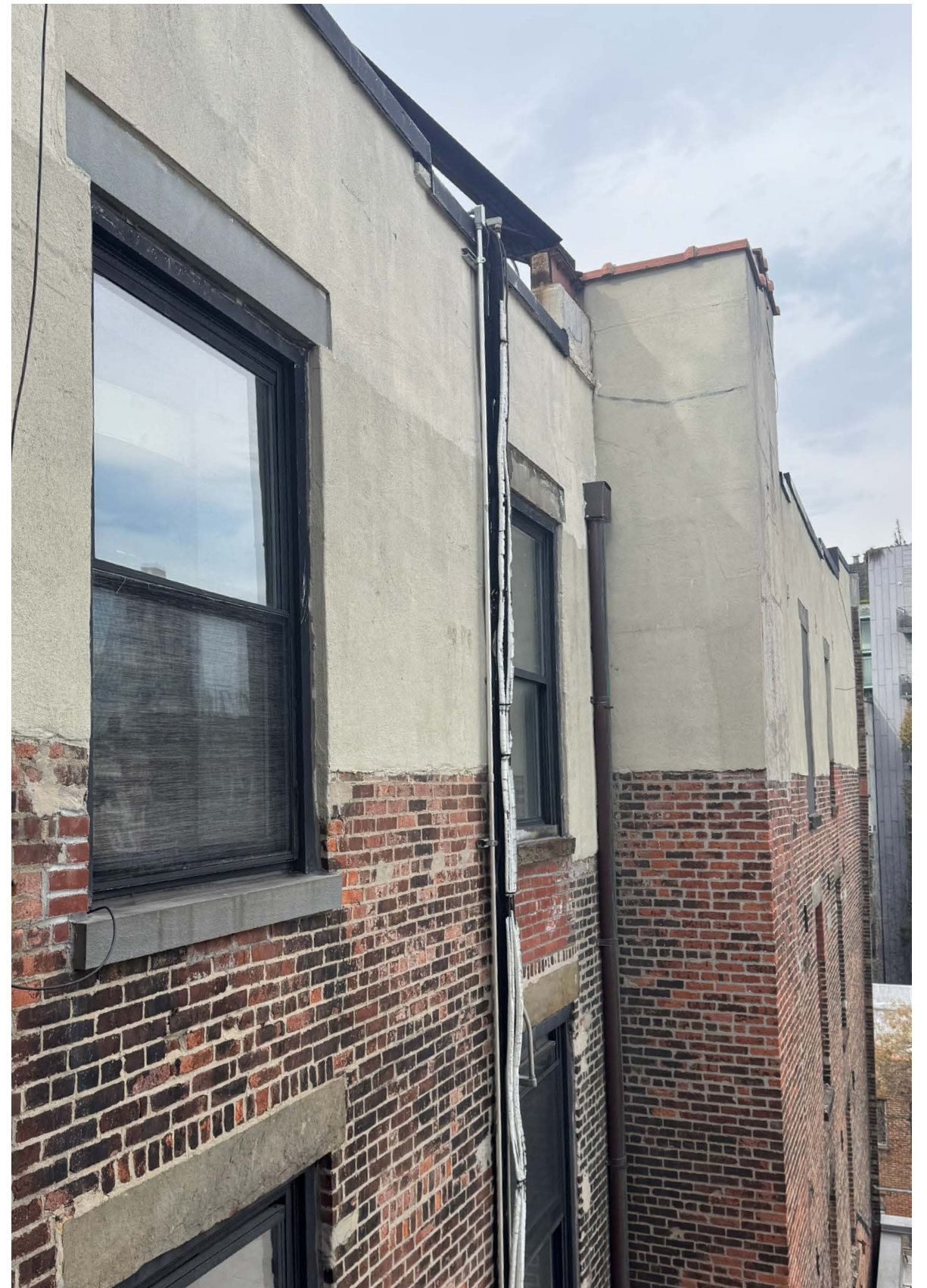
From Blecker Street, East Side Elevation
