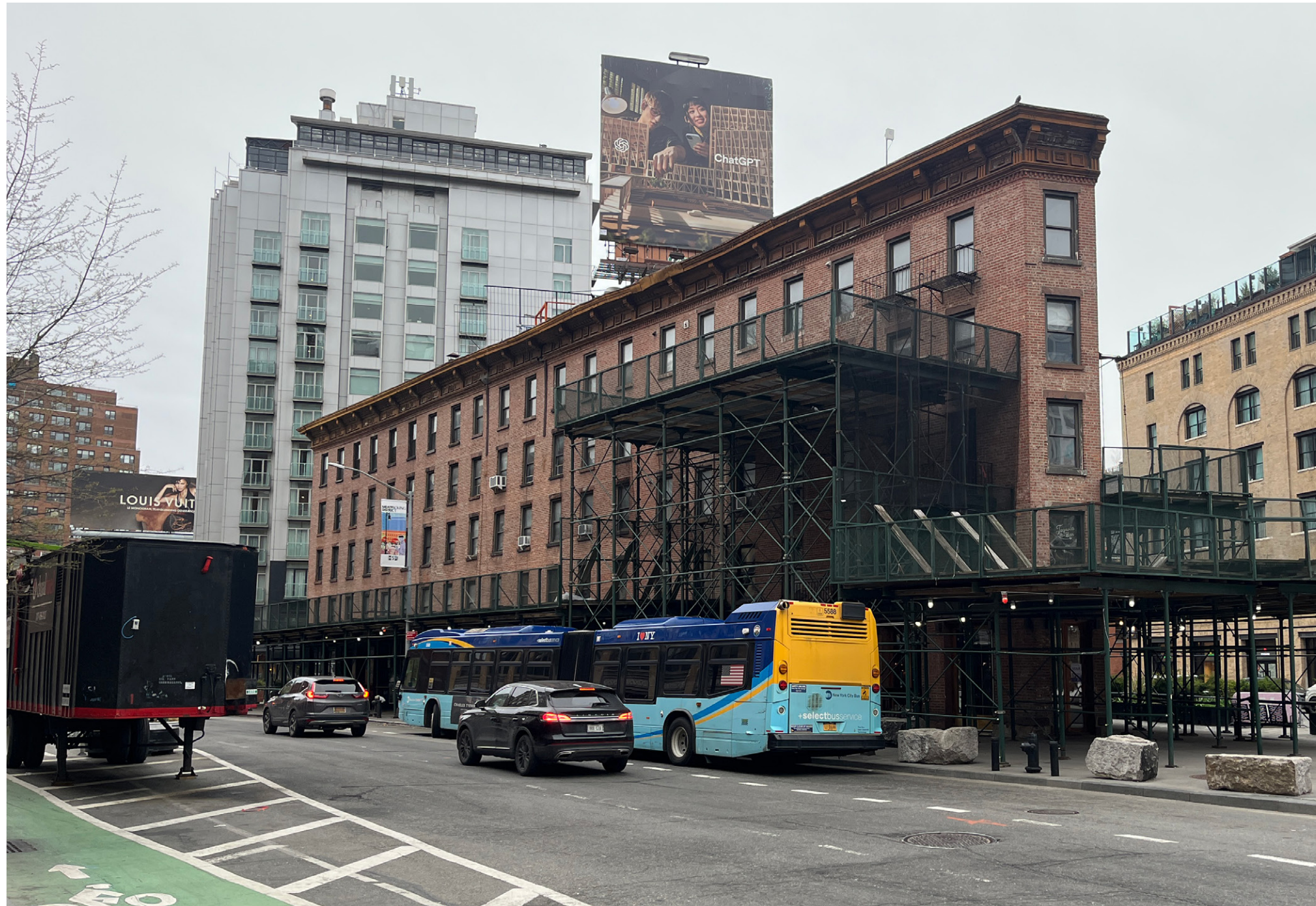
VIEW FROM THE CORNER OF HUDSON STREET AND WEST 14TH STREET
