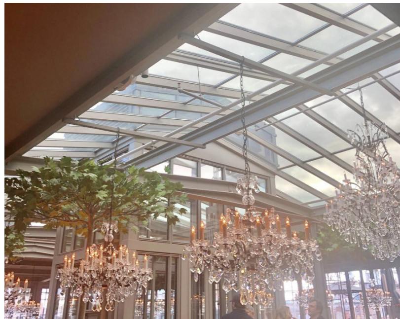
ROOFTOP OF 9-19 9TH AVENUE
