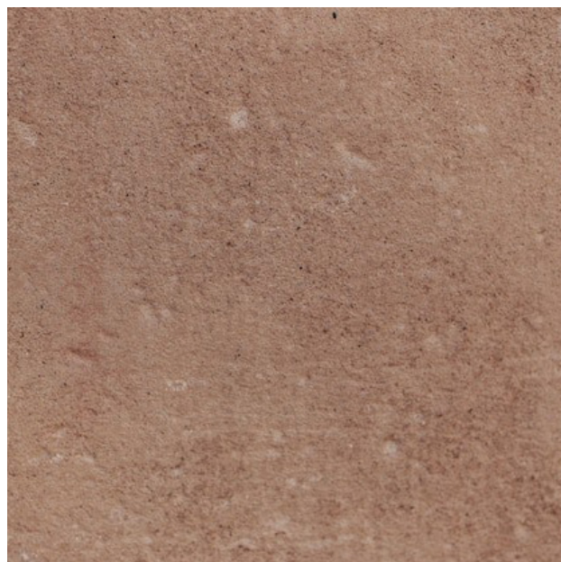
BROWNSTONE TO MATCH HISTORIC AT: - WINDOW SILLS
