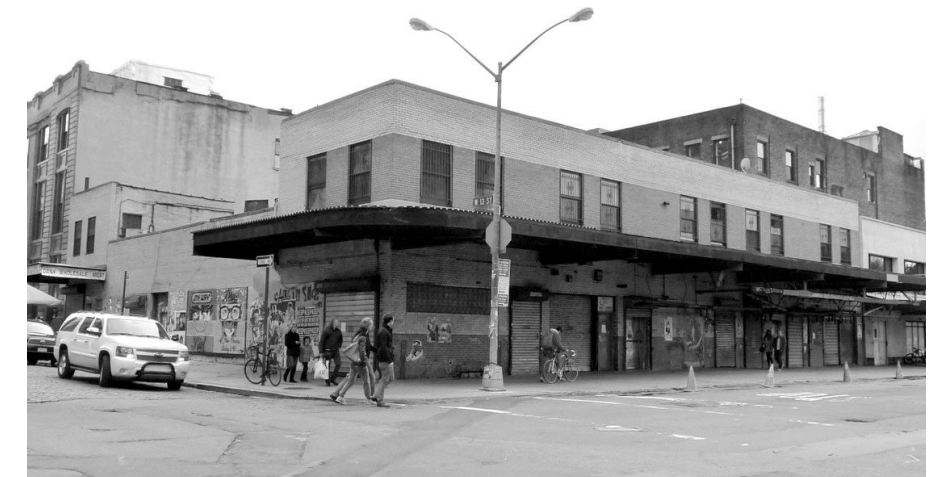
LPC DESIGNATION PHOTO 2003
