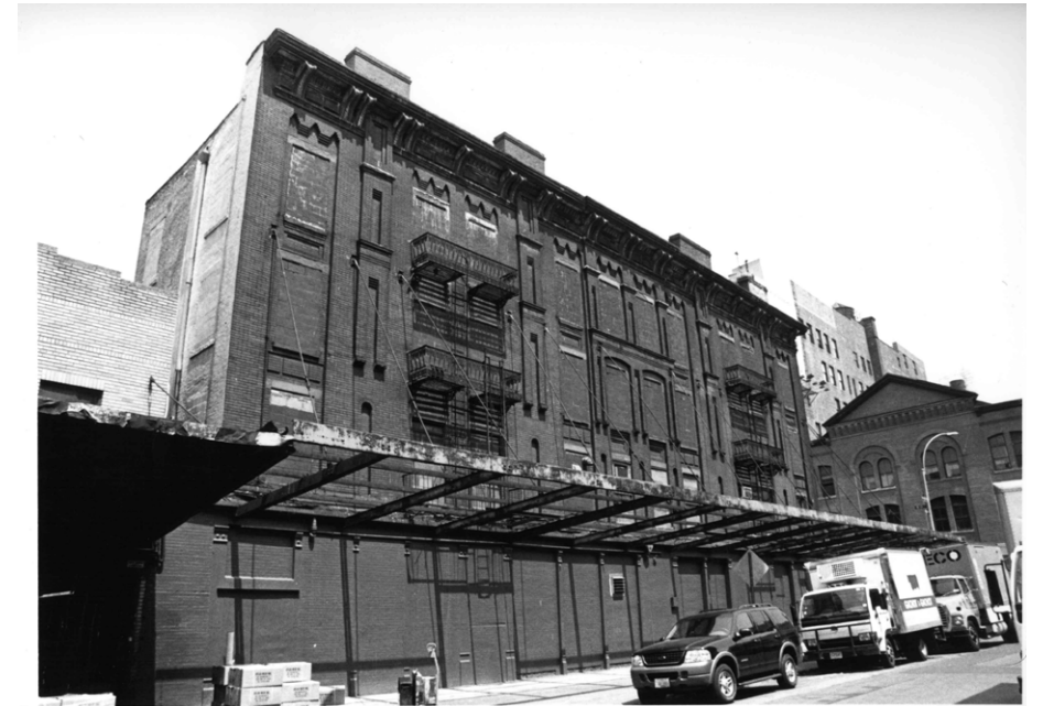
LPC DESIGNATION PHOTO 2003
