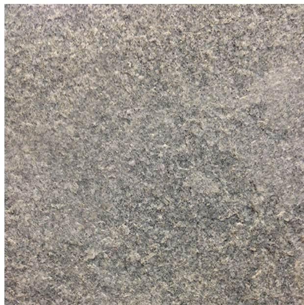
GRANITE TO MATCH HISTORIC AT: - GROUND FLOOR RESTORED BELT COURSE
