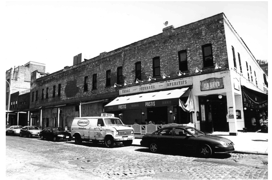
LPC DESIGNATION PHOTO 2003
