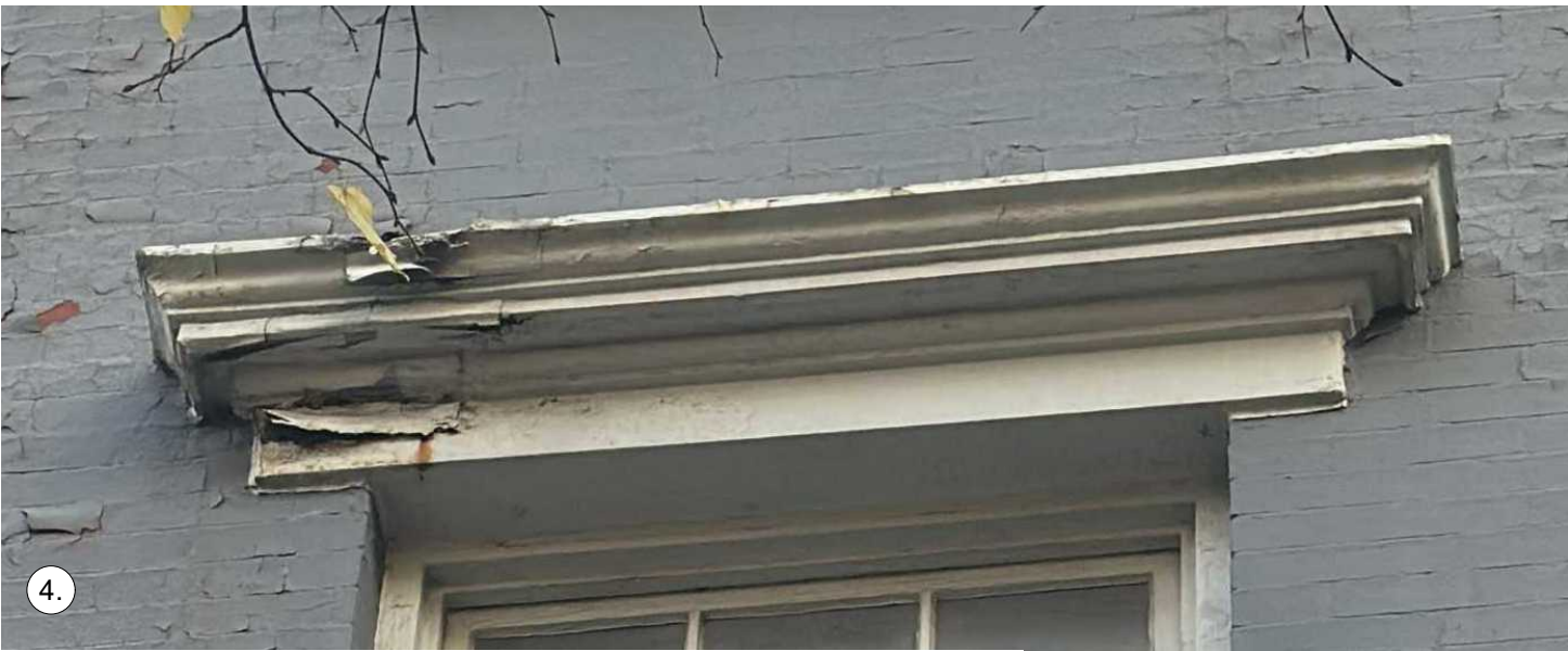
DETAIL PHOTO OF METAL CAPPING AT 1ST FLOOR WINDOW
