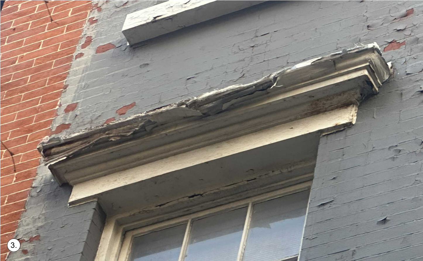
DETAIL PHOTO OF METAL CAPPING AT 1ST FLOOR WINDOW
