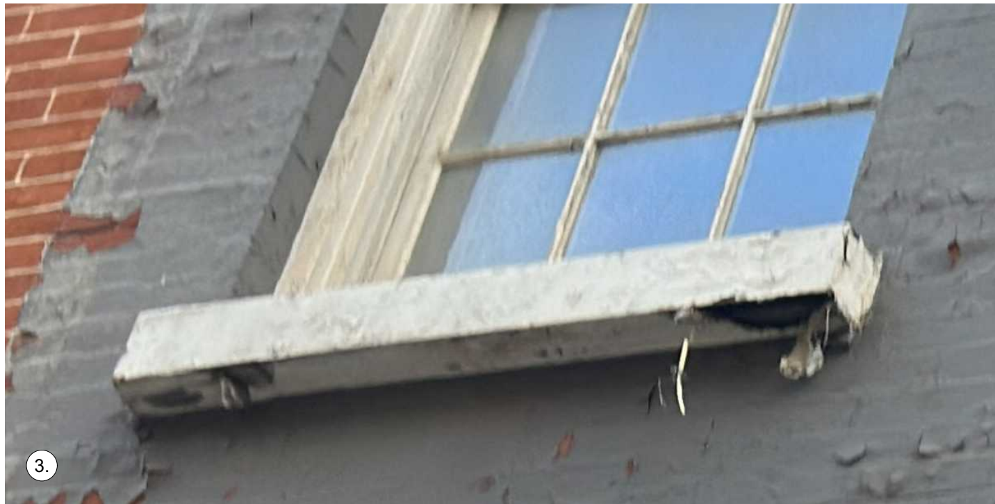
SAMPLE DETAIL PHOTO OF METAL CAPPED SILL AT THE 1ST FLOOR WINDOW
