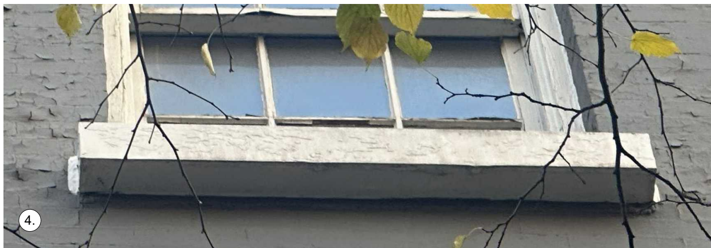
SAMPLE DETAIL PHOTO OF METAL CAPPED SILL AT THE 1ST FLOOR WINDOW
