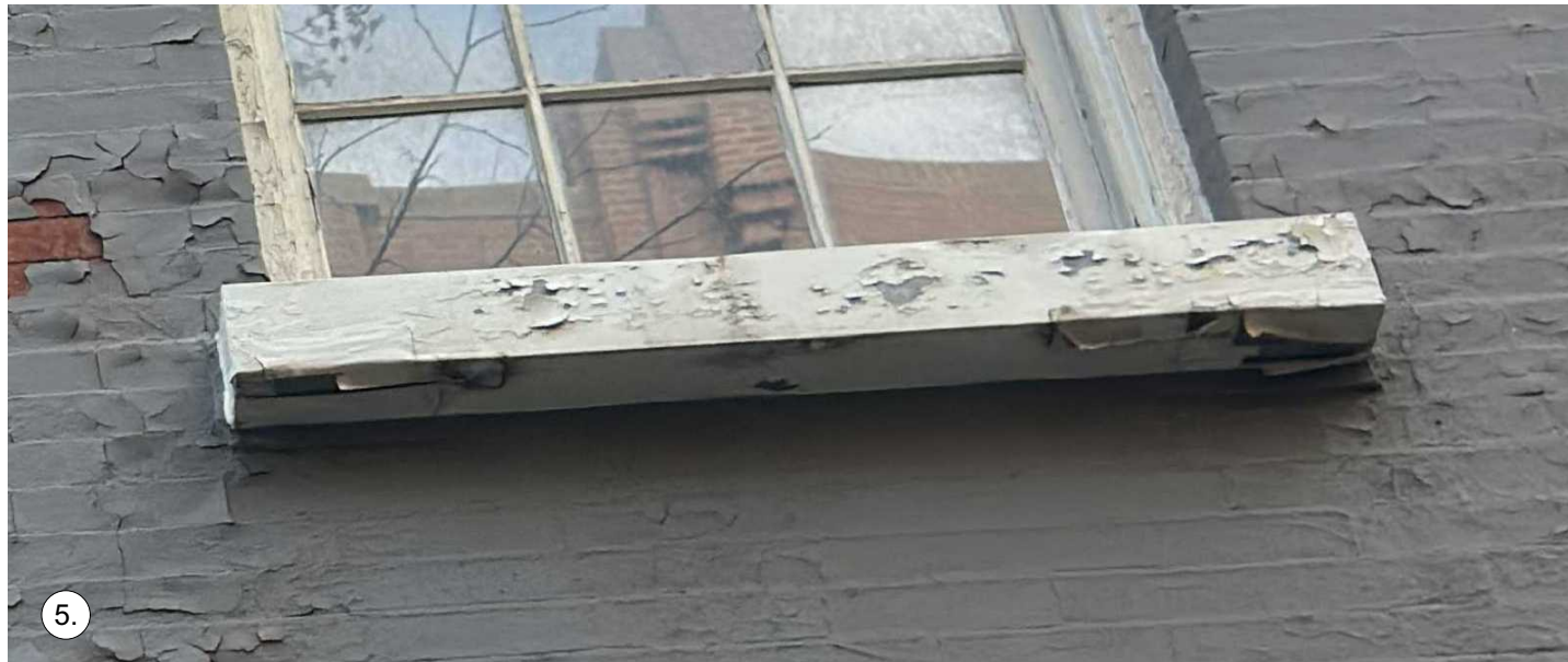
SAMPLE DETAIL PHOTO OF METAL CAPPED SILL AT THE 1ST FLOOR WINDOW
