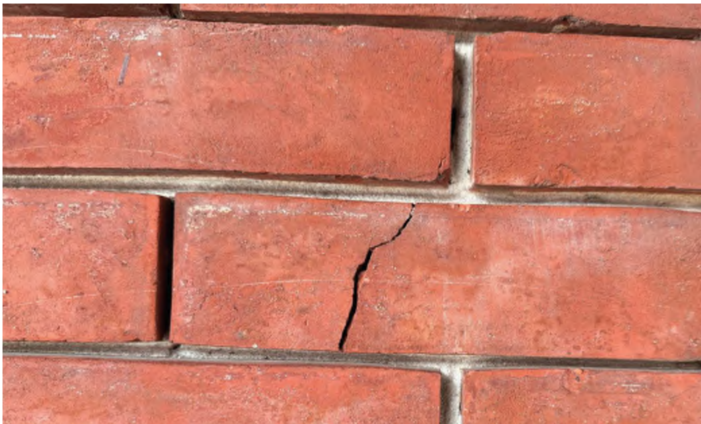
3 Brick Crack
