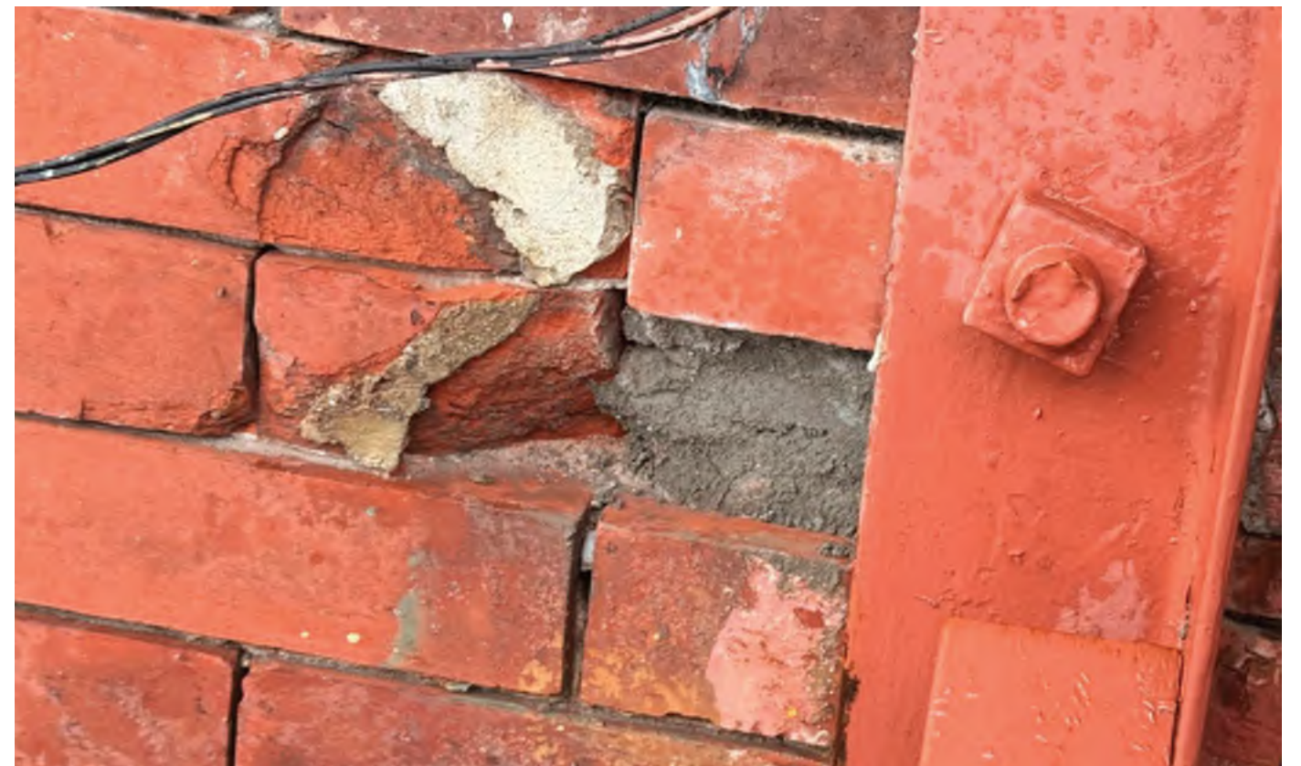
4 Missing/Damaged Brick
