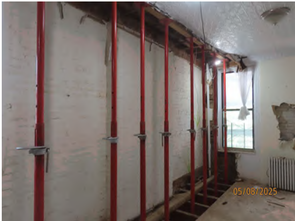
SHORING JACKS SPANNING TWO FLOORS
