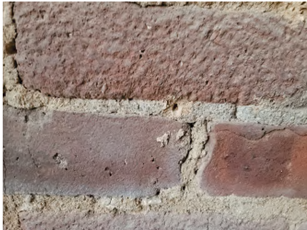
DETAIL OF MASONRY FOLLOWING PIN TEST
