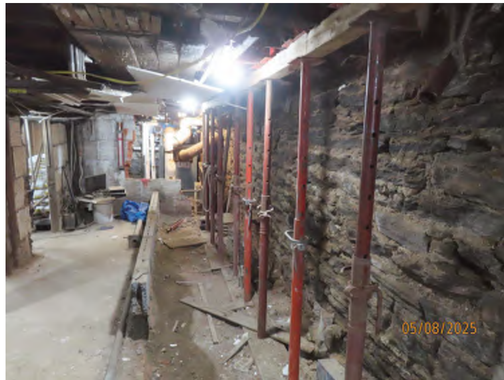
CURRENT CONDITION AT CELLAR
