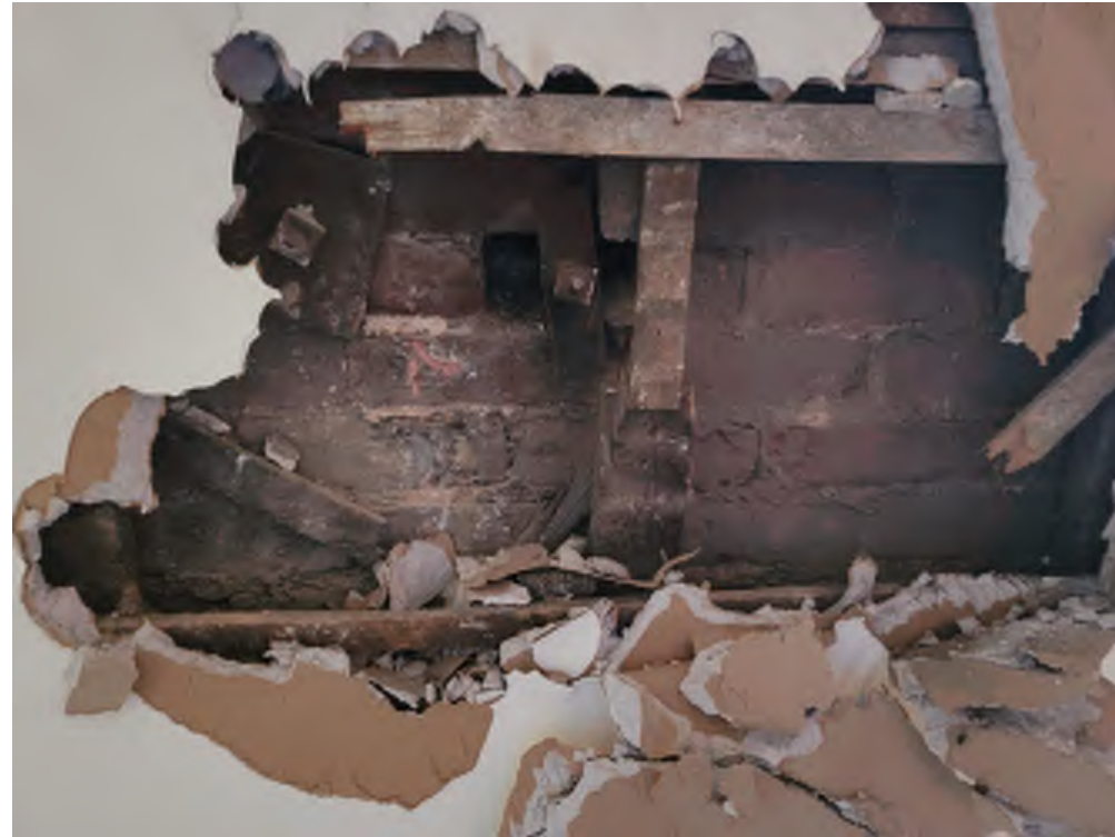
PROBE AT INTERIOR OF FACADE
