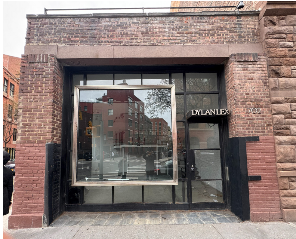
CURRENT BUILDING PHOTO - 2025
