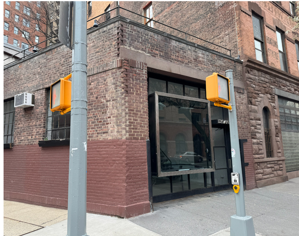
CURRENT BUILDING PHOTO - 2025
