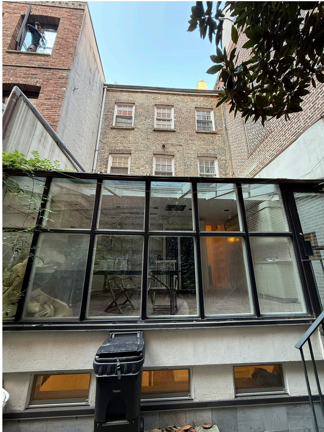
Existing rear extension
