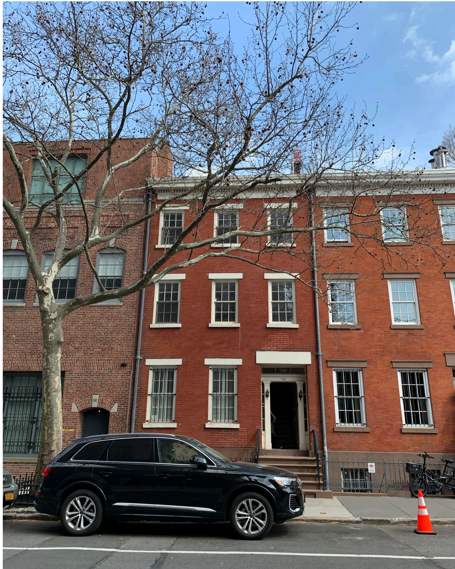
View east toward primary facade from across Washington Street, chimney extension is visible
