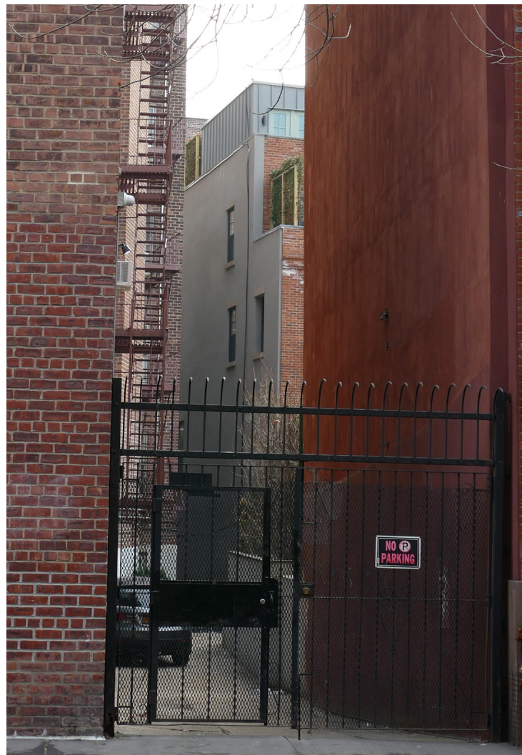
105-107 Bank Street, Rear Elevation
