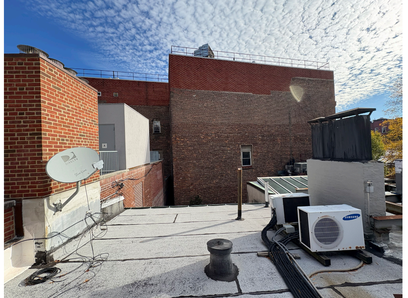
View of the roof - looking east
