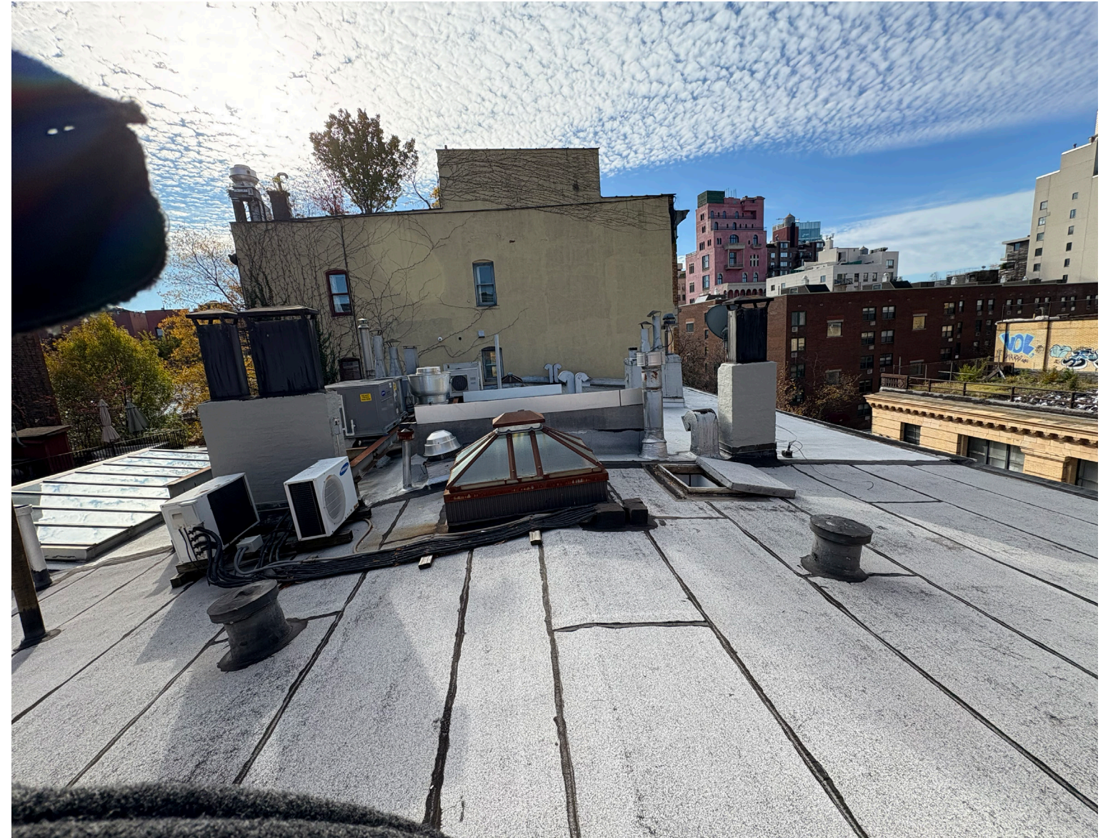
View of the roof - looking south
