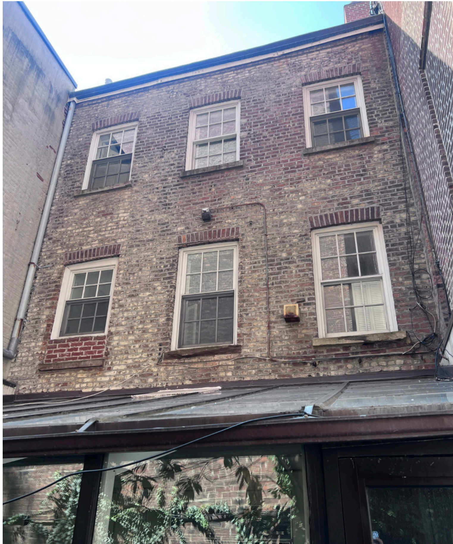
Existing Conditions - Rear Facade Details
