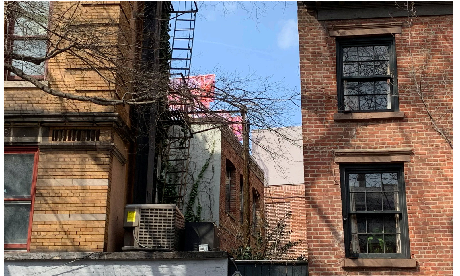
Stair bulkhead and mechanical enclosure detail
