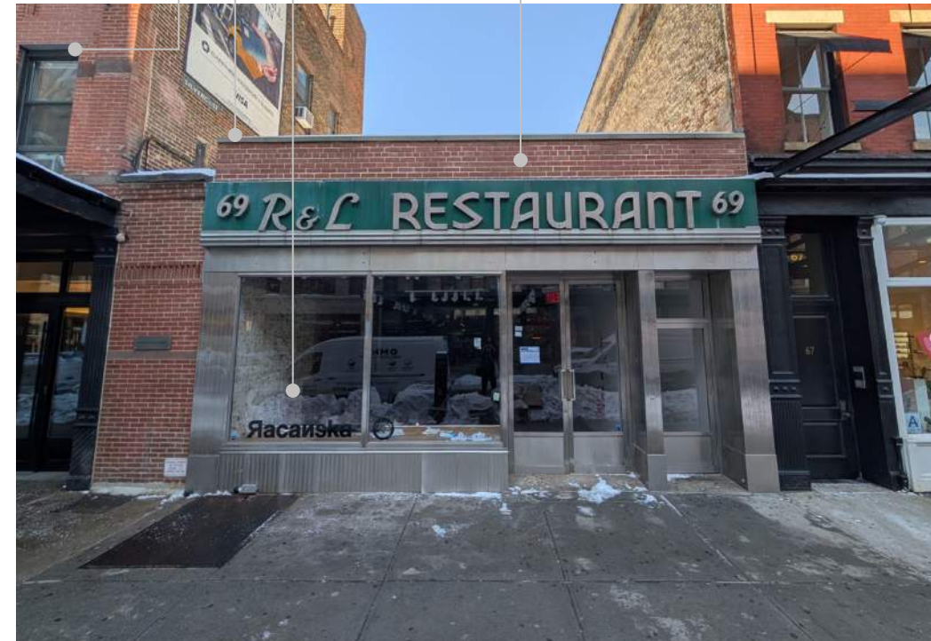
EXISTING STREET FACADE
