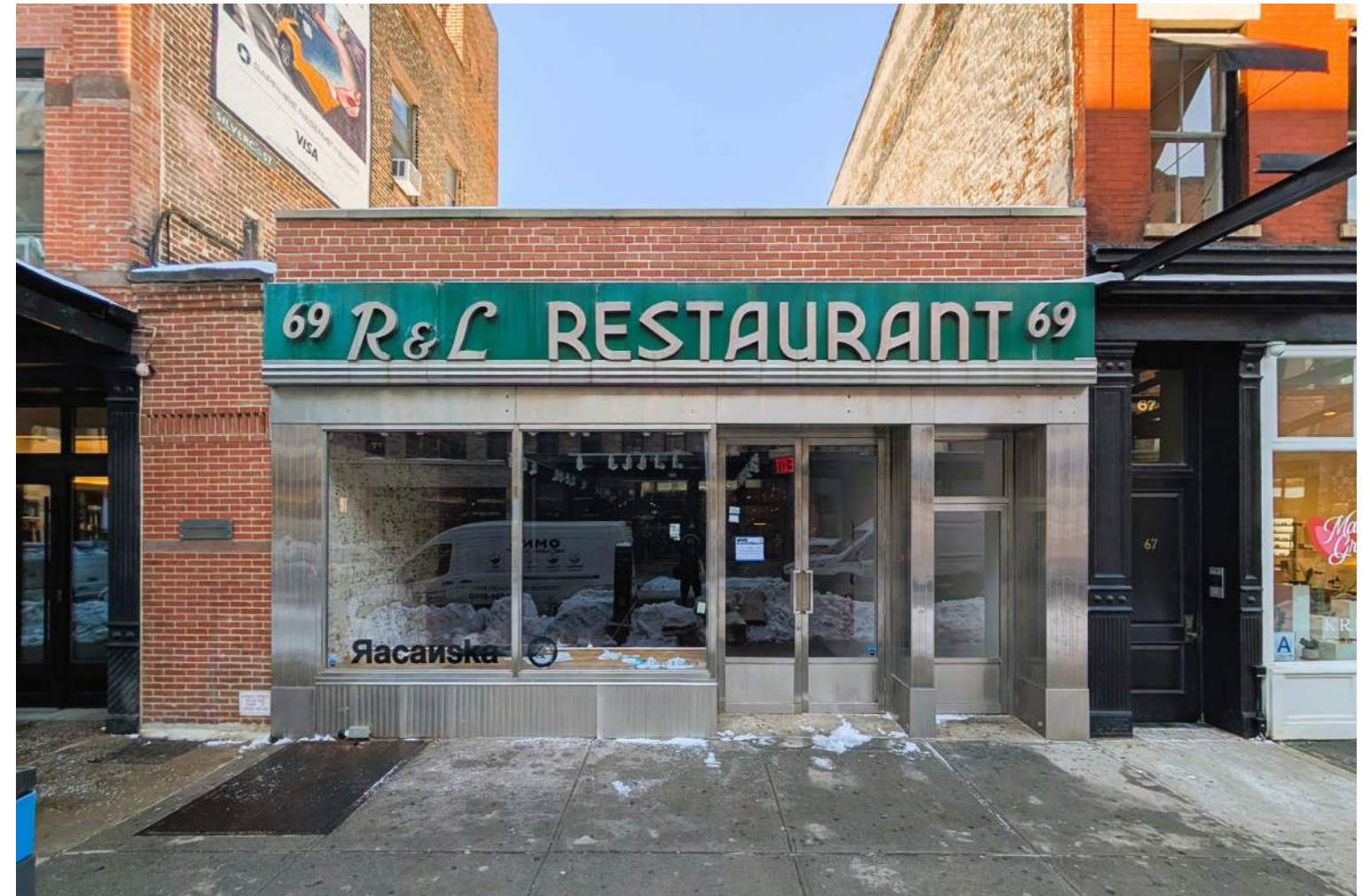
EXISTING SOUTH FACADE
