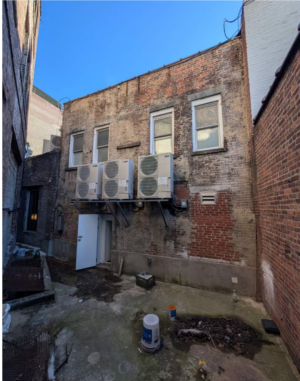
1 | NORTH ELEVATION - REAR FACADE
