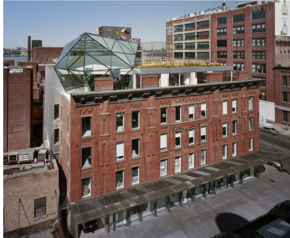
440 WEST 14TH STREET DOB ALT1 104028062 | APPLICATION APPROVED 04/01/2005 CONTRASTING MODERN INTERVENTION
