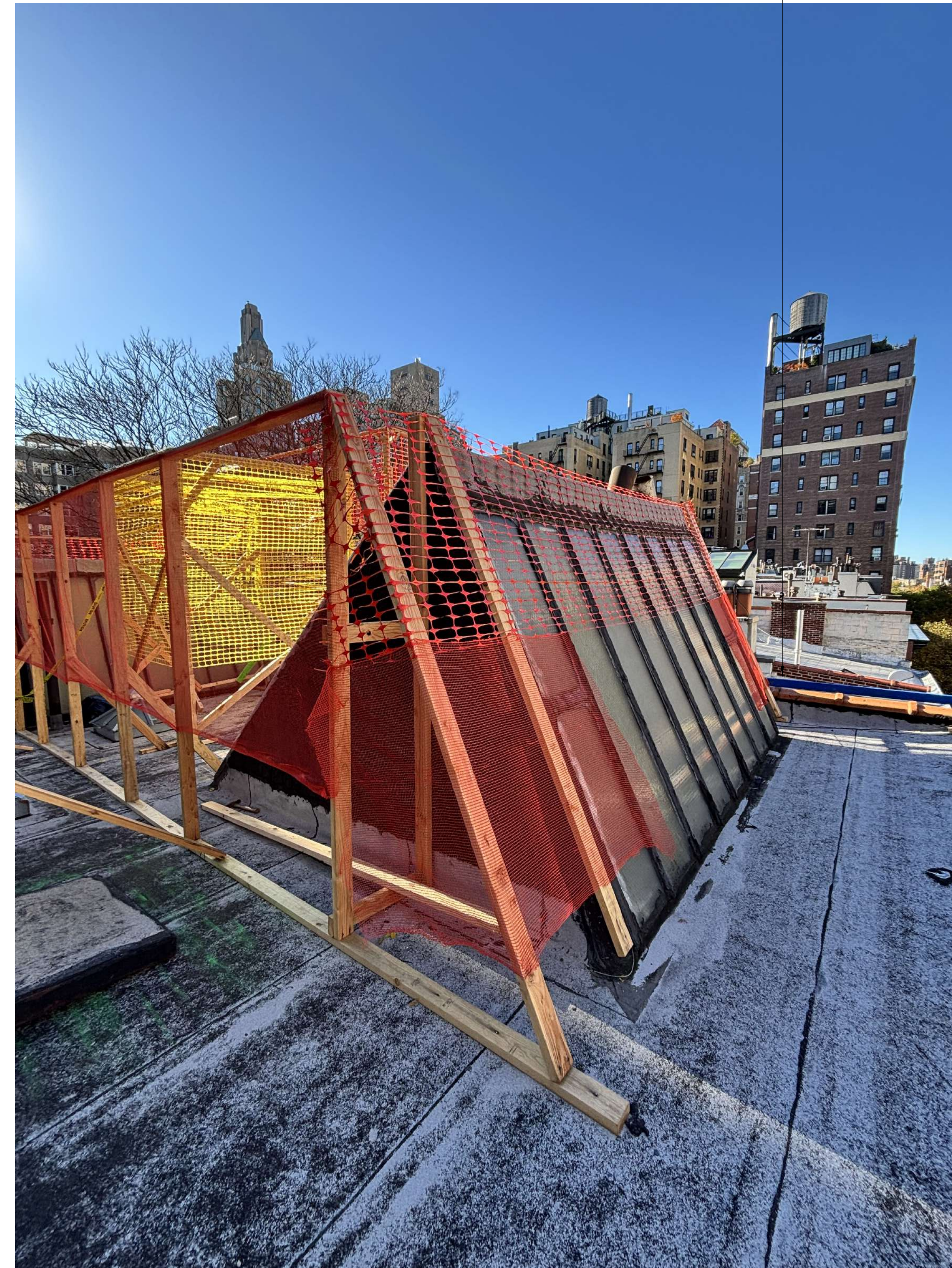
B - MOCKUP LOOKING SOUTHWEST TOWARDS SKYLIGHT
