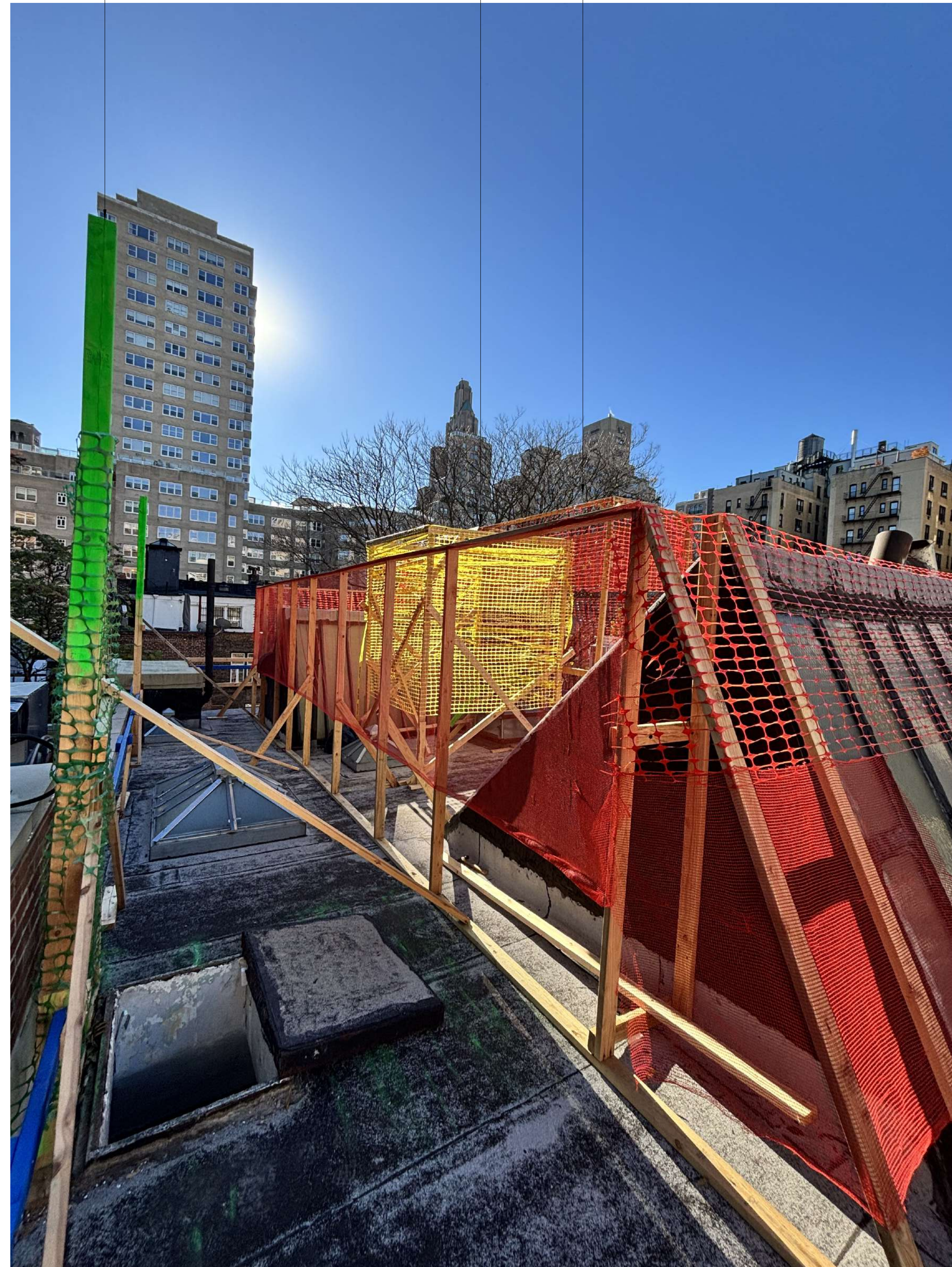
A - MOCKUP LOOKING SOUTH TOWARDS REAR YARD
