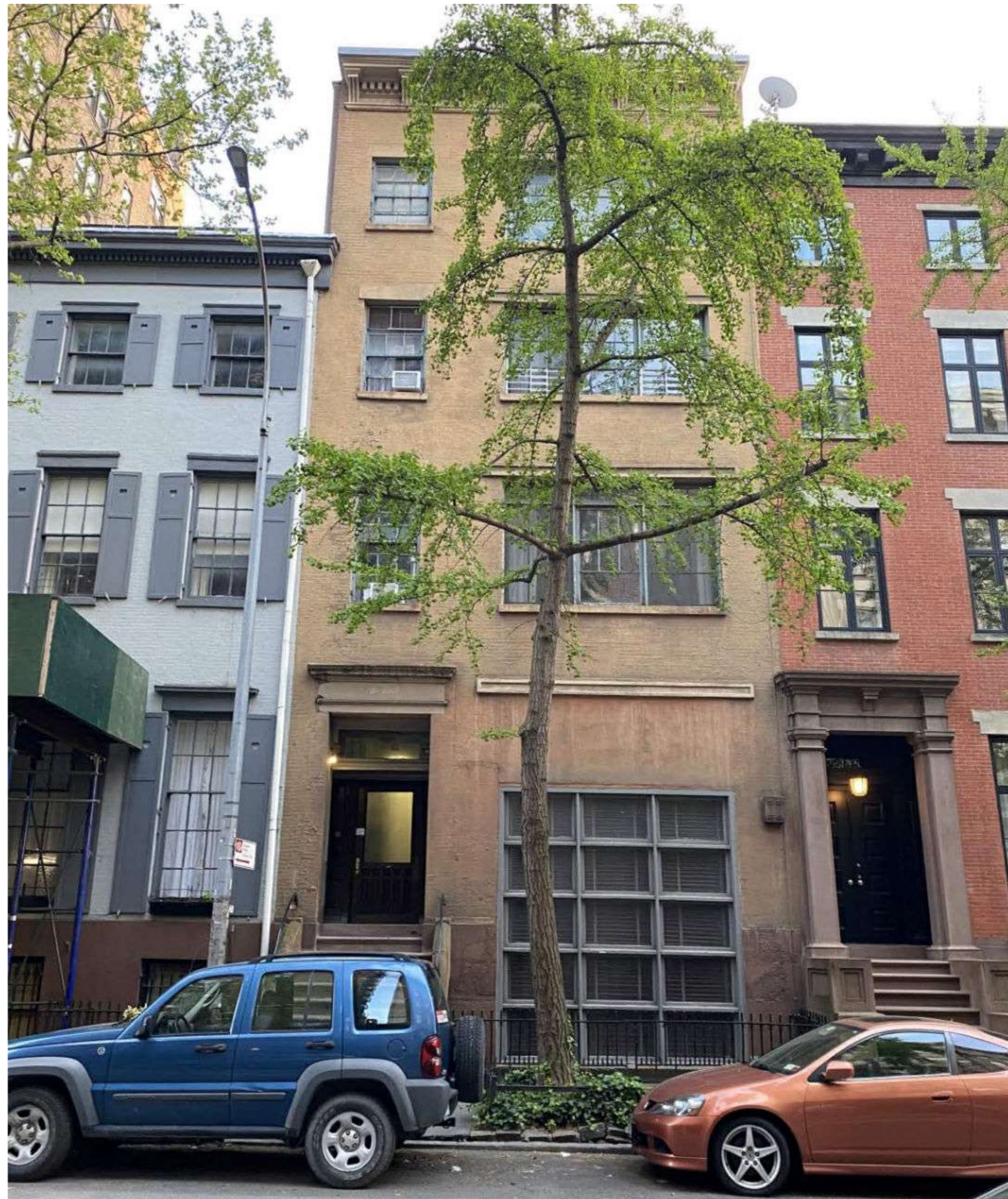
EXISTING FRONT FACADE PHOTO 2025 ORIGINALLY BUILT IN 1844 AS PAIR WITH #24 IN GREEK REVIVAL STYLE
