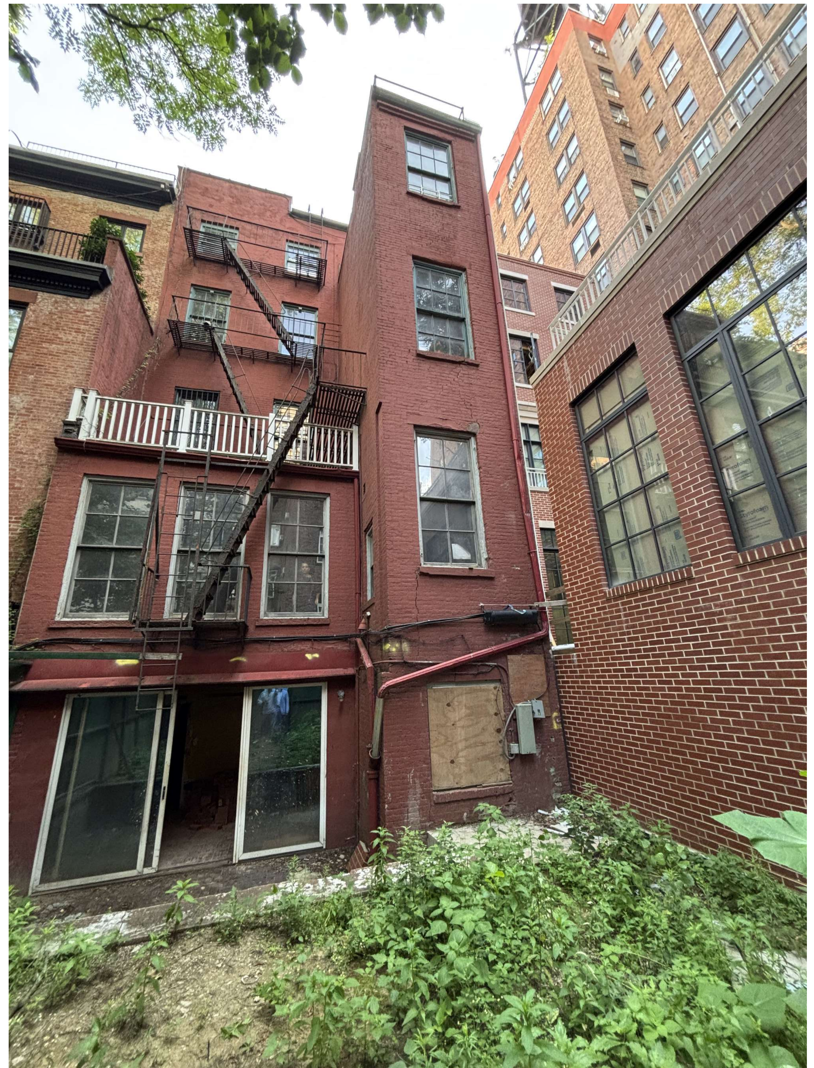
EXISTING REAR FACADE PHOTO
