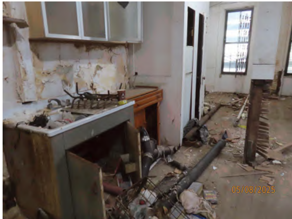
CURRENT CONDITION OF INTERIOR (TYPICAL)
