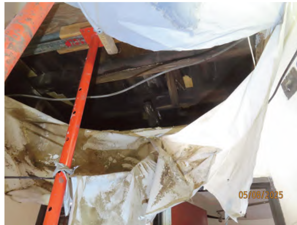
TYPICAL OVERHEAD CONDITION WITH SHORING JACK IN PLACE
