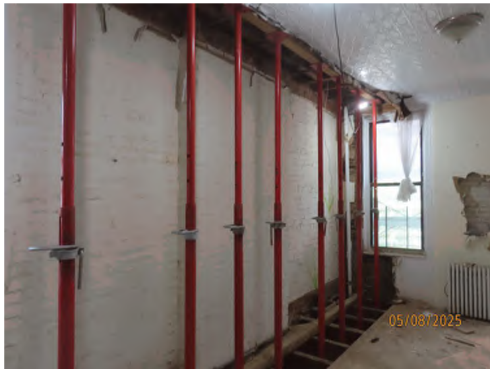
SHORING JACKS SPANNING TWO FLOORS
