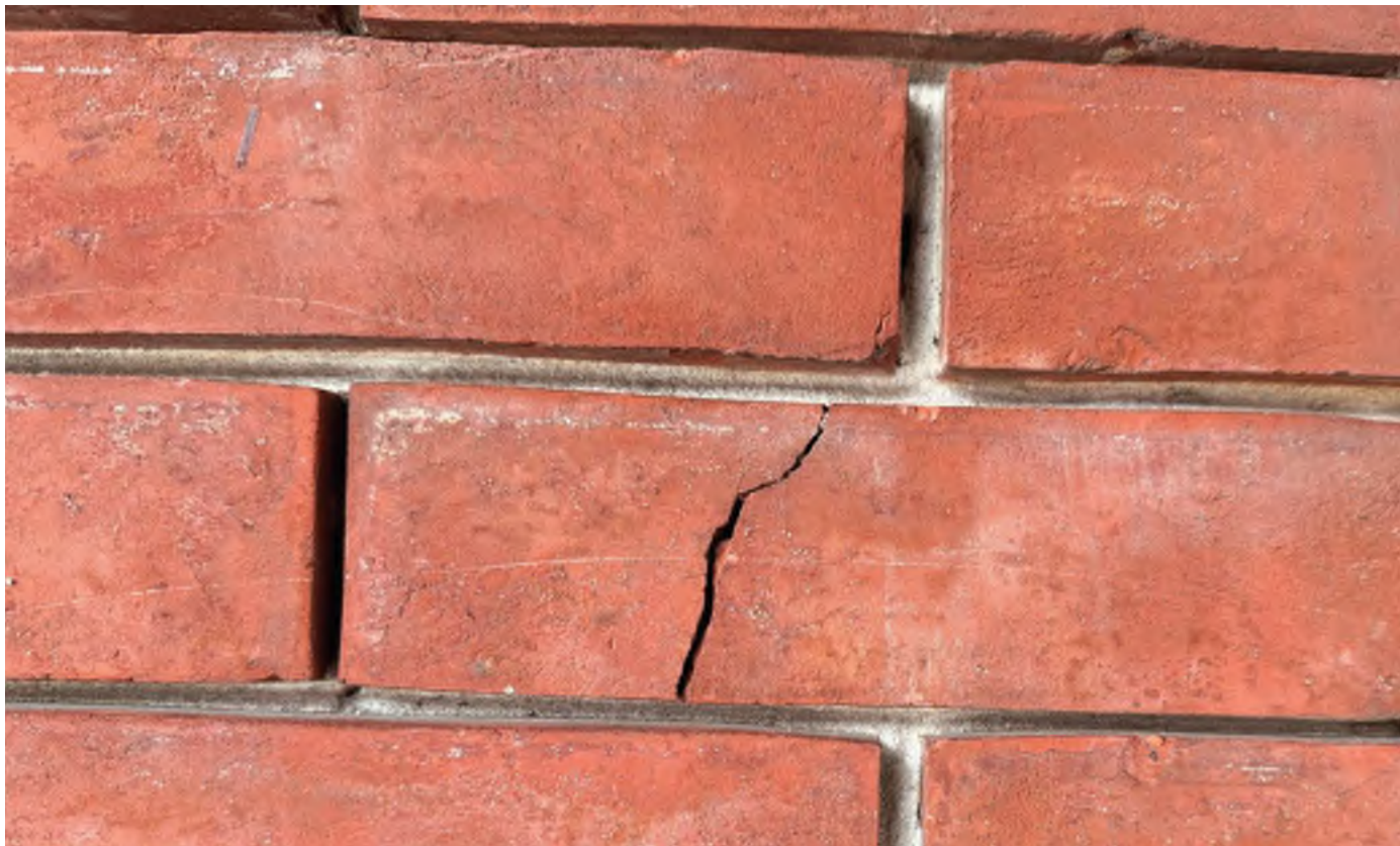
3 Brick Crack
