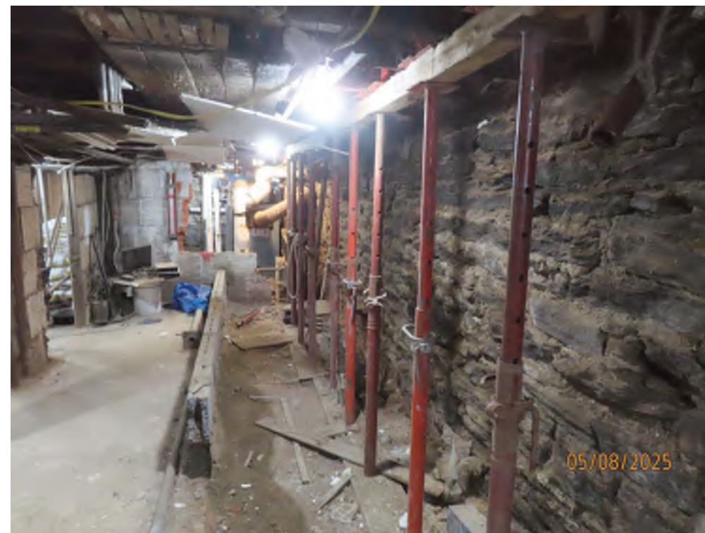
CURRENT CONDITION AT CELLAR
