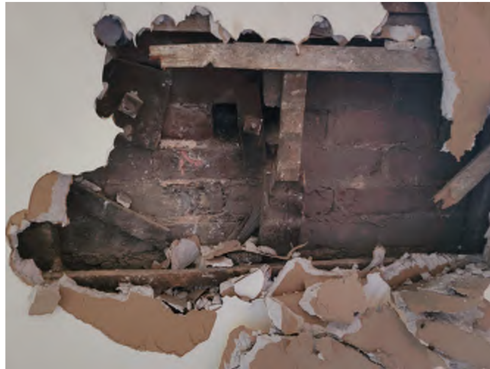
PROBE AT INTERIOR OF FACADE
