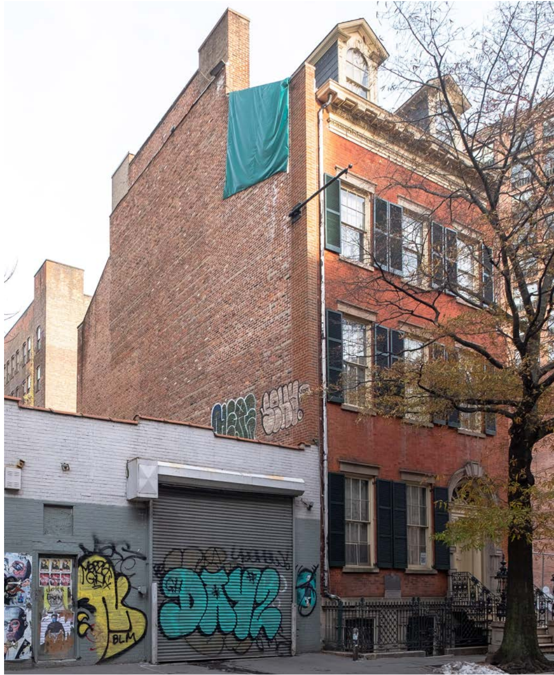
CURRENT LOT LINE WALL CONDITION
