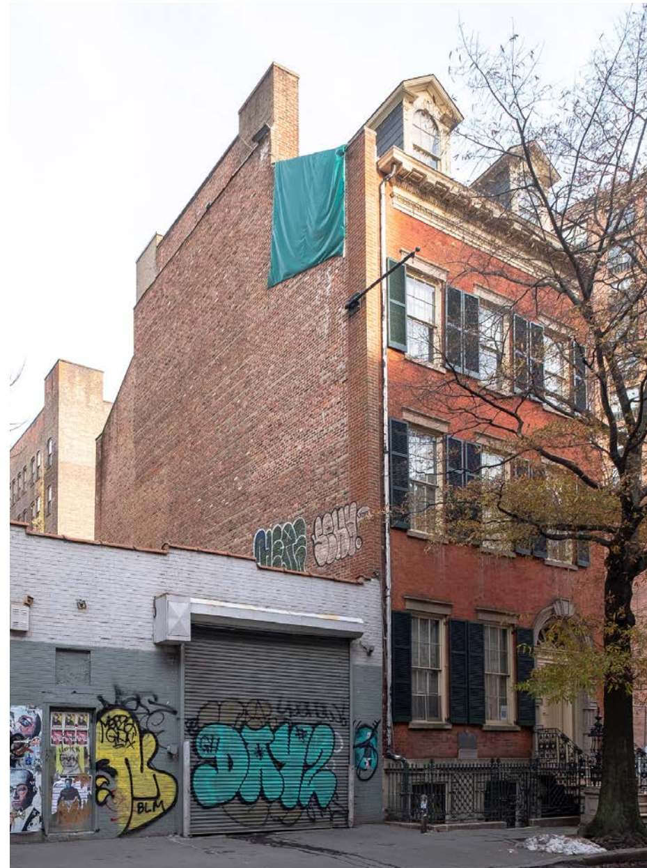
CURRENT LOT LINE WALL CONDITION
