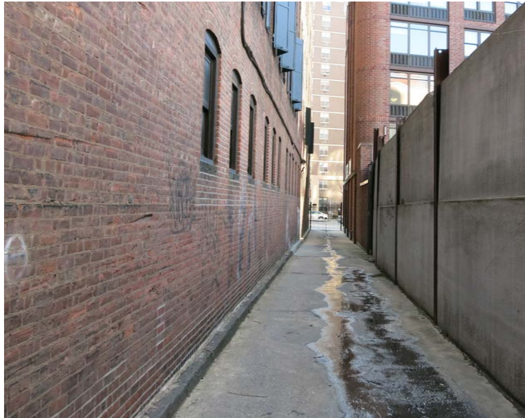
D - EXISTING CONDITIONS - STABLE COURT, ALLEY ACCESS TO BOWERY
