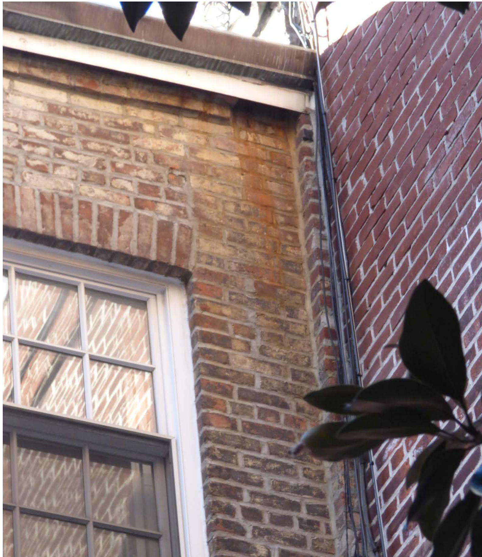
Existing Conditions - Rear Facade Details
