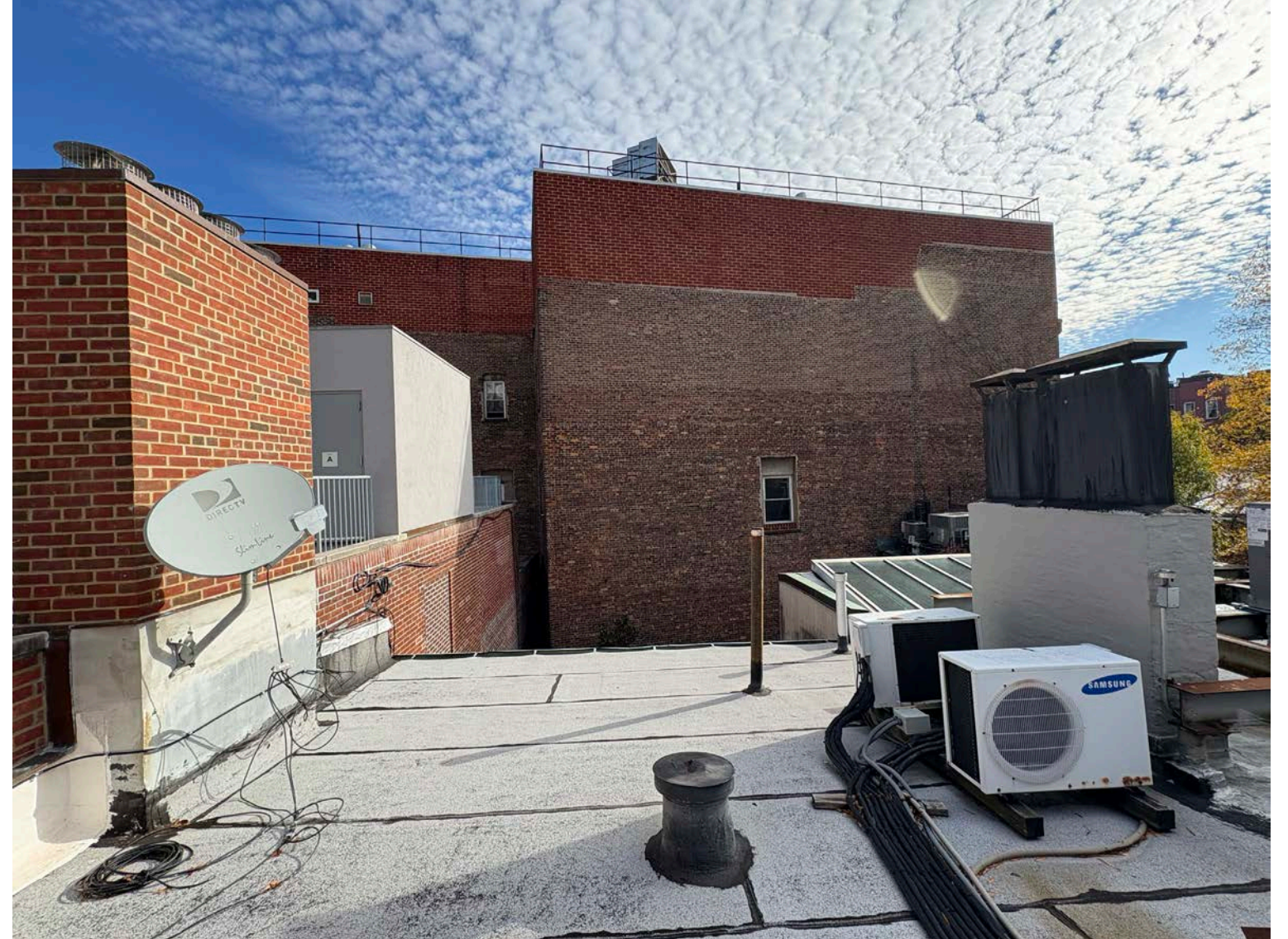
View of the roof - looking east
