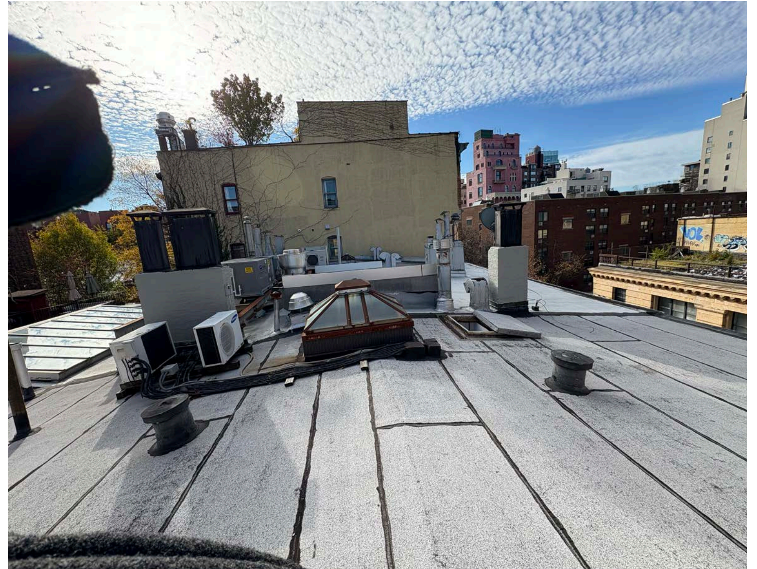
View of the roof - looking south
