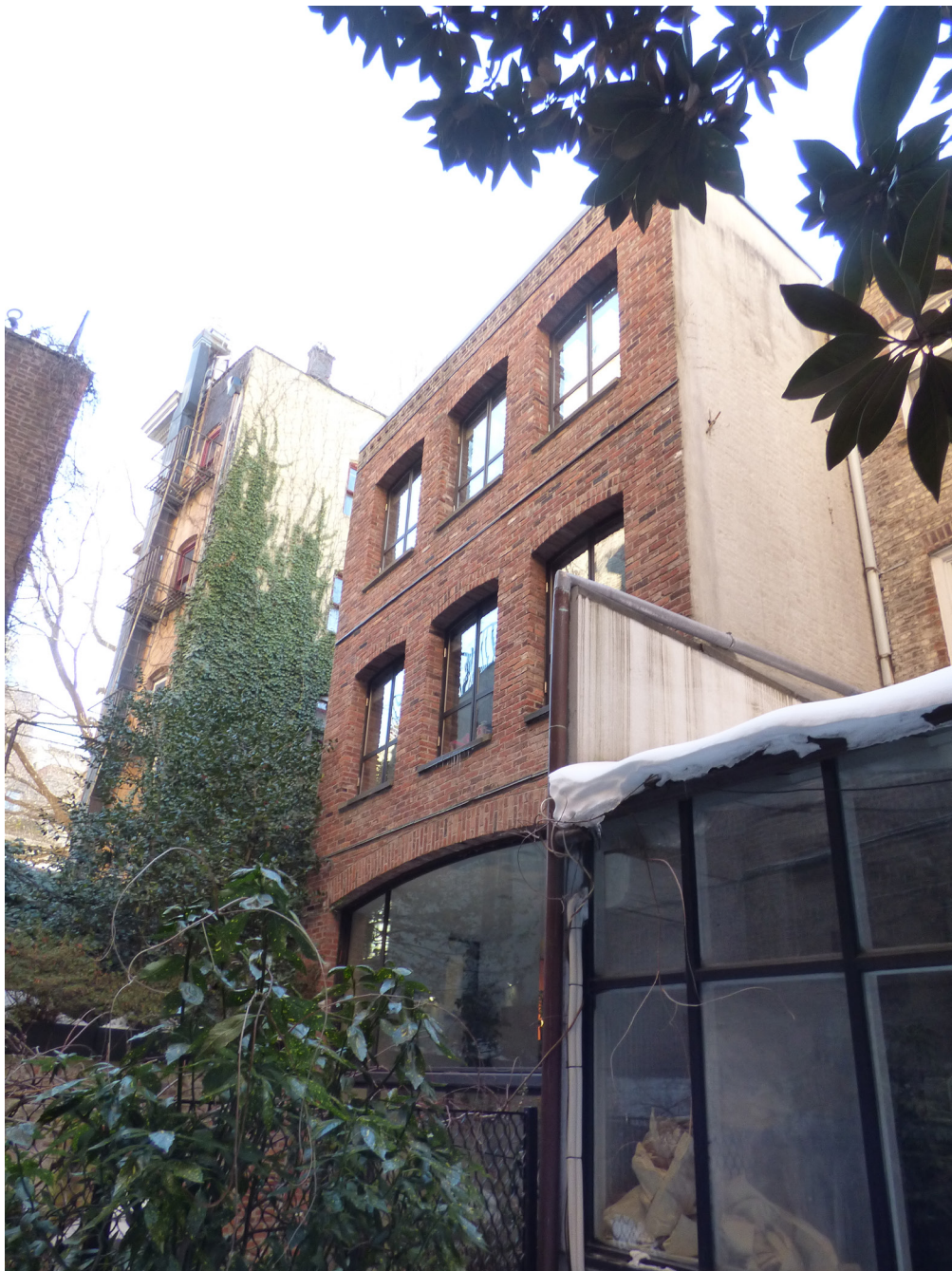
Rear yard, facing southwest
