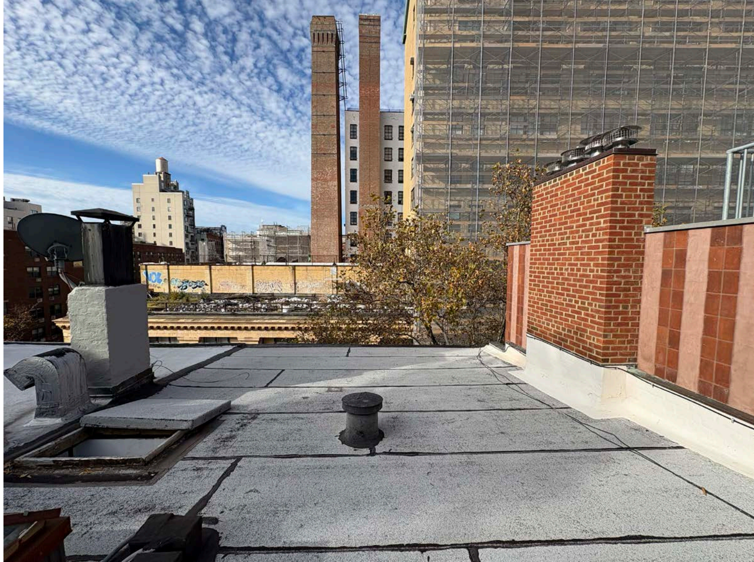
View of the roof - looking west
