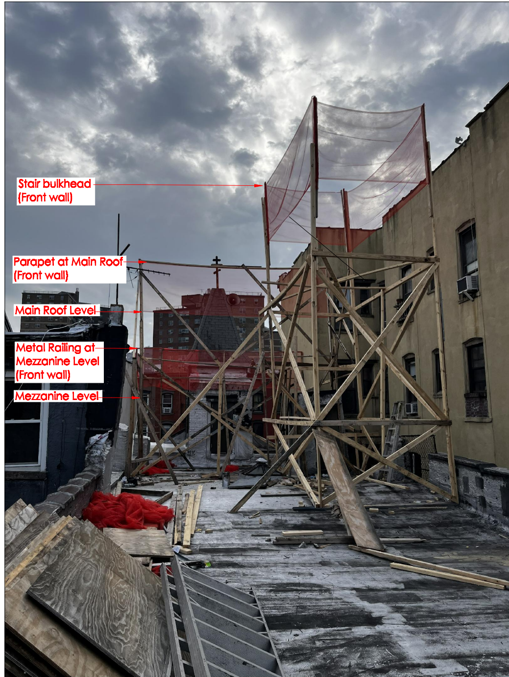
Rear view looking south at stair bulkhead
