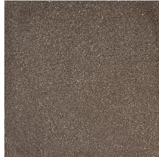
Brownstone masonry trim at front facade
