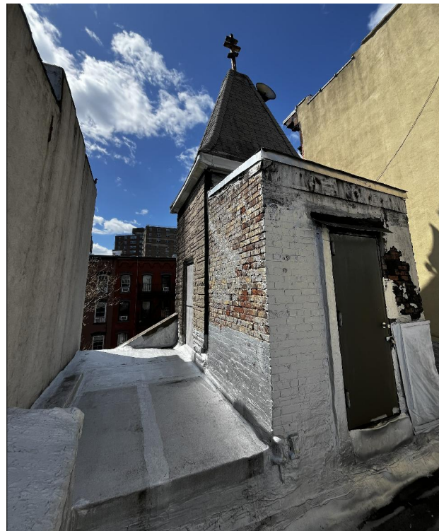
bell tower view at roof - east
