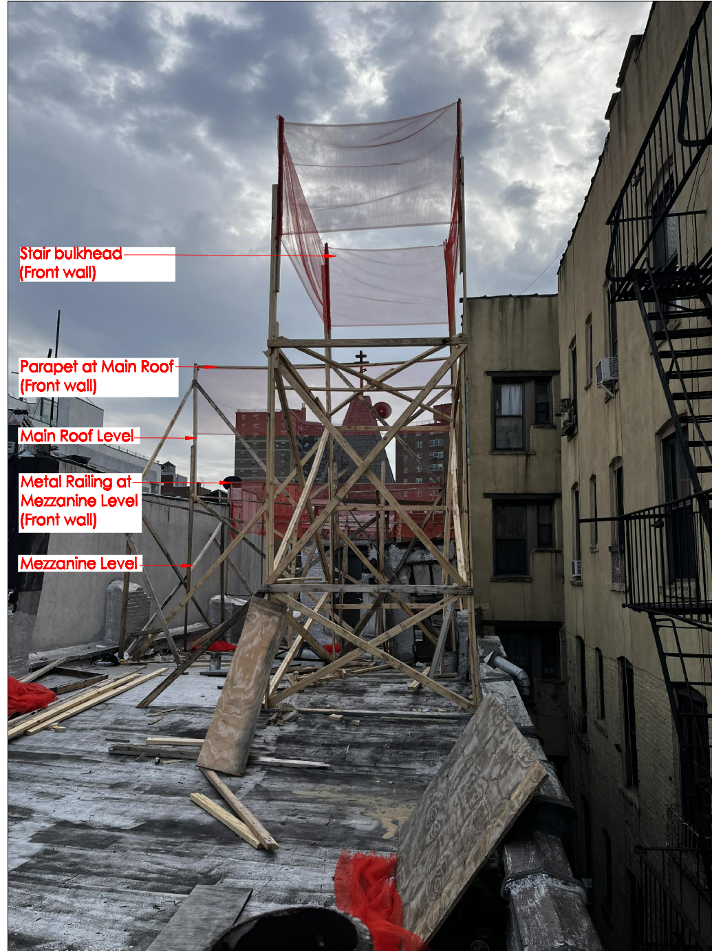
Rear view looking south at stair bulkhead
