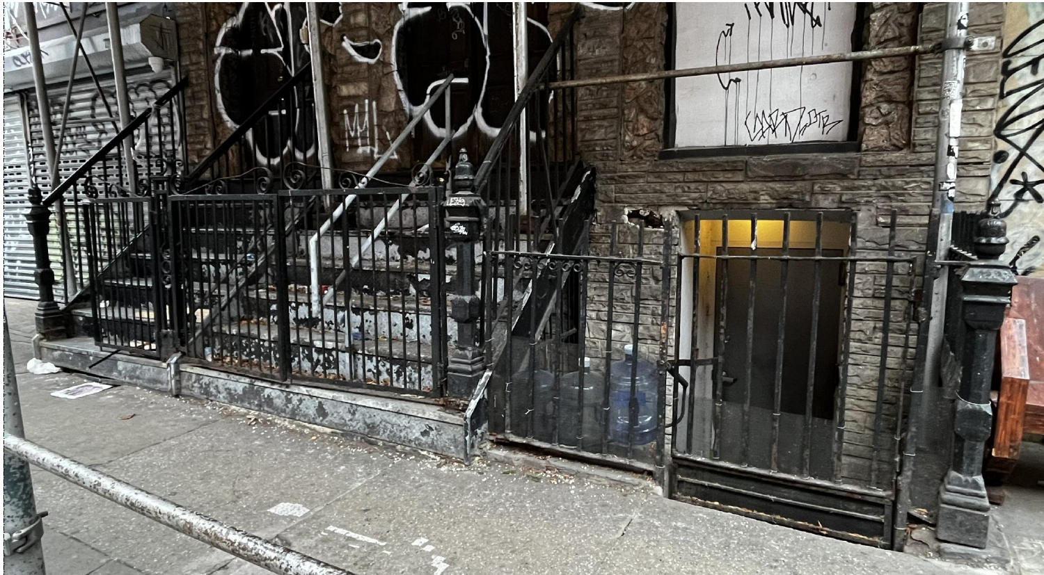
existing stoop at front areaway
