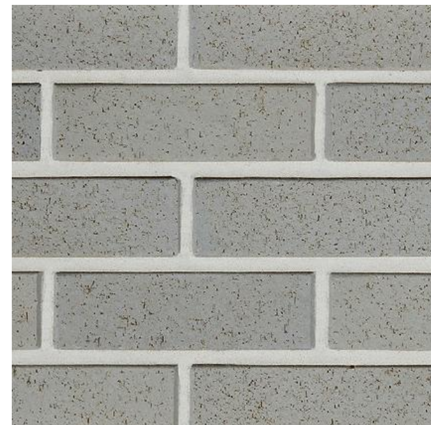
Existing brick facade
