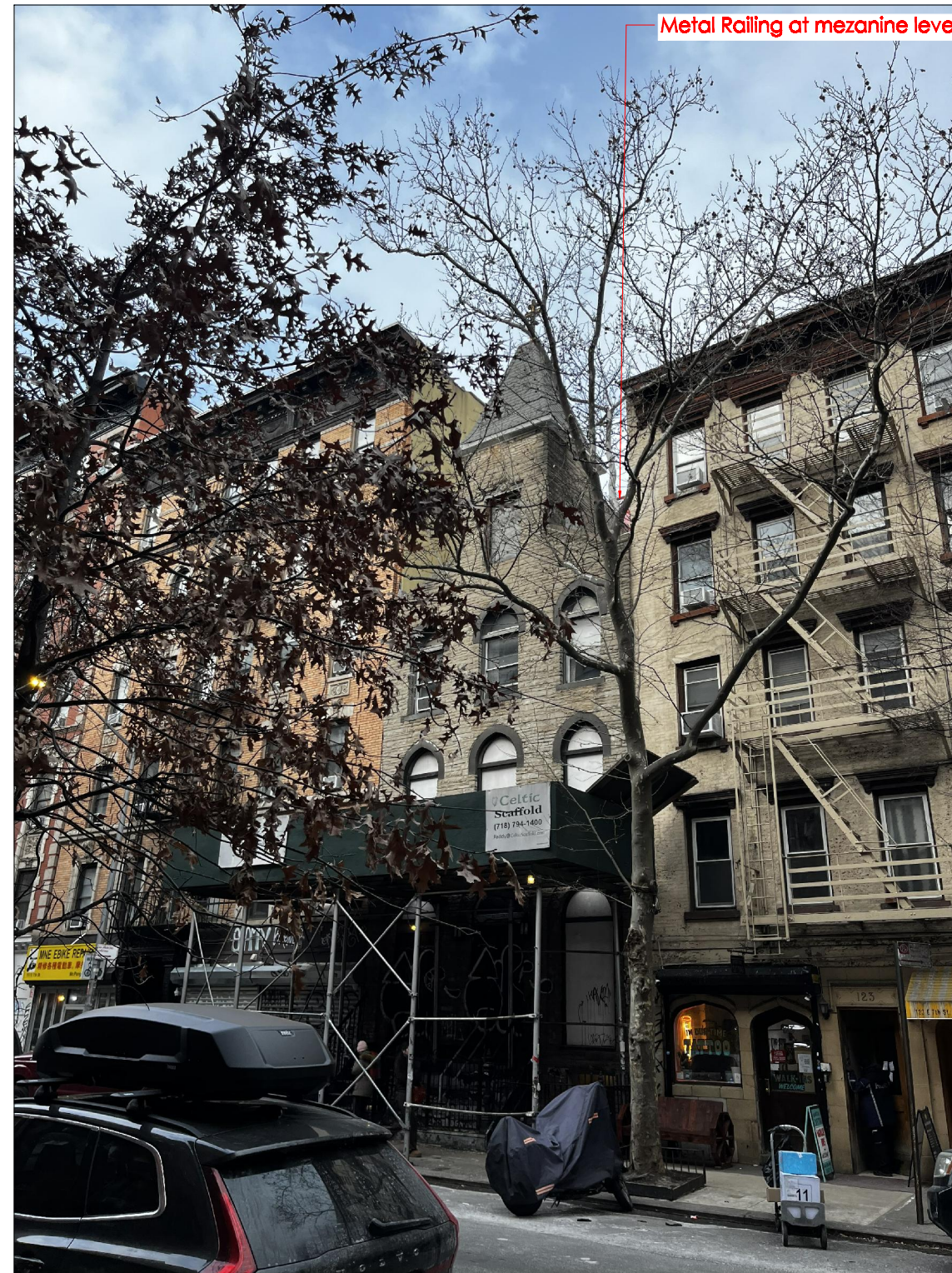
C. Street view looking east
