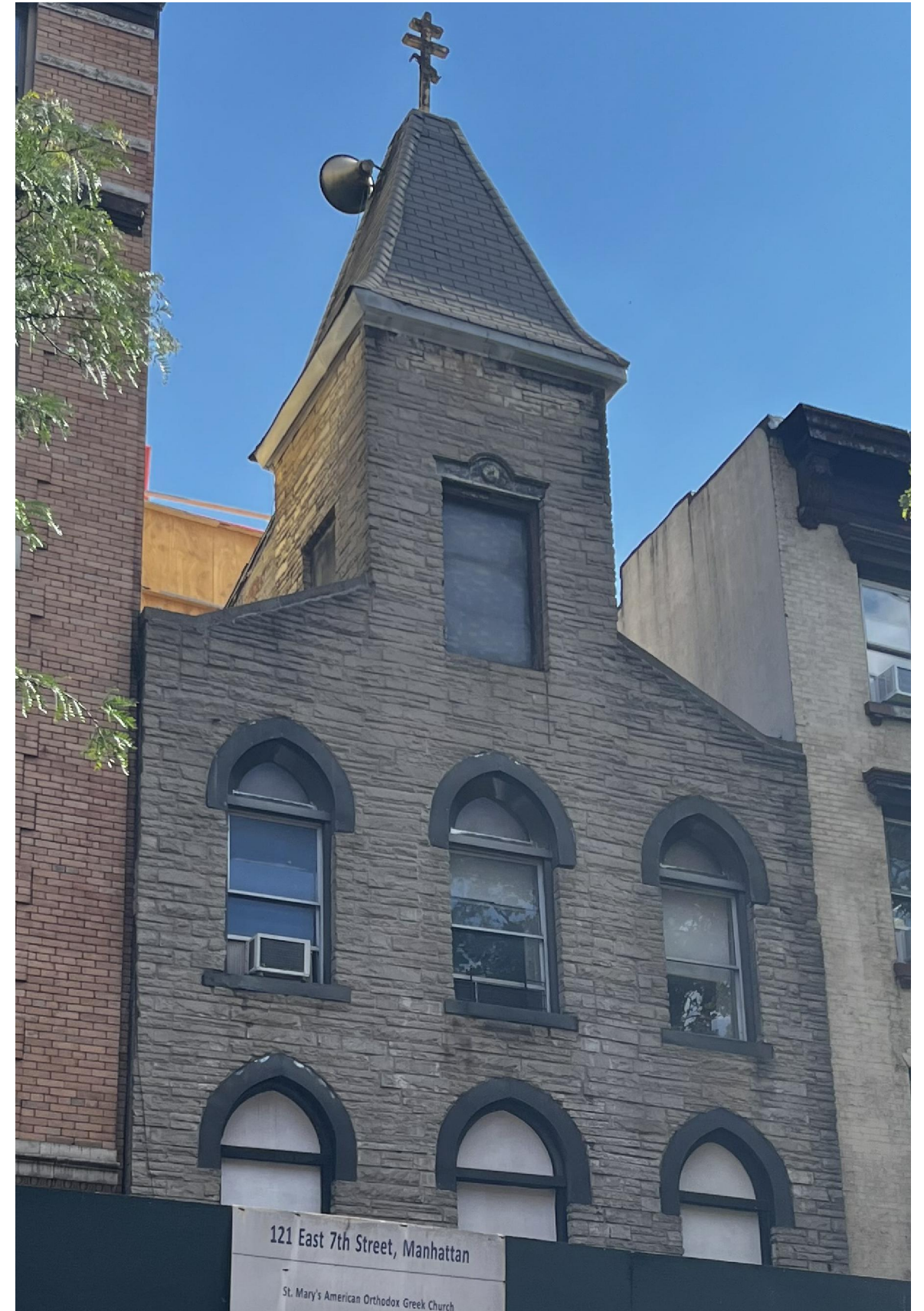
existing facade at 2nd & 3rd floor level & bell tower
