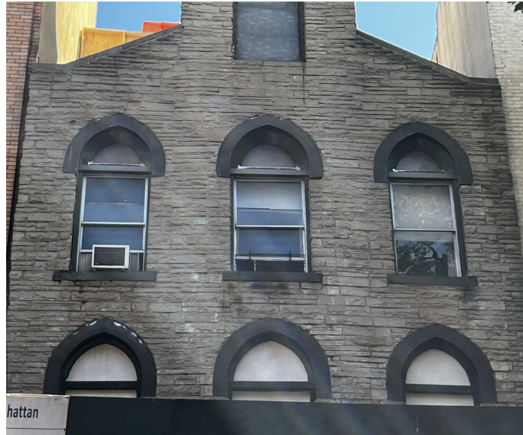
view at 2nd floor stained glass window & transom
