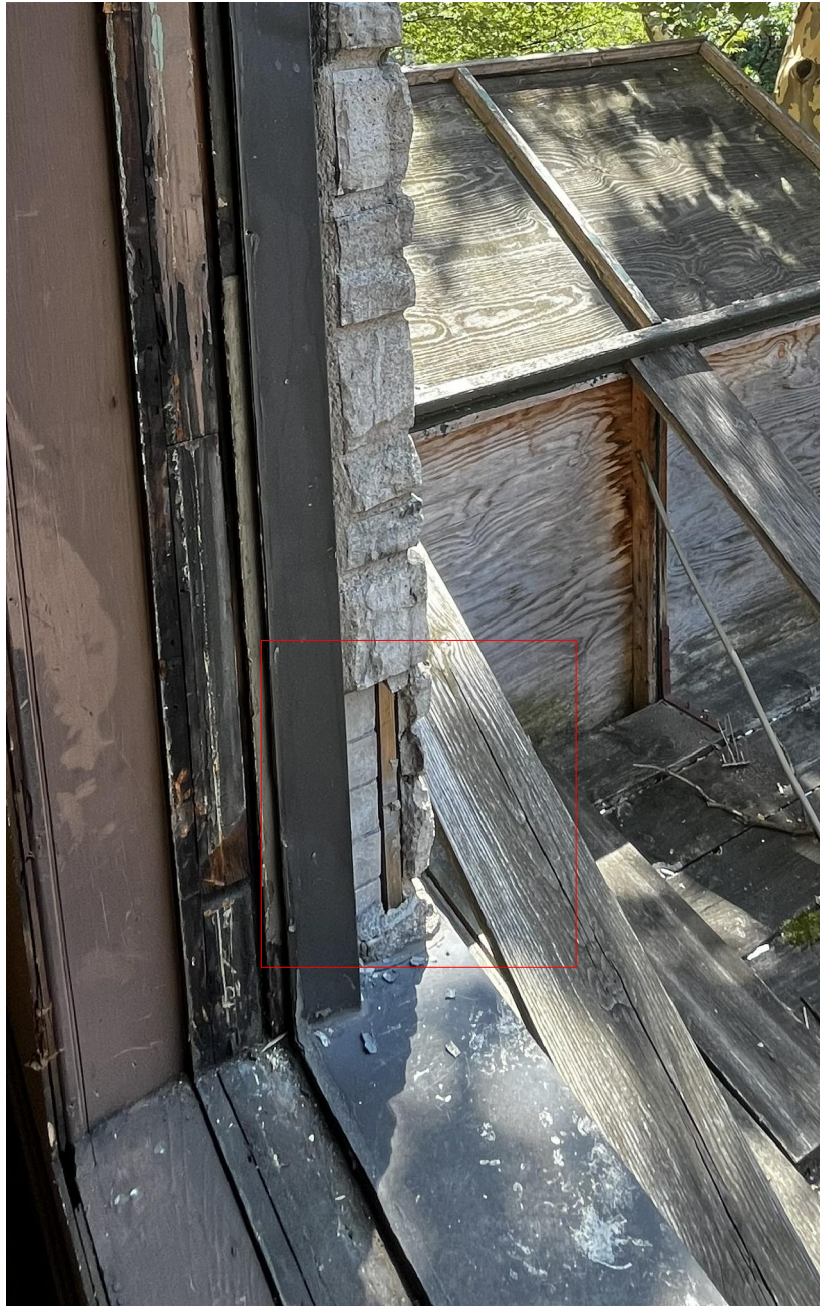
Interior view at 2nd floor window
