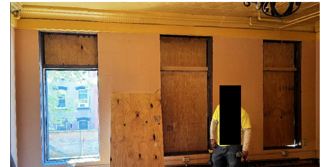
view from interior
