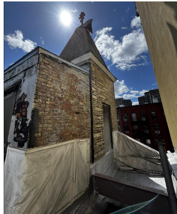
bell tower view at roof - west
