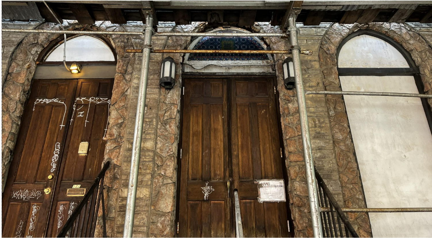
existing facade at 1st floor level
