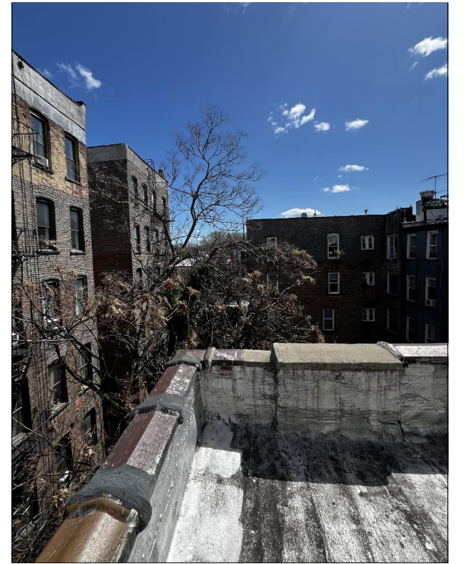
rear east view at roof
