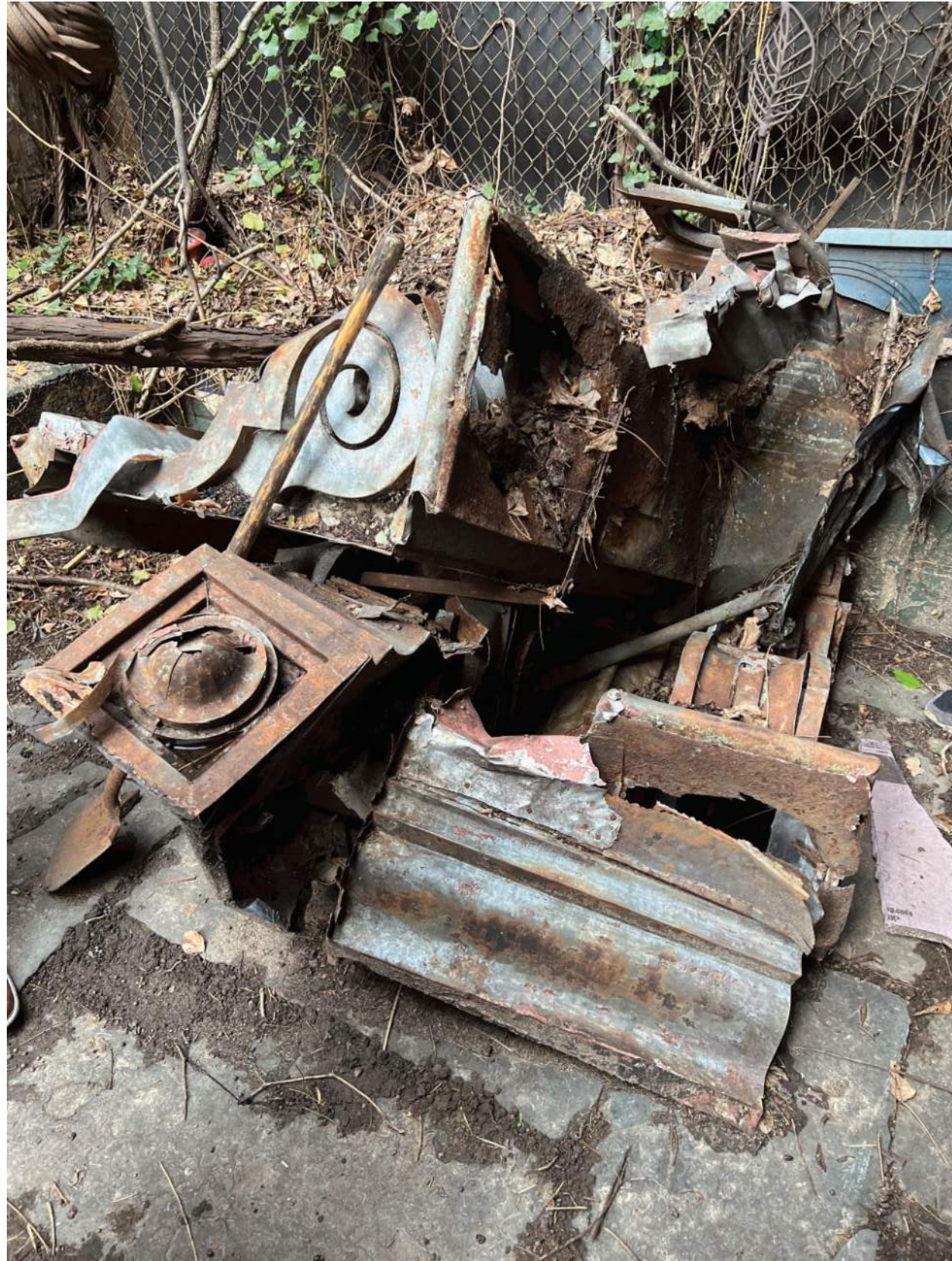
RUBBLE PILE IN REAR YARD, CONSISTING OF ORIGINAL FACADE
