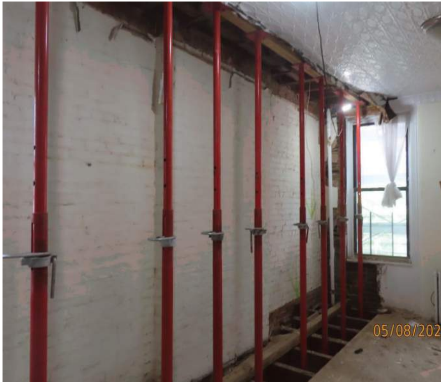
C. SHORING JACKS SPANNING TWO FLOORS
