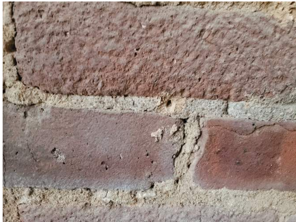
DETAIL OF MASONRY FOLLOWING PIN TEST
