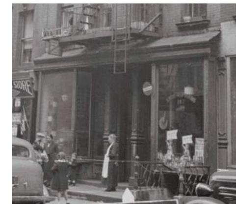
HISTORICAL IMAGE OF 137 THOMPSON STREET STOREFRONT
