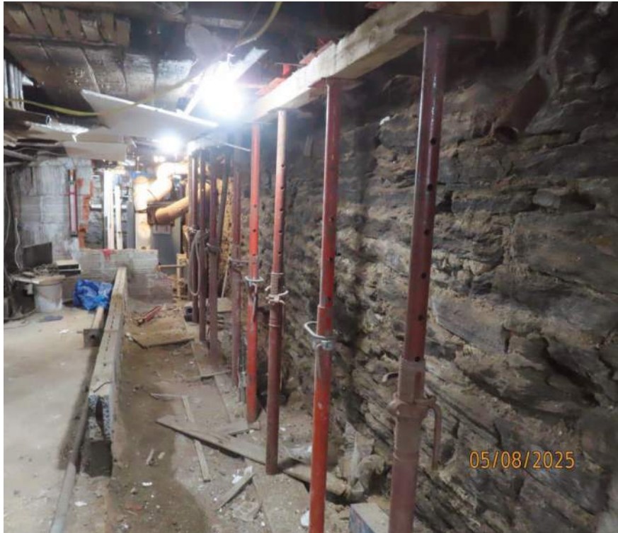
A. CURRENT CONDITION AT CELLAR
