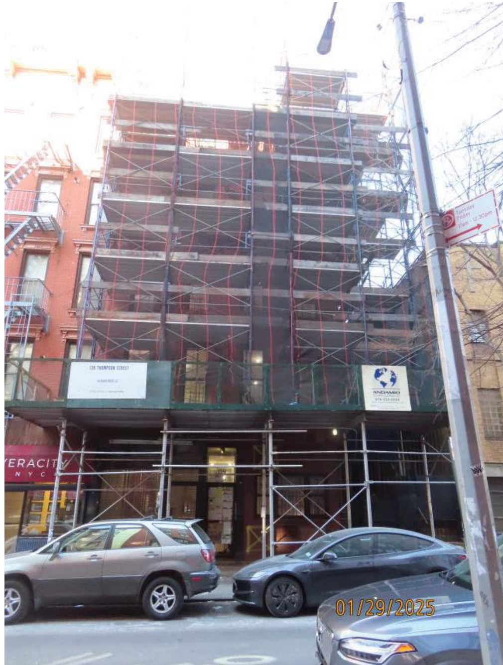
FRONT FACADE WITH SCAFFOLDING
