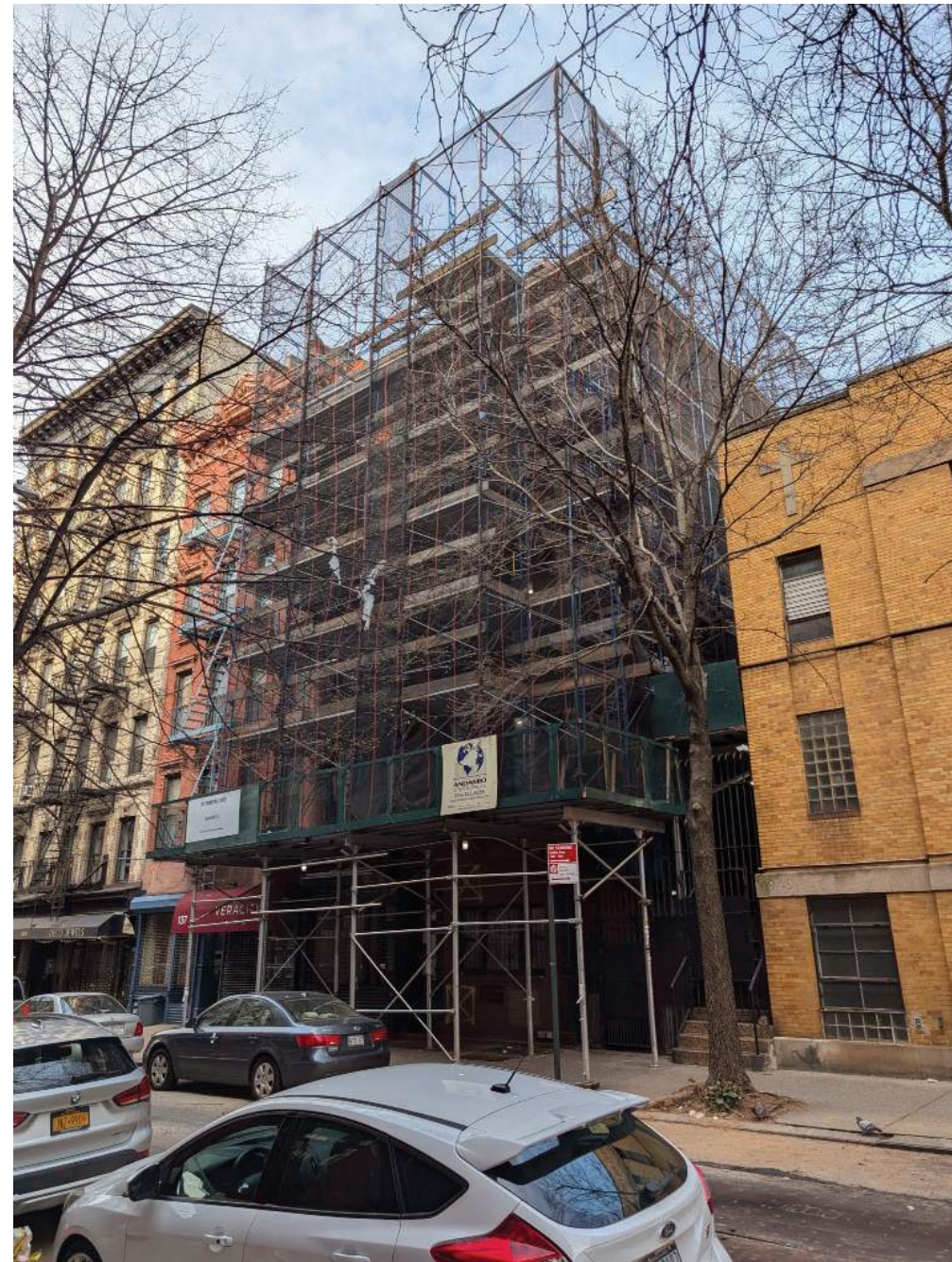
FRONT FACADE WITH SCAFFOLDING
