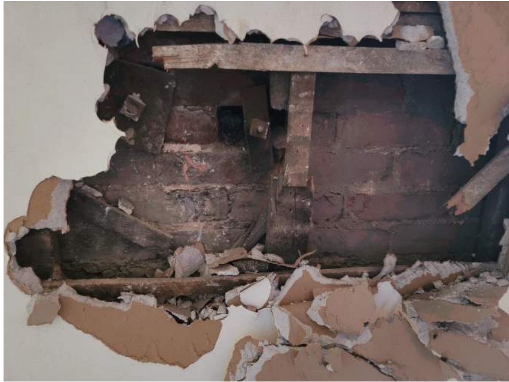
PROBE AT INTERIOR OF FACADE
