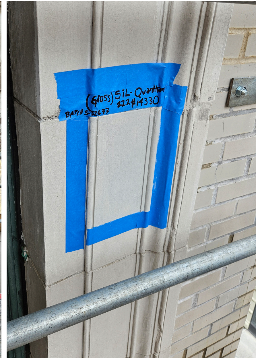
Custom coating to match existing Edison Coatings Inc. Aquathan breathable coating
