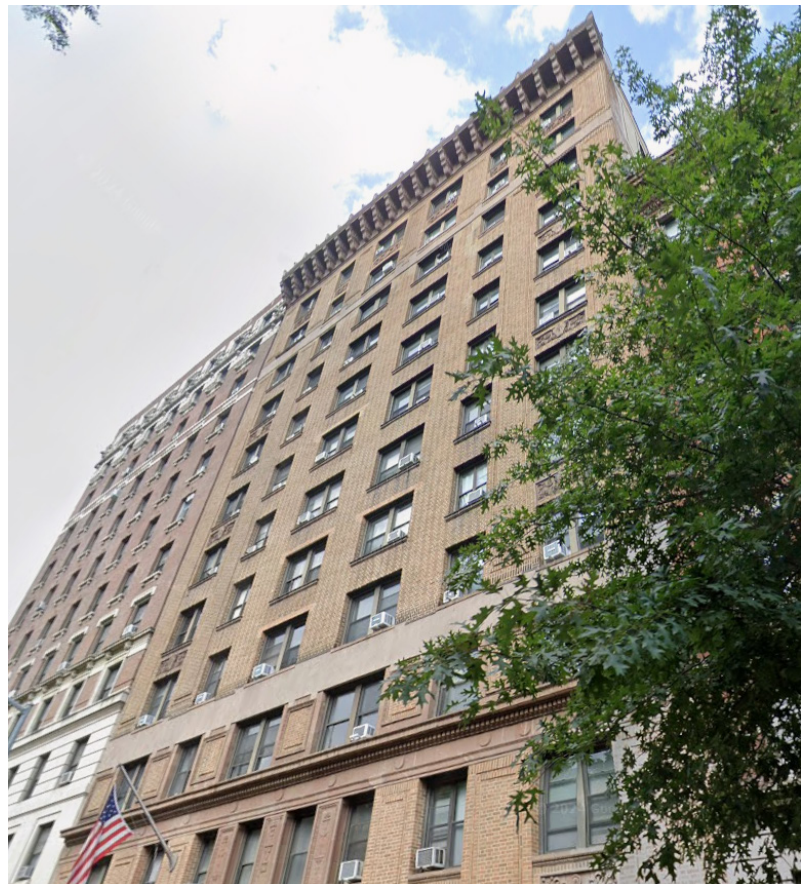
949 West End Avenue, NYC Riverside-West End Historic District Extension II
