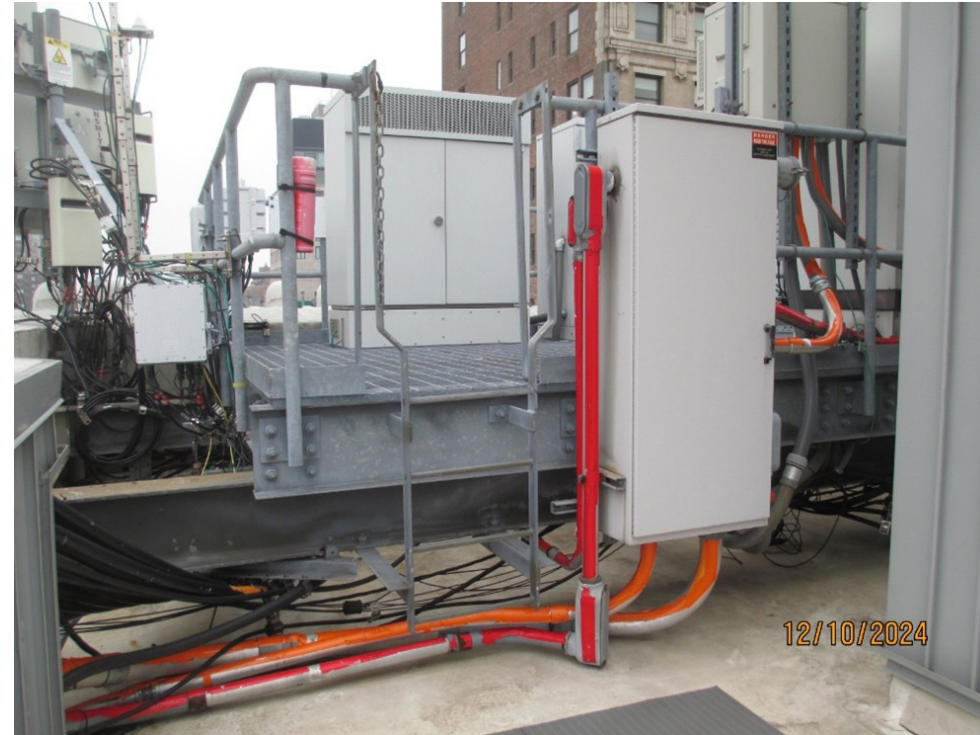
East parapet roof dunnage
