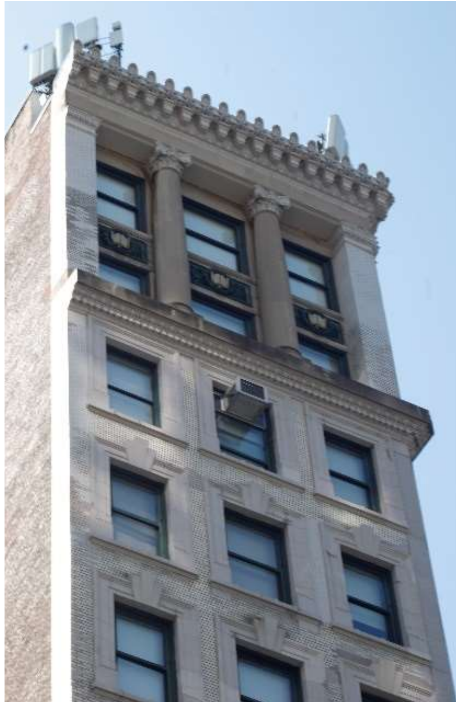
View of parapet cornice (Image from NYC LPC Designation Report)
