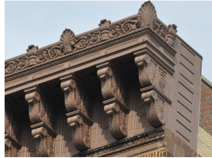
Seal Reinforced Fiberglass, Inc. GFRP Replaced Terracotta Cornice
