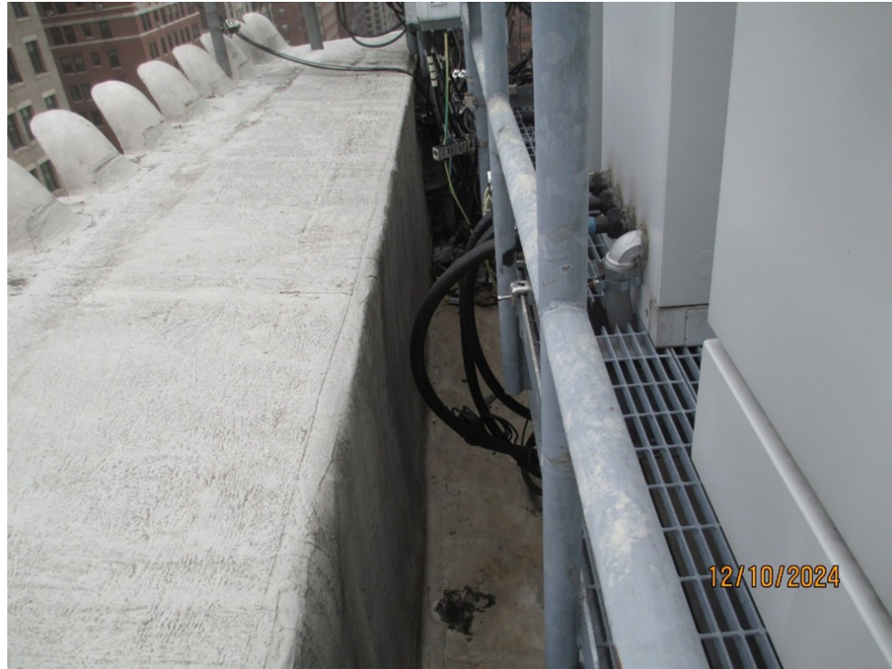
East parapet roof dunnage
