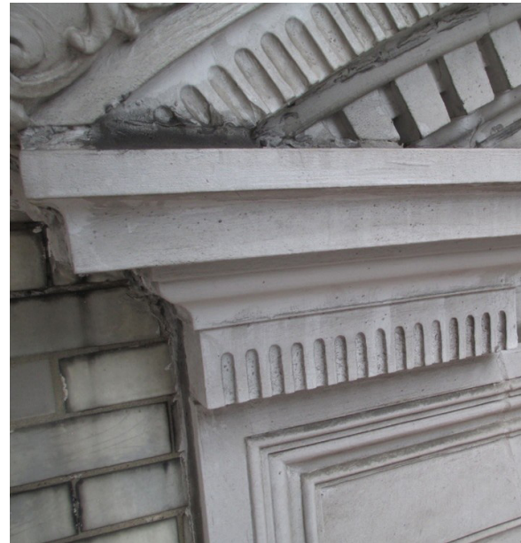
Painted window surrounds
