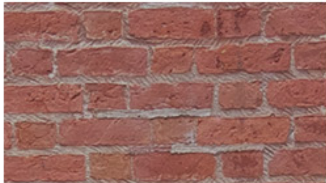
Existing Restored Brick 85 Sullivan Areaway
