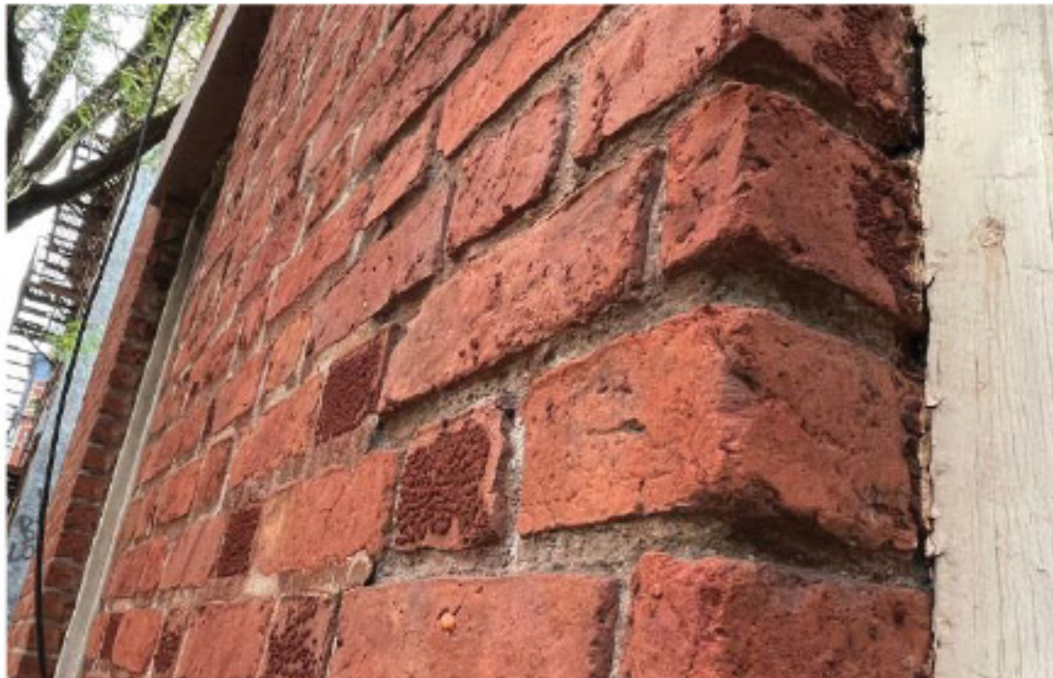
Mortar Erosion
