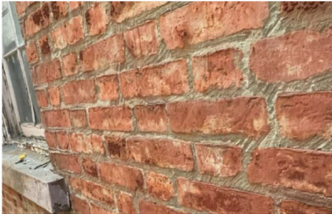
Mechanically Scraped Bricks
