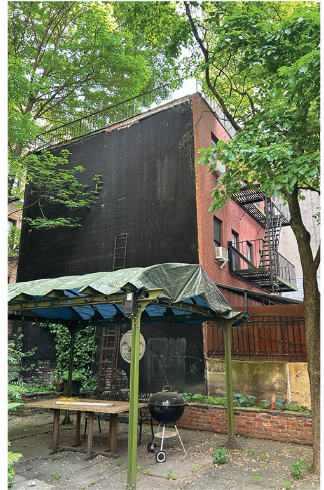
Existing Rear Building at 81 Sullivan Street
