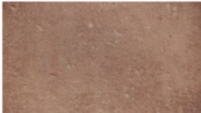
Restored Brownstone 83 & 85 Sullivan Sills and Lintels
