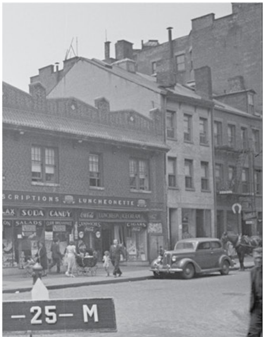
Spring Street - Federal Style context Source: NYCMA 1940 Tax Photo
