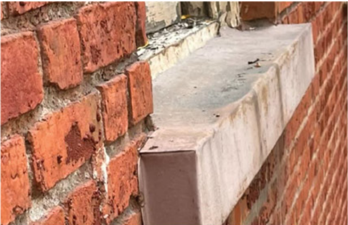
Sill Covered in Break Metal
