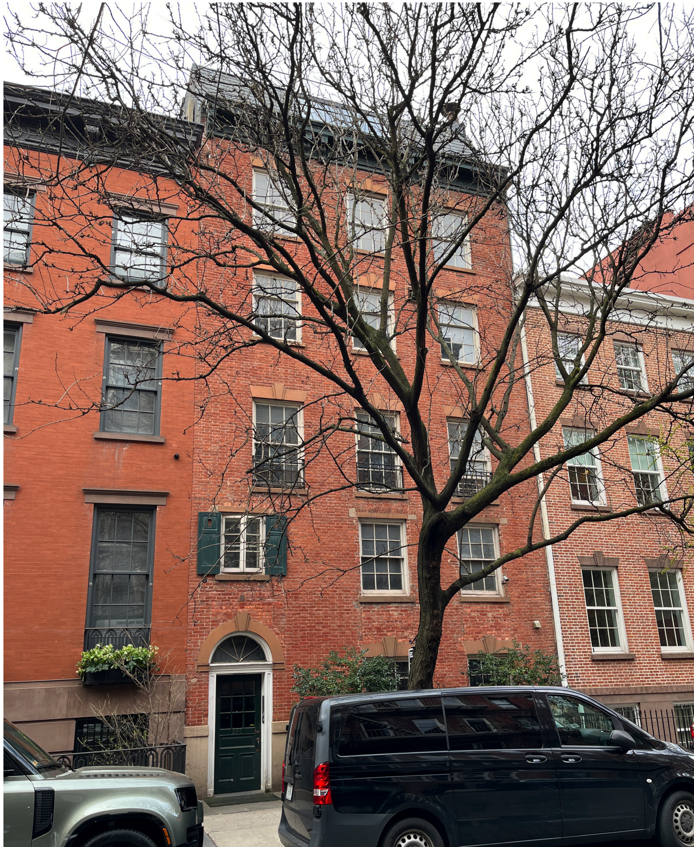
1. EXISTING FACADE OF 280 WEST 11TH STREET
