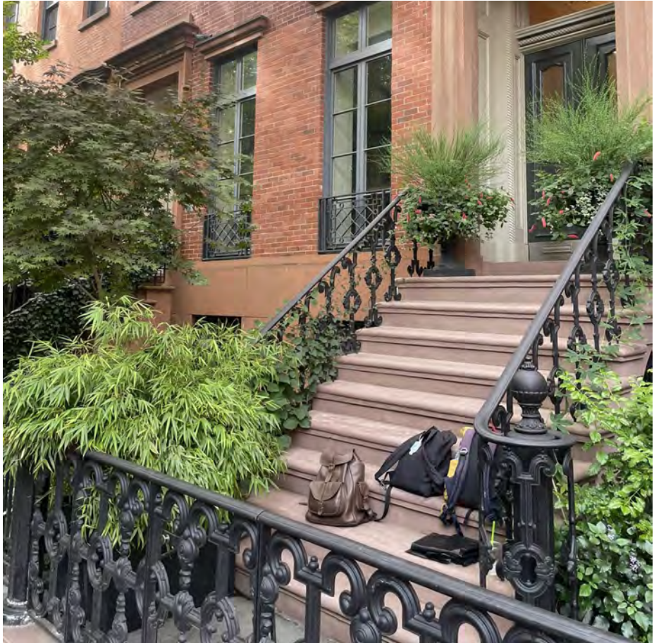
13 Bank Street Existing Ironwork
