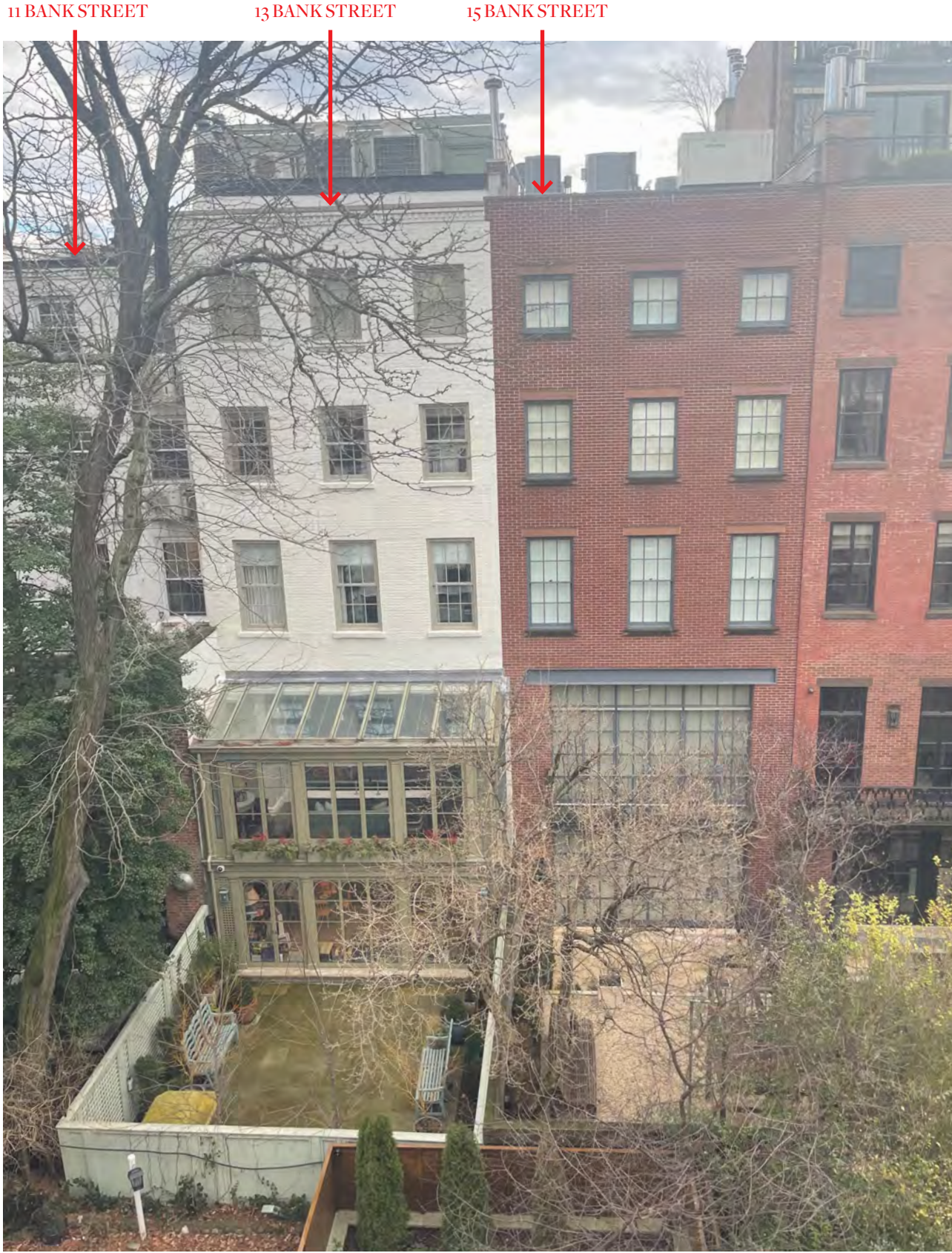
Existing conditions at 13 and 15 Bank Street
