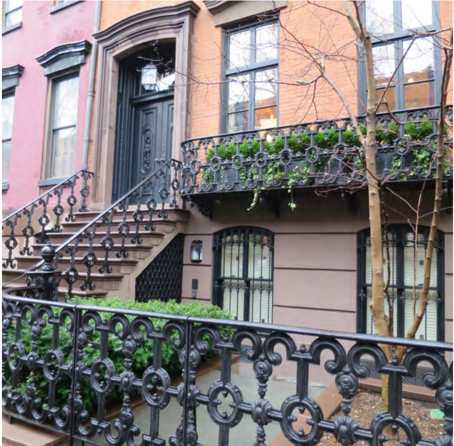
17 Bank Street Existing Ironwork
