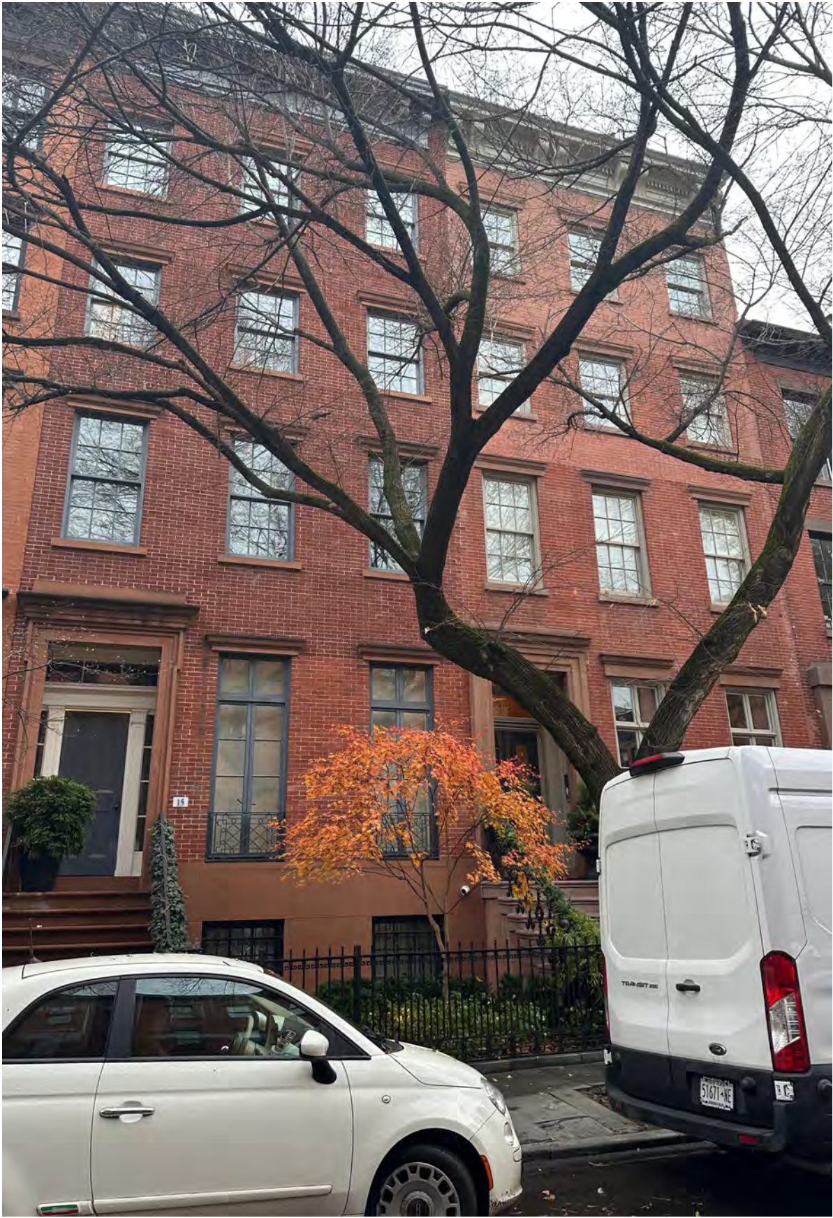
15 Bank Street (Left) And 13 Bank Street (Right)
