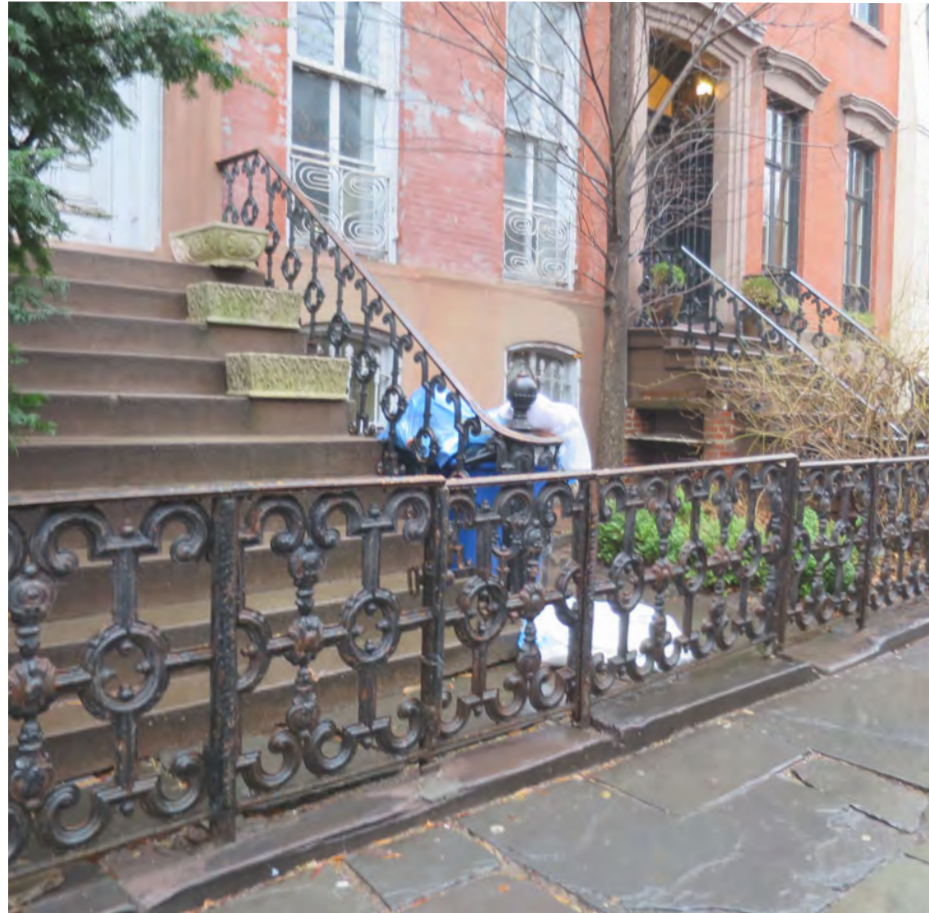
25 Bank Street Existing Ironwork
