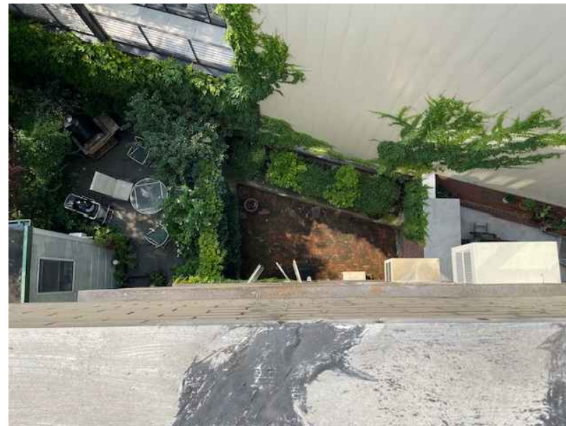
5 SOUTH VIEW FROM ROOF OVERLOOKING REAR YARD
