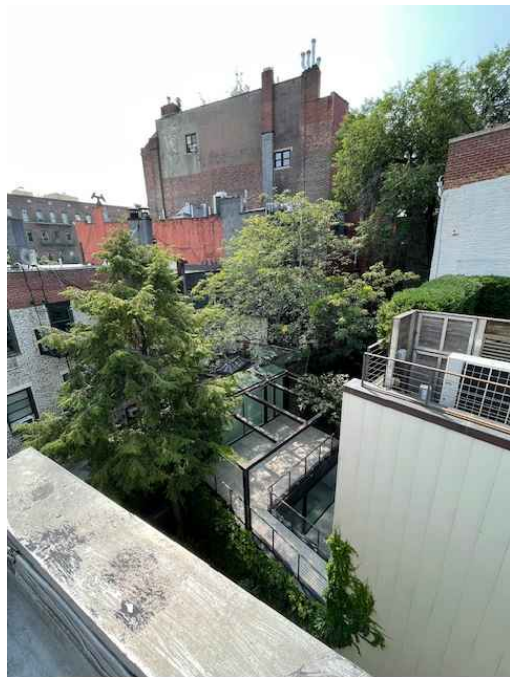
4 SOUTH EAST VIEW FROM ROOF OVERLOOKING REAR YARDS
