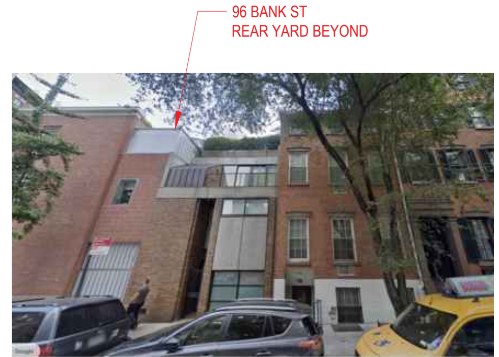
3 STREET VIEW OF PROPERTY FROM GREENWICH STREET
