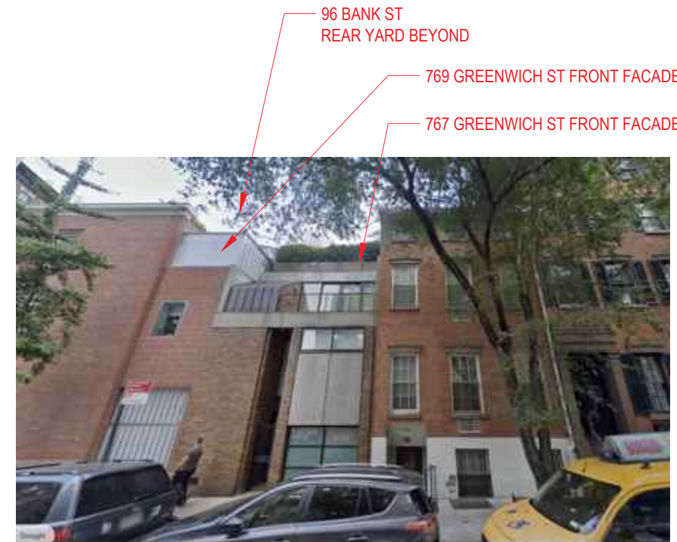
3 STREET VIEW OF PROPERTY FROM GREENWICH STREET
