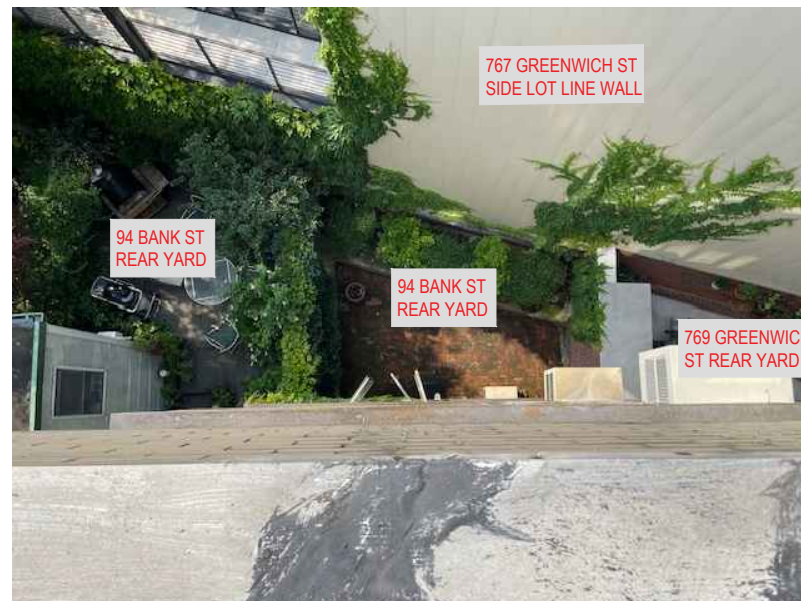
5 SOUTH VIEW FROM ROOF OVERLOOKING REAR YARD
