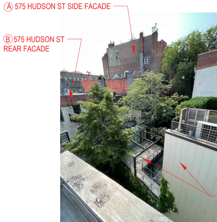
4 SOUTH EAST VIEW FROM ROOF OVERLOOKING REAR YARDS
