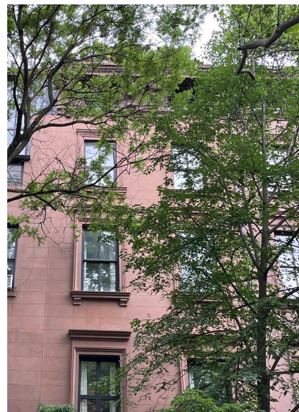
4. VIEW OF MOCKUP FACING SOUTHEAST; MOCKUP NOT VISIBLE
