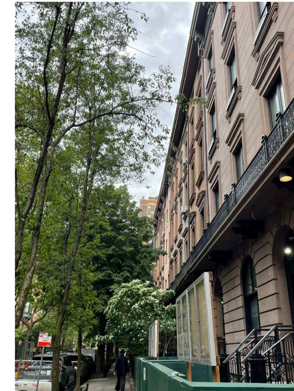
3. VIEW OF MOCKUP FACING SOUTHWEST; MOCKUP NOT VISIBLE
