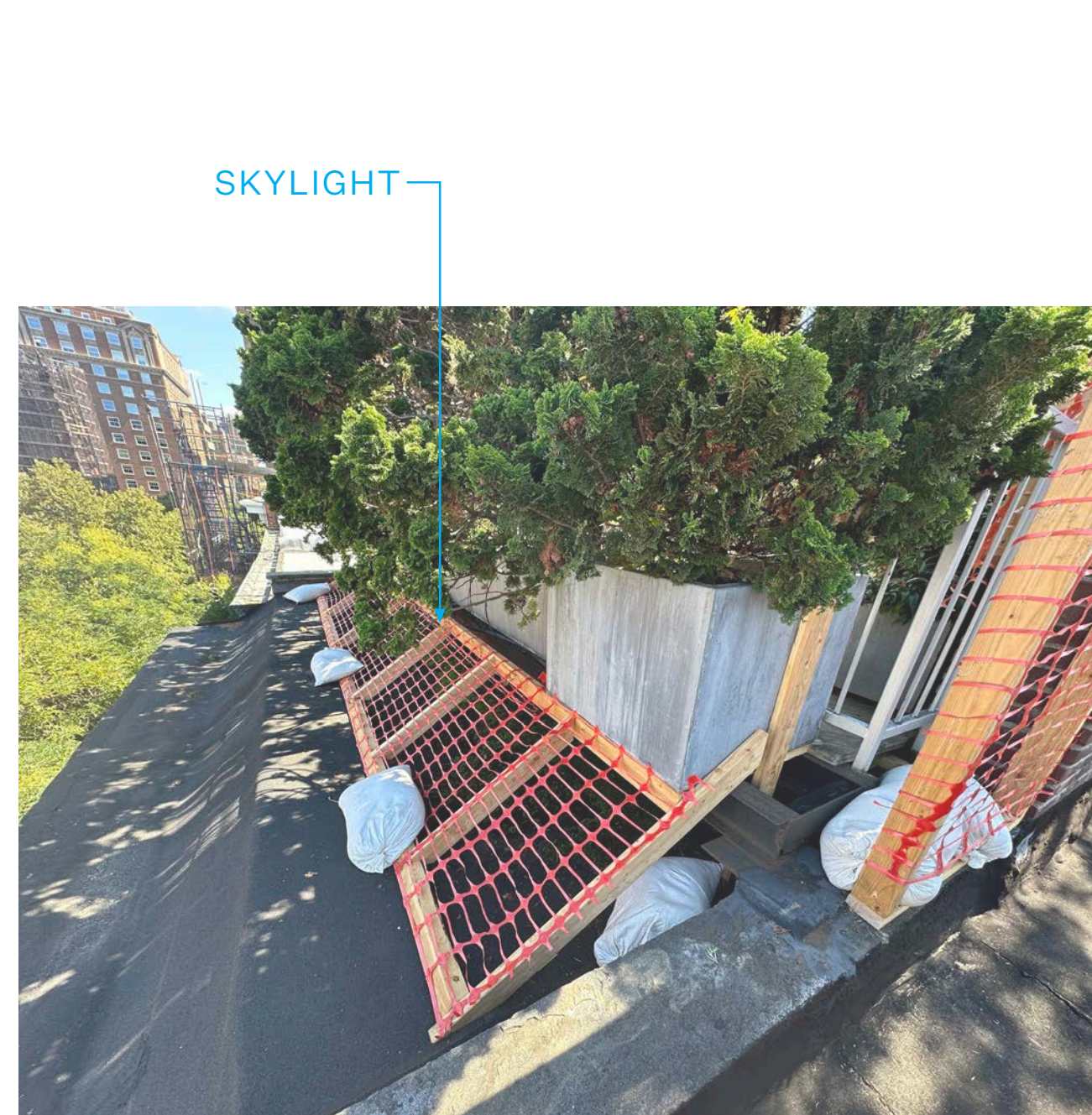
4. VIEW FACING EAST SHOWING SKYLIGHT & RAILING PREVIOUSLY APPROVED SKYLIGHT
