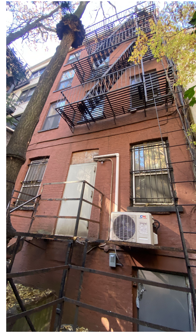
104 GREENWICH AVE NYC EXISTING PHOTO (REAR)
