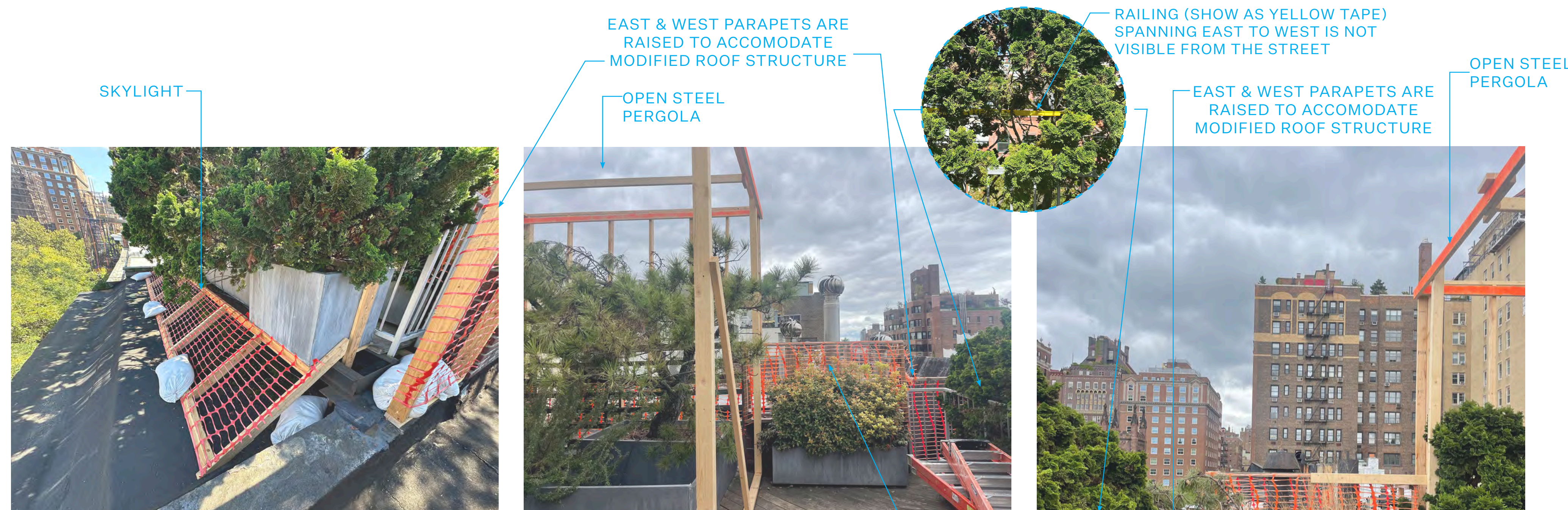
4. VIEW FACING EAST SHOWING SKYLIGHT & RAILING
