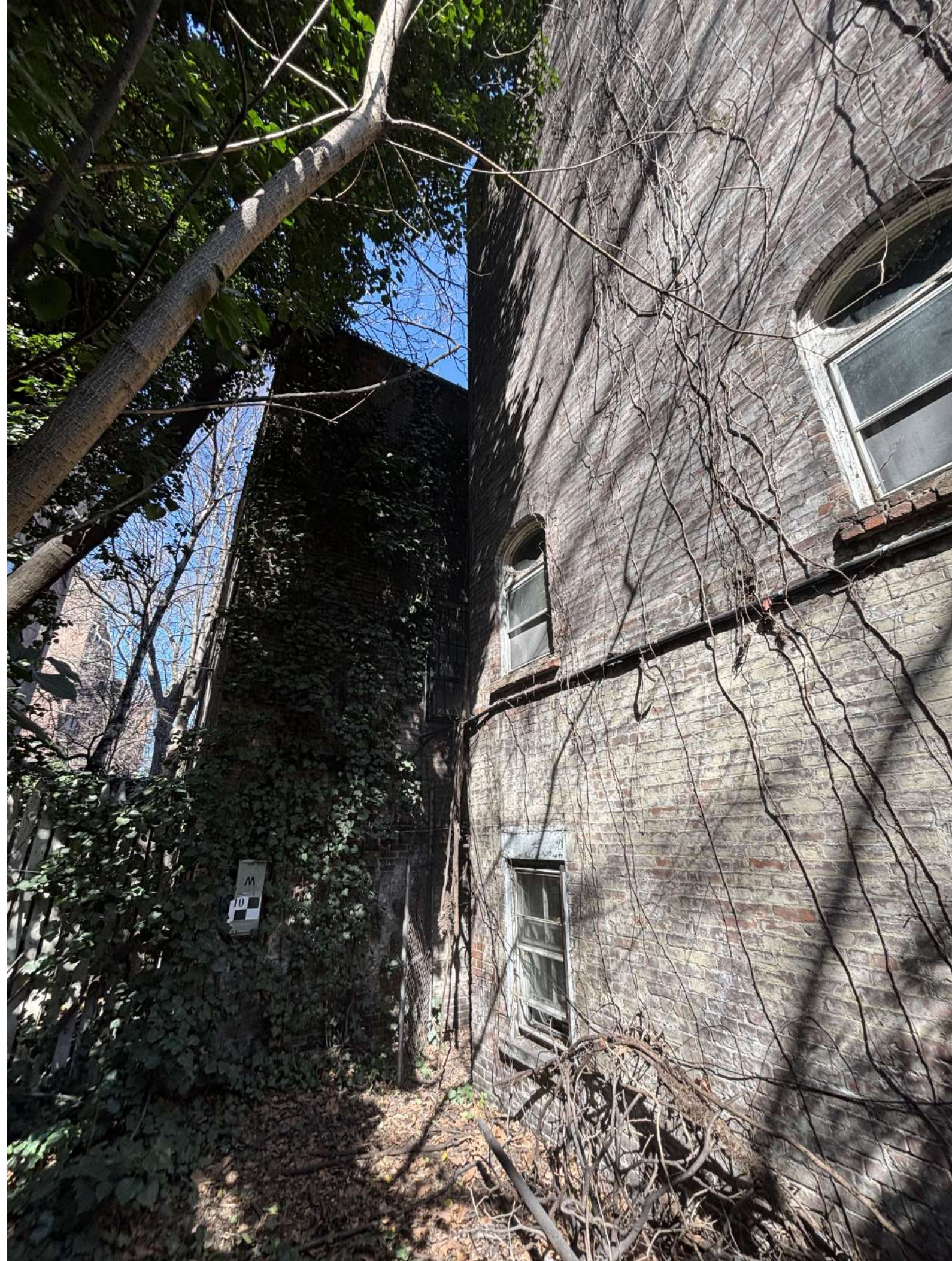
EXISTING 12'-5" REAR YARD LOOKING WEST
