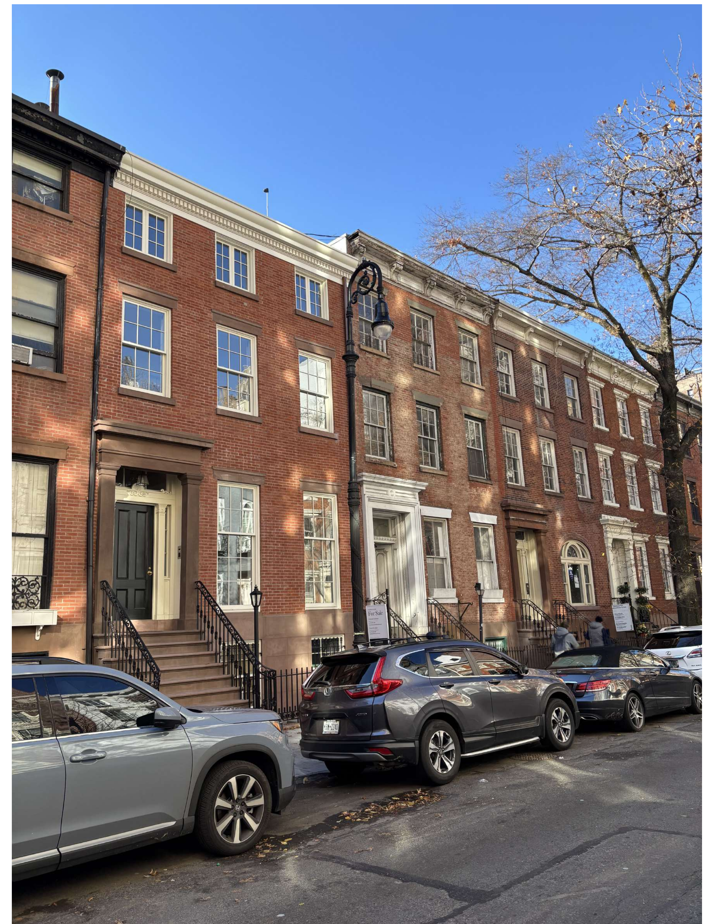
VIEW OF 36 W11TH STREET ORIGINALLY BUILT AS PART OF A ROW OF FIVE (NOS. 36-44) BUILT BY JAMES HARRIOT, 1840-41 3 STORY W/BASEMENT GREEK RIVALRY STYLE W/BACKETED ROOF CORNICE & ATTIC STORY
