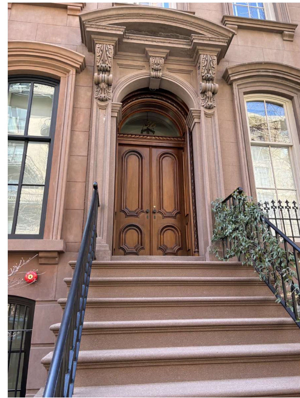
DOOR & STOOP RESTORATION - 36 W12TH
