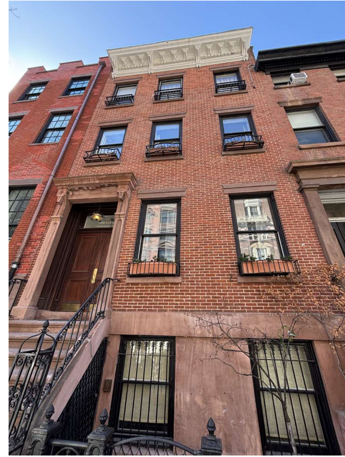
BRICK CLEANING & POINTING - 30 W11TH
