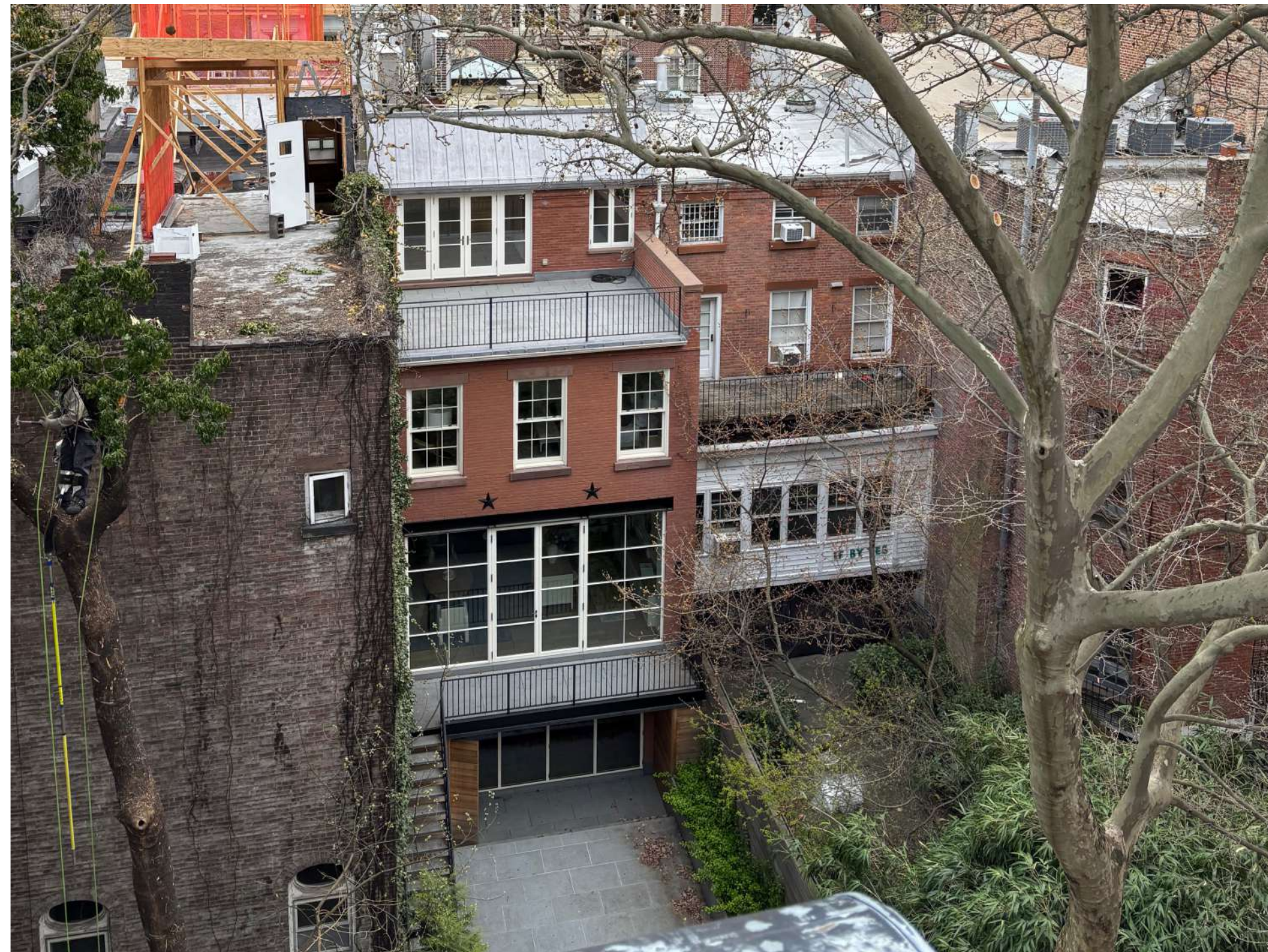
C) 34 W11TH REAR YARD EXCAVATION & ATTIC EXTENSION APPROVED 2/21/18
