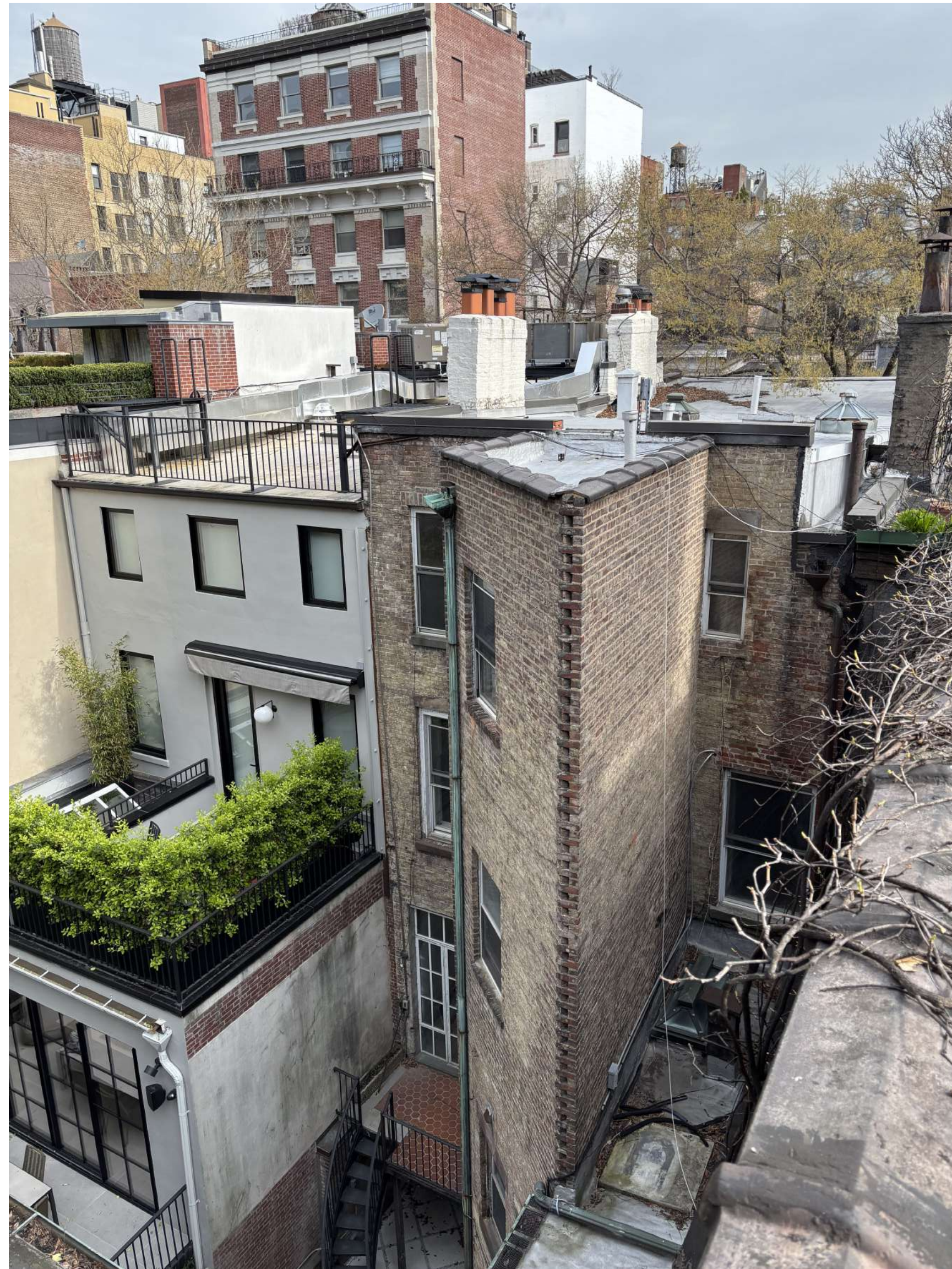
B - EXISTING REAR ROOFLINE LOOKING NORTH
