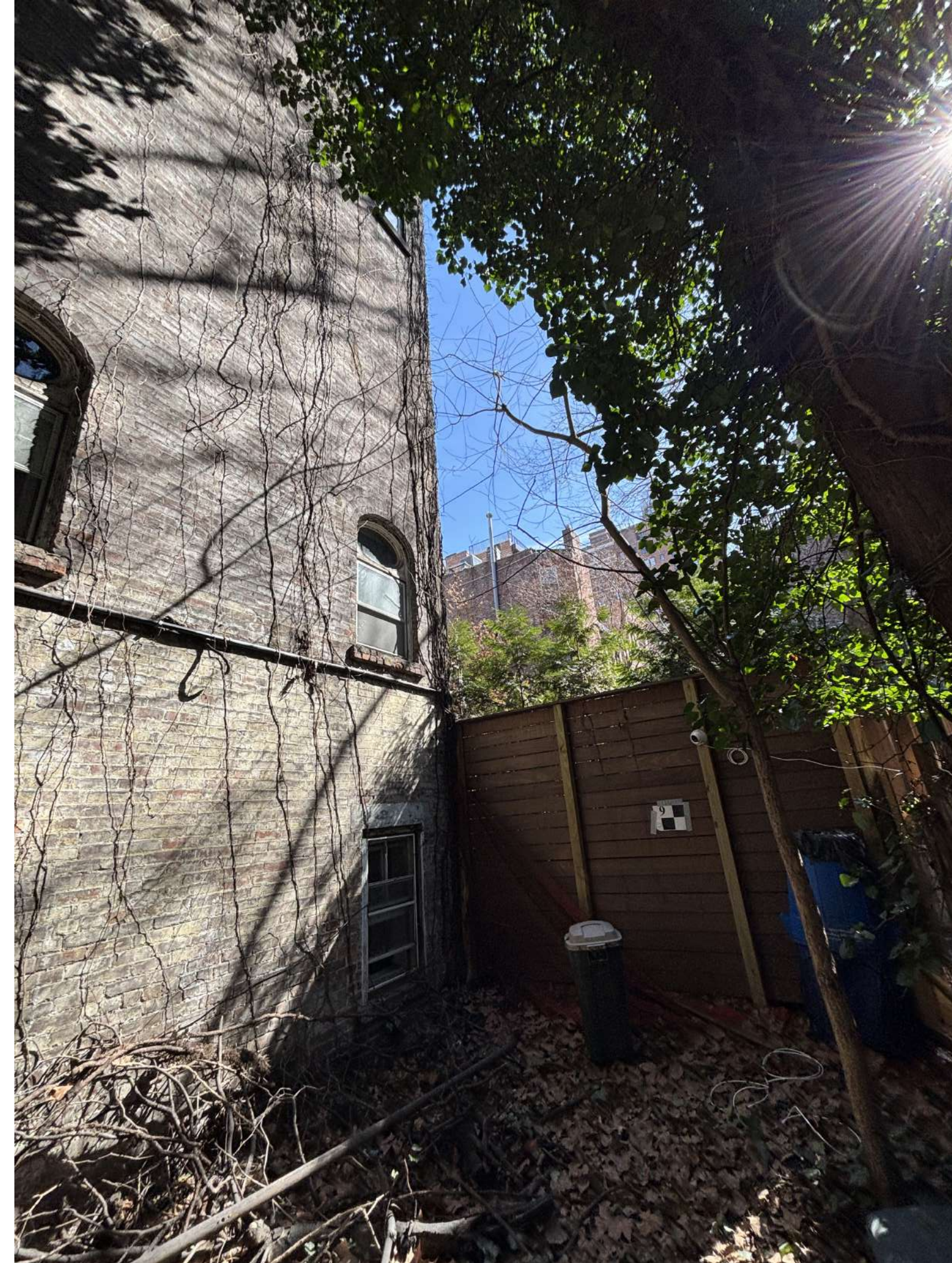
EXISTING 12'-5" REAR YARD LOOKING EAST
