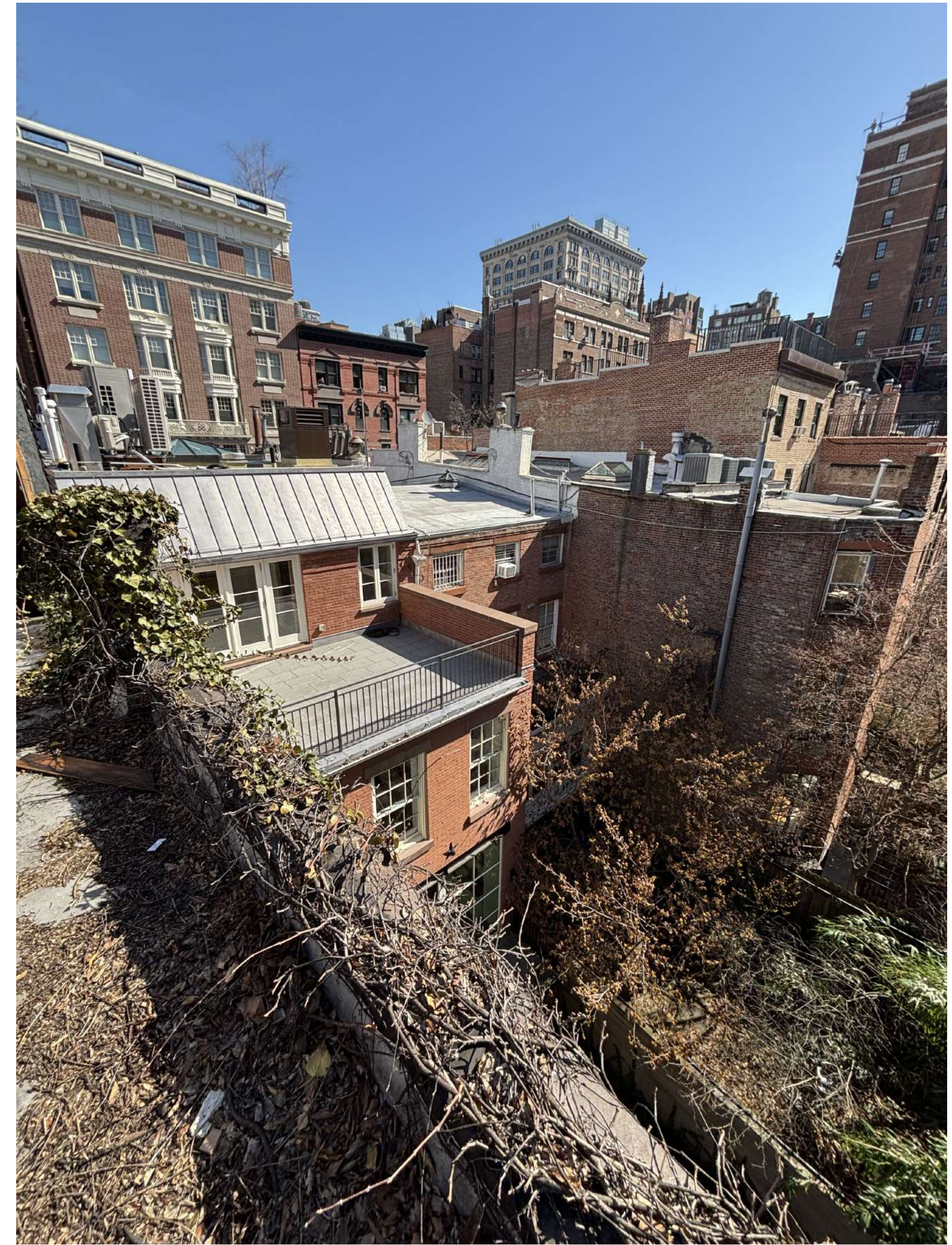
C - EXISTING REAR ROOFLINE LOOKING NORTH WEST
