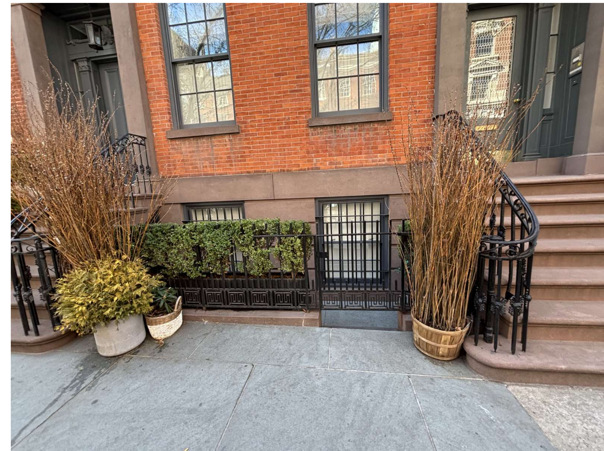
IRON & SIDEWALK RESTORATION - 42 W11TH
