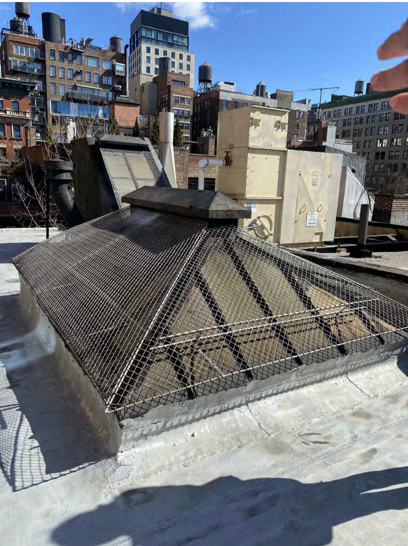
2 SITE PHOTOS: EXISTING SKYLIGHT NTS
