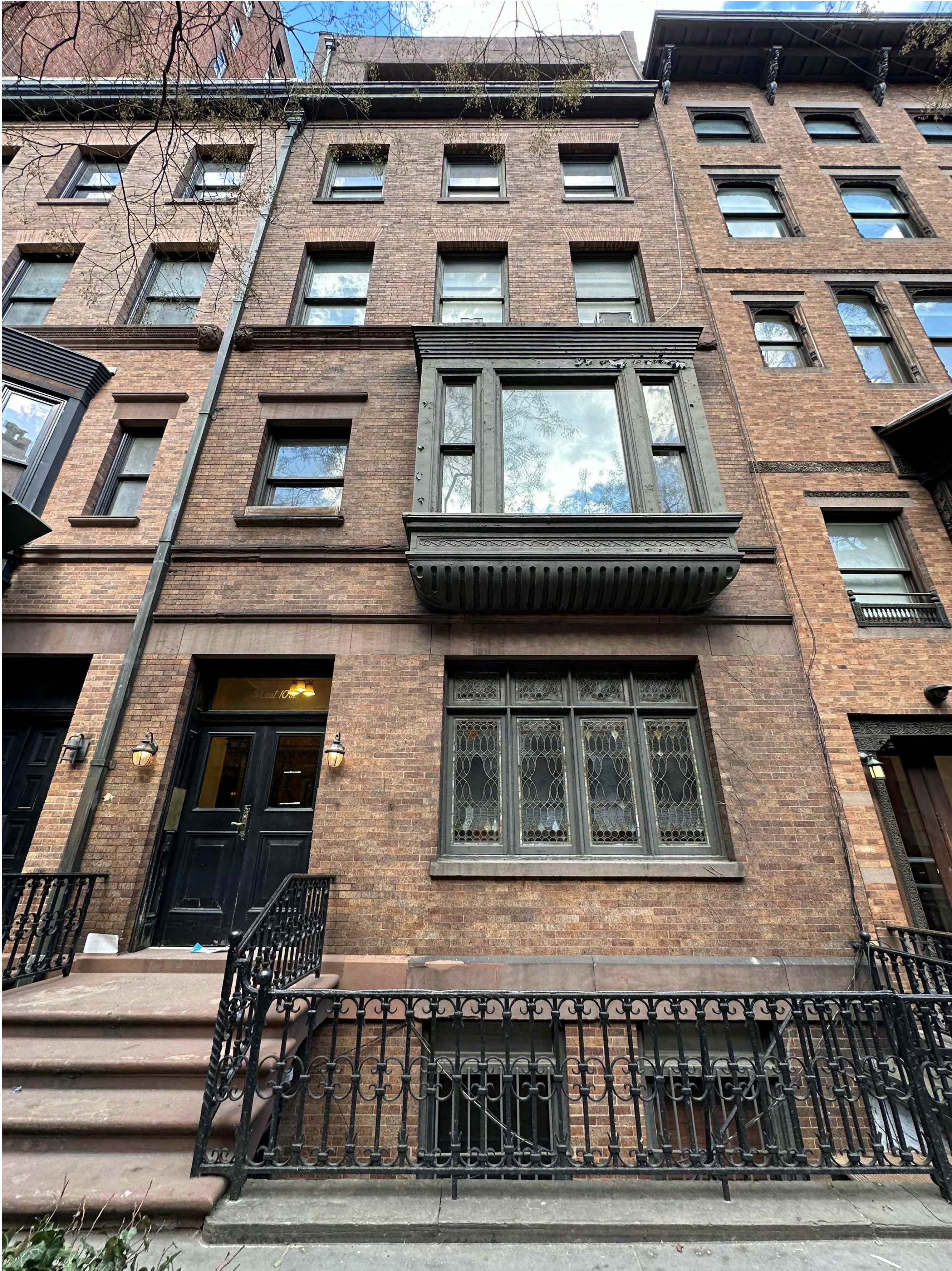
1 SITE PHOTO: EXISTING FRONT FACADE (SOUTH ELEVATION) NTS
