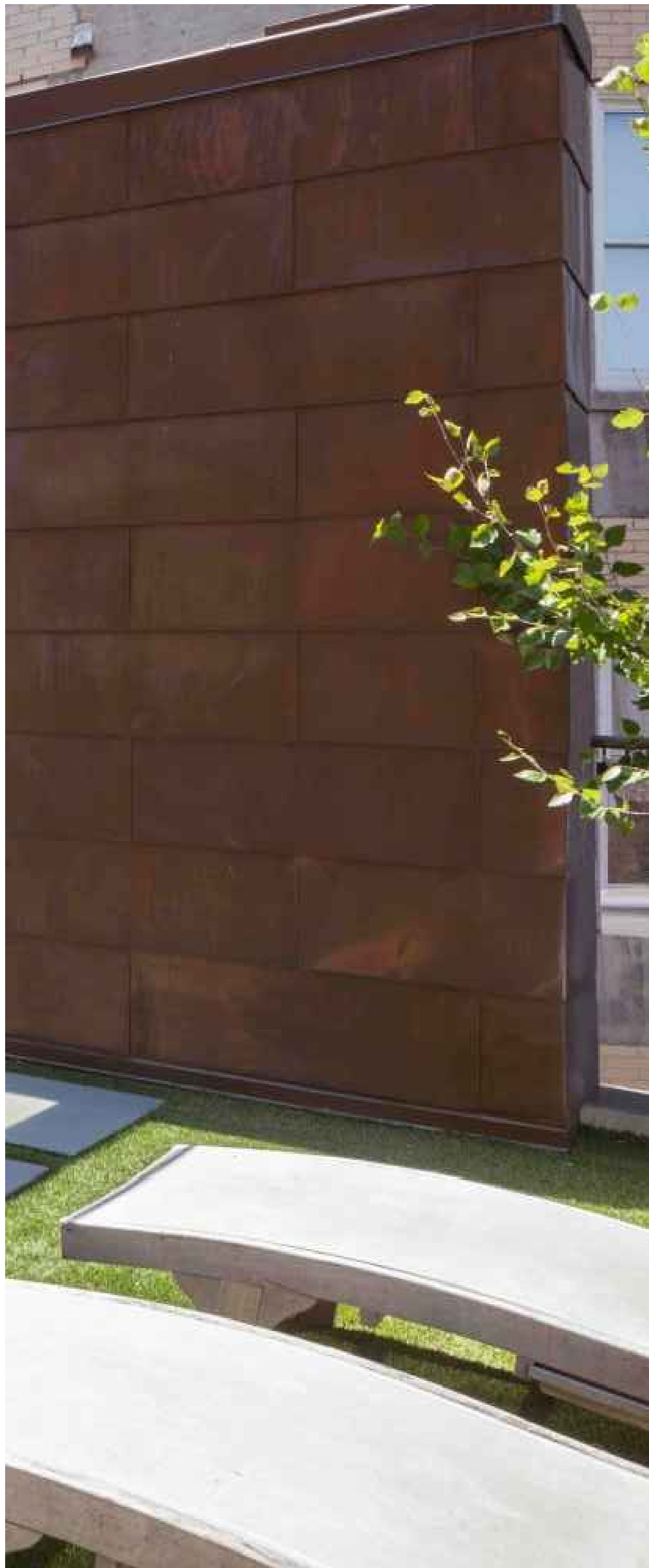
3 MATERIAL: COPPER PANEL CLADDING NTS
