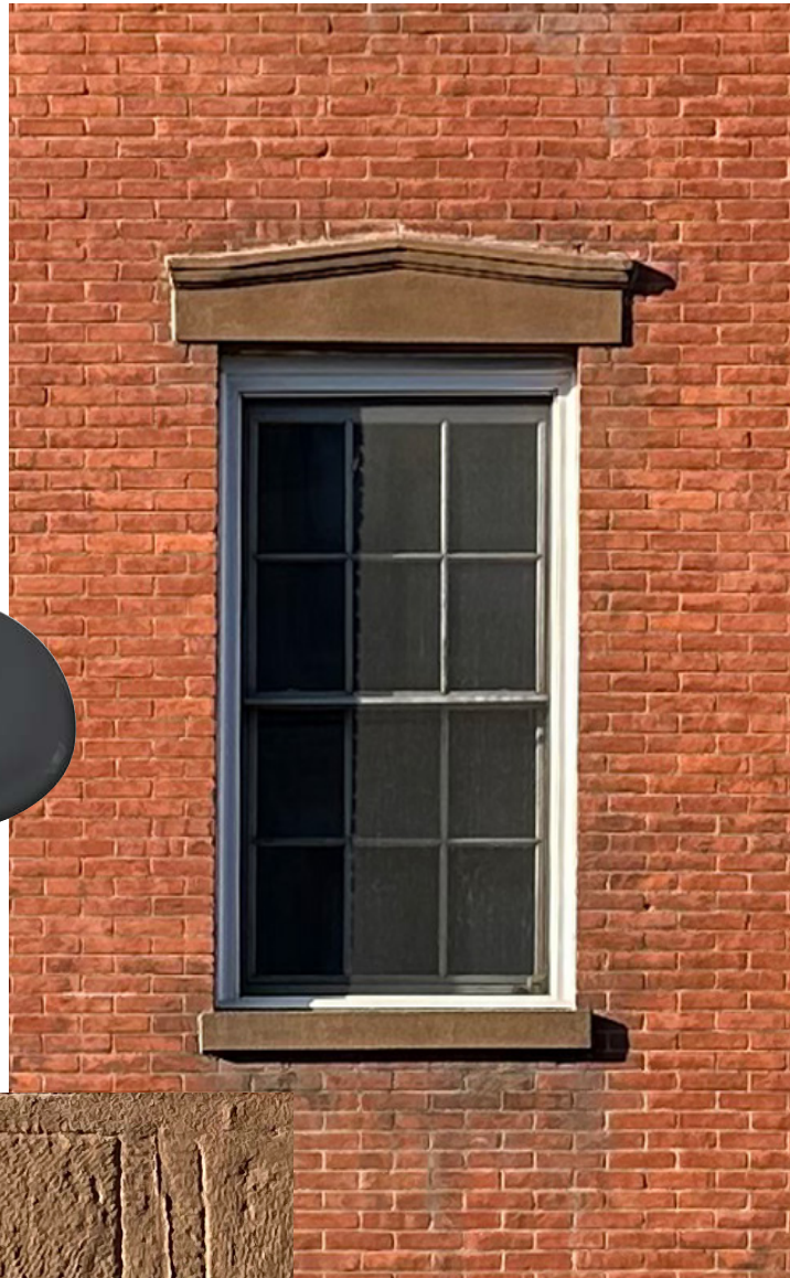
restore existing brick
