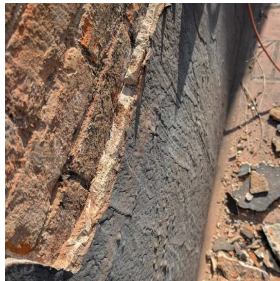
removal in progress
