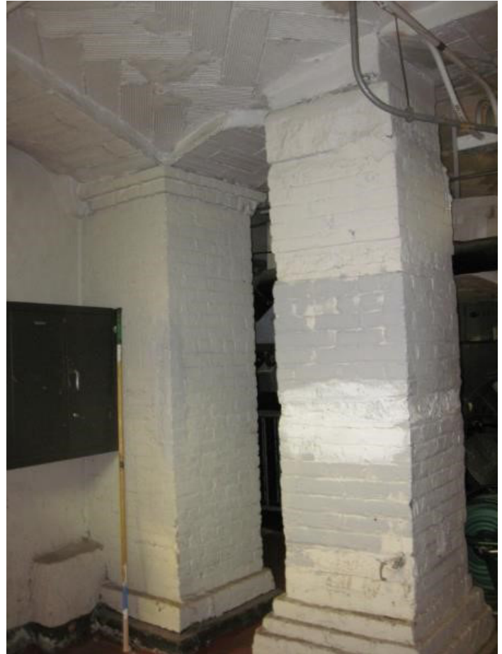
Basement Guastavino Arch Construction
