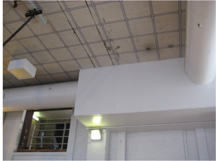
Gym #2 - Connection to Mezzanine Level
