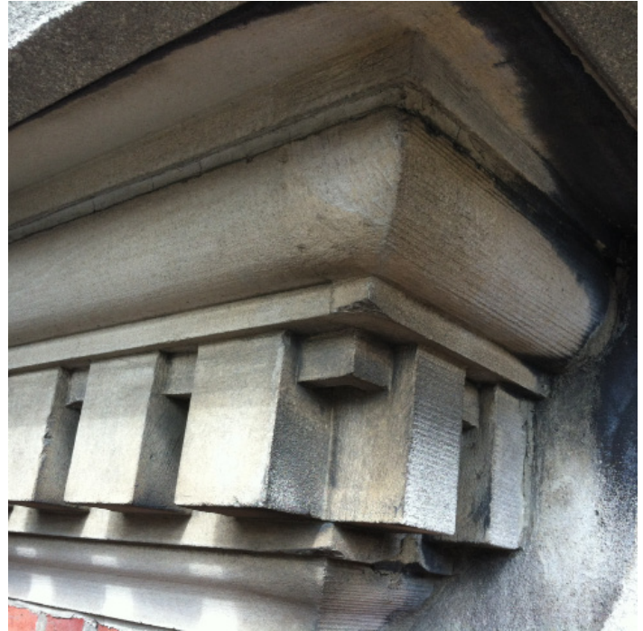
Limestone Dentil Molding at Cornice (Temp Safety Net Removal)
