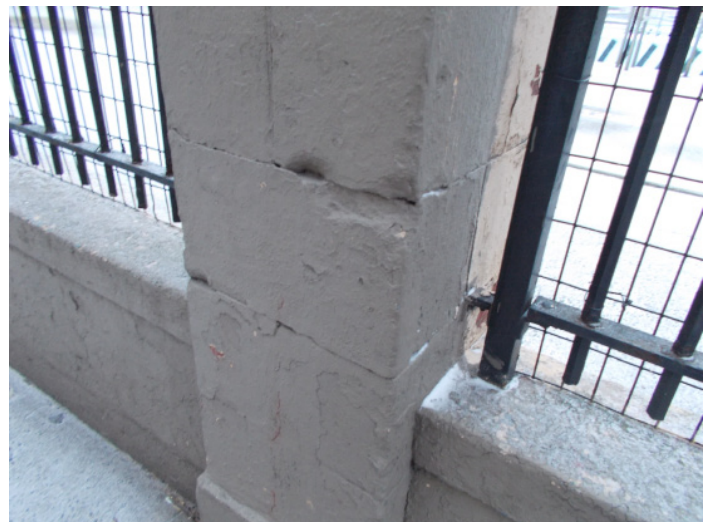
Clarkson Street - Pier at Barrier Wall
