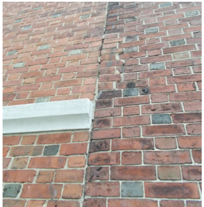
Mortared Joint between 1908 and 1929 Construction
