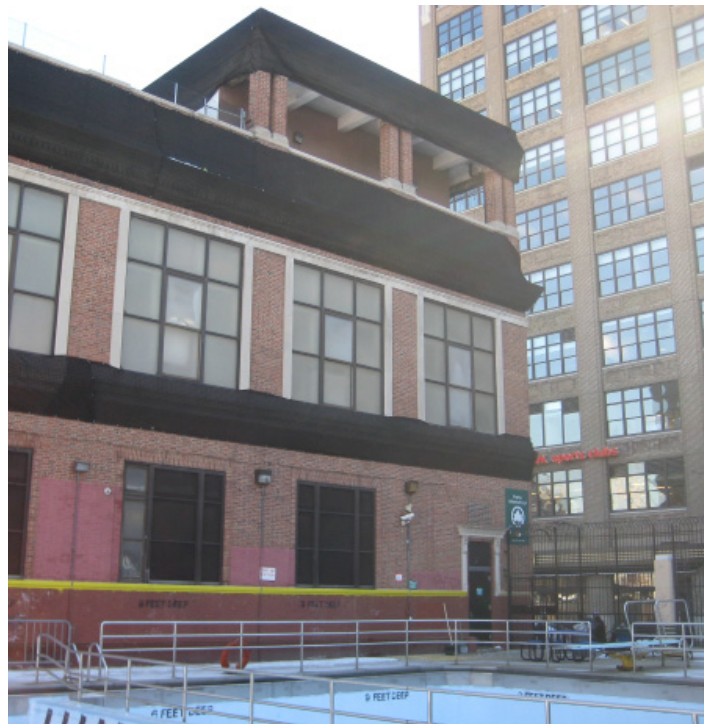
Colonnade / Mechanical Bulkhead
