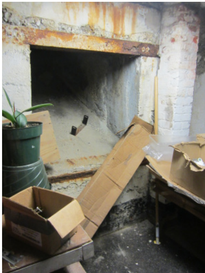
Coal Chute Opening in Basement
