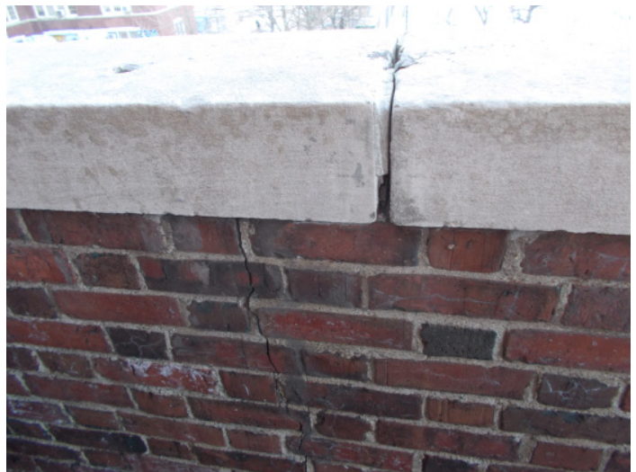
Priority 2 - Parapet and Coping Repair
