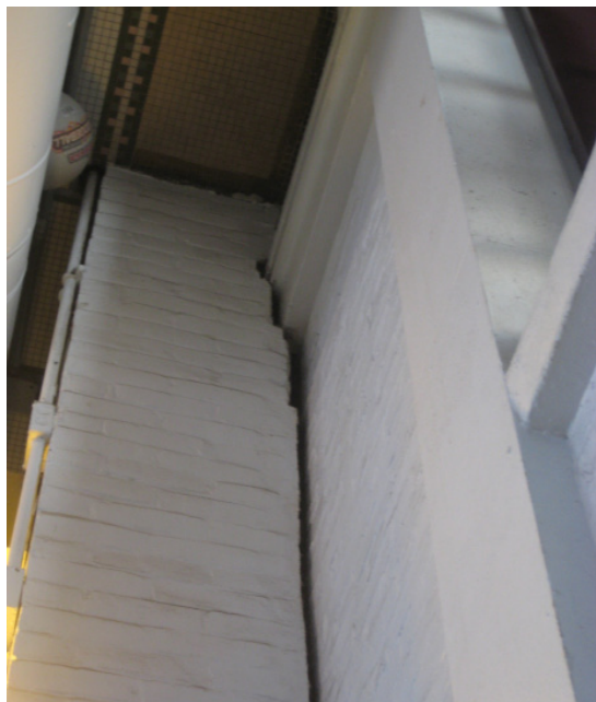
Expansion Separation between 1908 and 1929 Constructions
