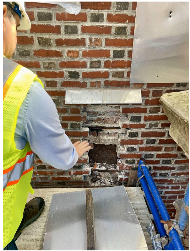
Damaged historic brickwork at exterior of Recreation Center Both photographs by Village Preservation staff, April 23, 2025
