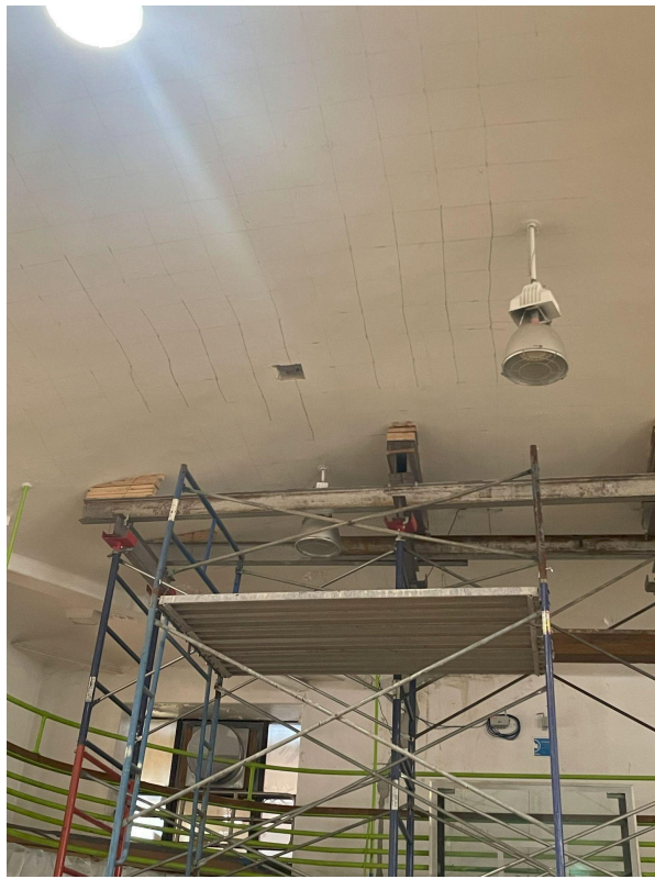
Temporary structural bracing in place at the interior
