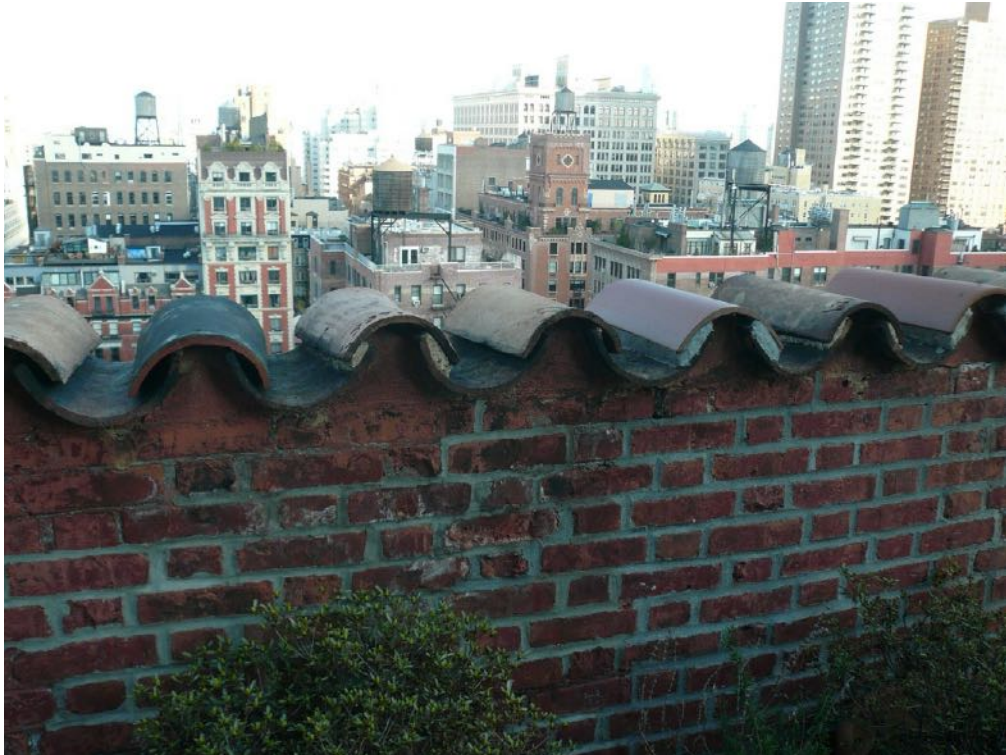
DETAIL VIEW OF EXISTING PARAPET WALL
