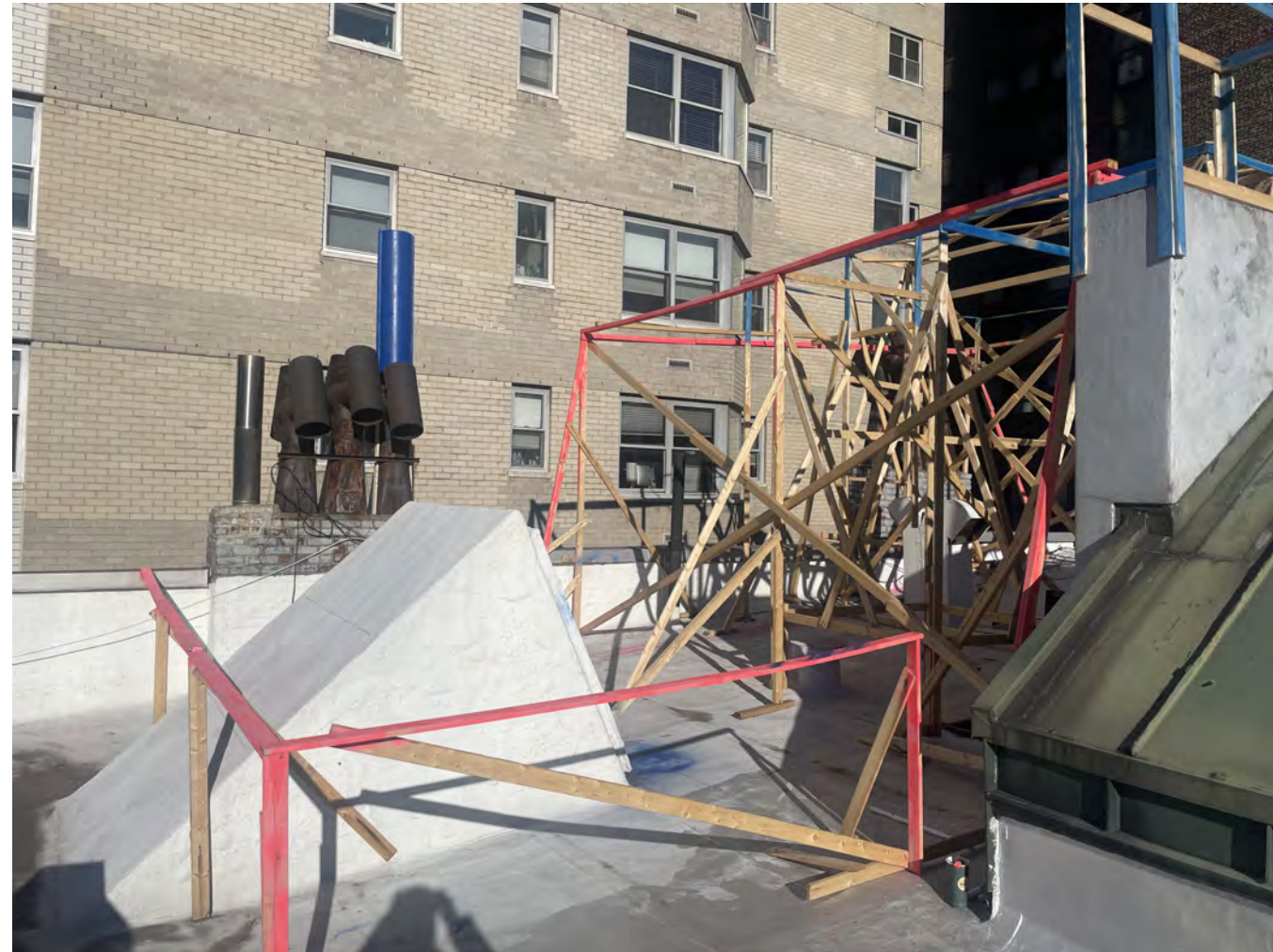
LOOKING NORTHEAST FROM ROOFTOP ADDITION MOCKUP
