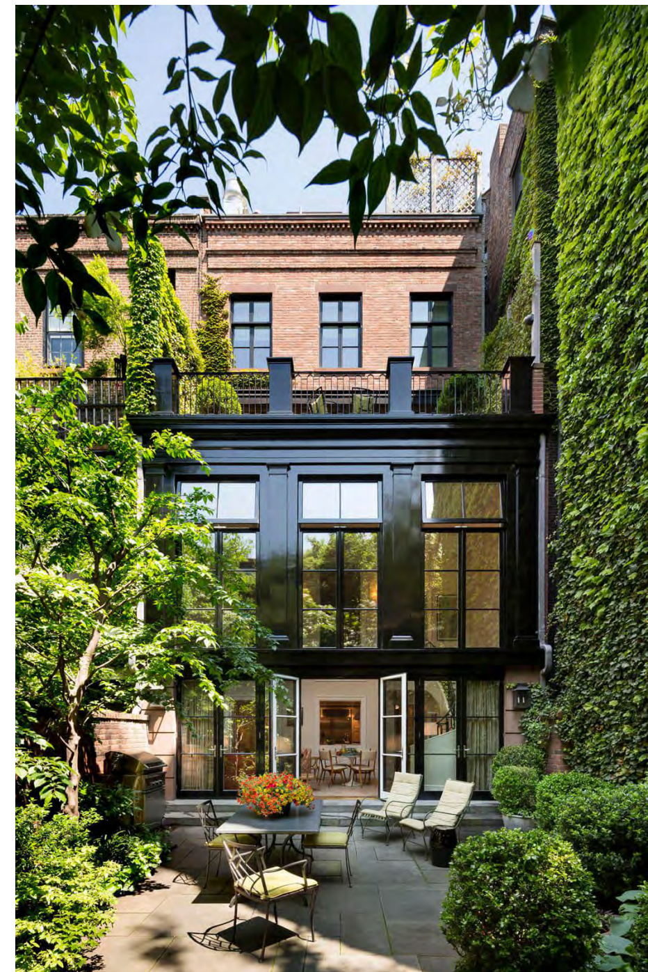
58 MORTON STREET RECONSTRUCTED TEA PORCH
