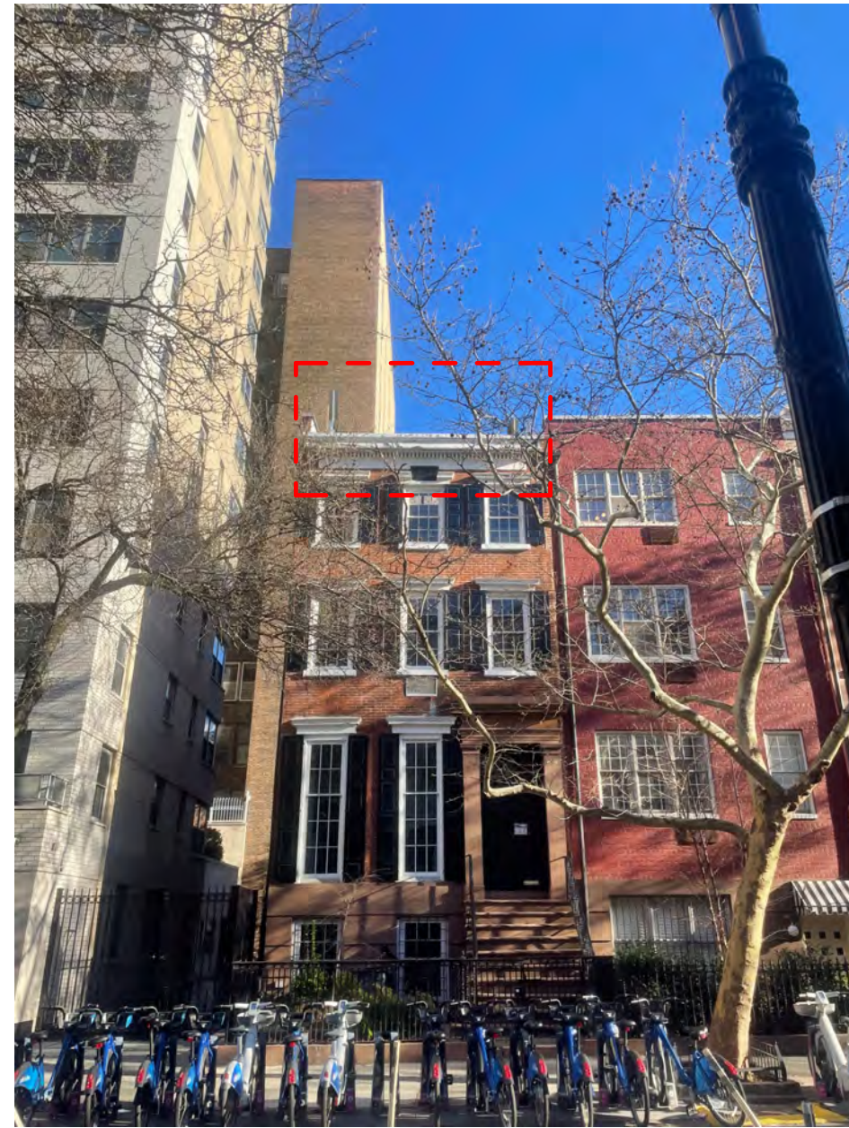
RENDERED ADDITION (FLUE EXTENSIONS) VIEWED FROM SOUTH SIDE 13TH STREET
