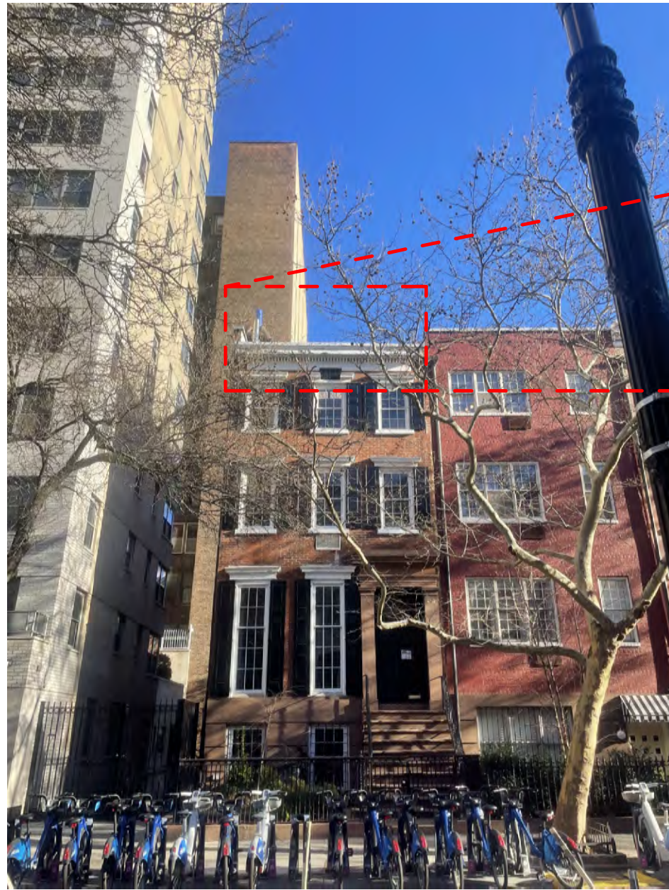
MOCKUP ADDITION (FLUE EXTENSIONS) VIEWED FROM SOUTH SIDE 13TH STREET
