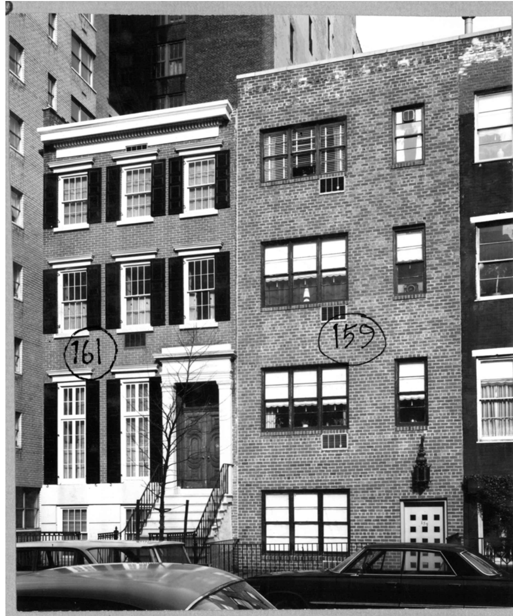
1968 LPC DESIGNATION PHOTO
