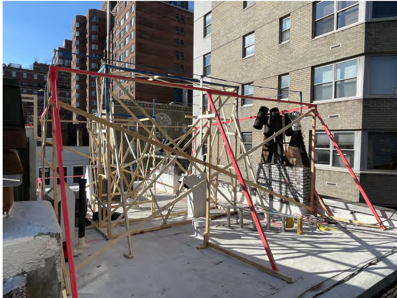
LOOKING SOUTH FROM ROOFTOP ADDITION MOCKUP
