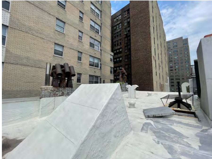
LOOKING NORTHWEST FROM EXISTING SKYLIGHT
