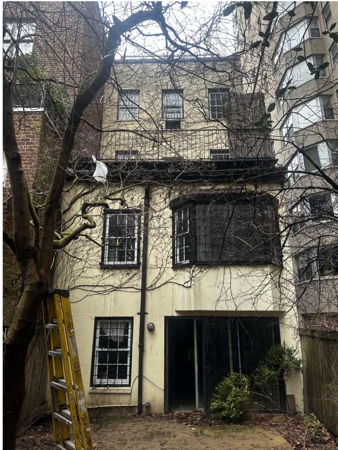
REAR FACADE; BASEMENT LEVEL THROUGH LEVEL 3
