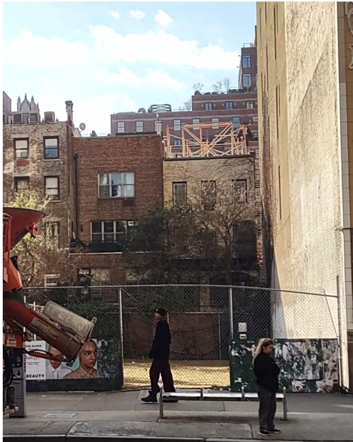
EXISTING REAR VIEW FROM 14TH STREET
