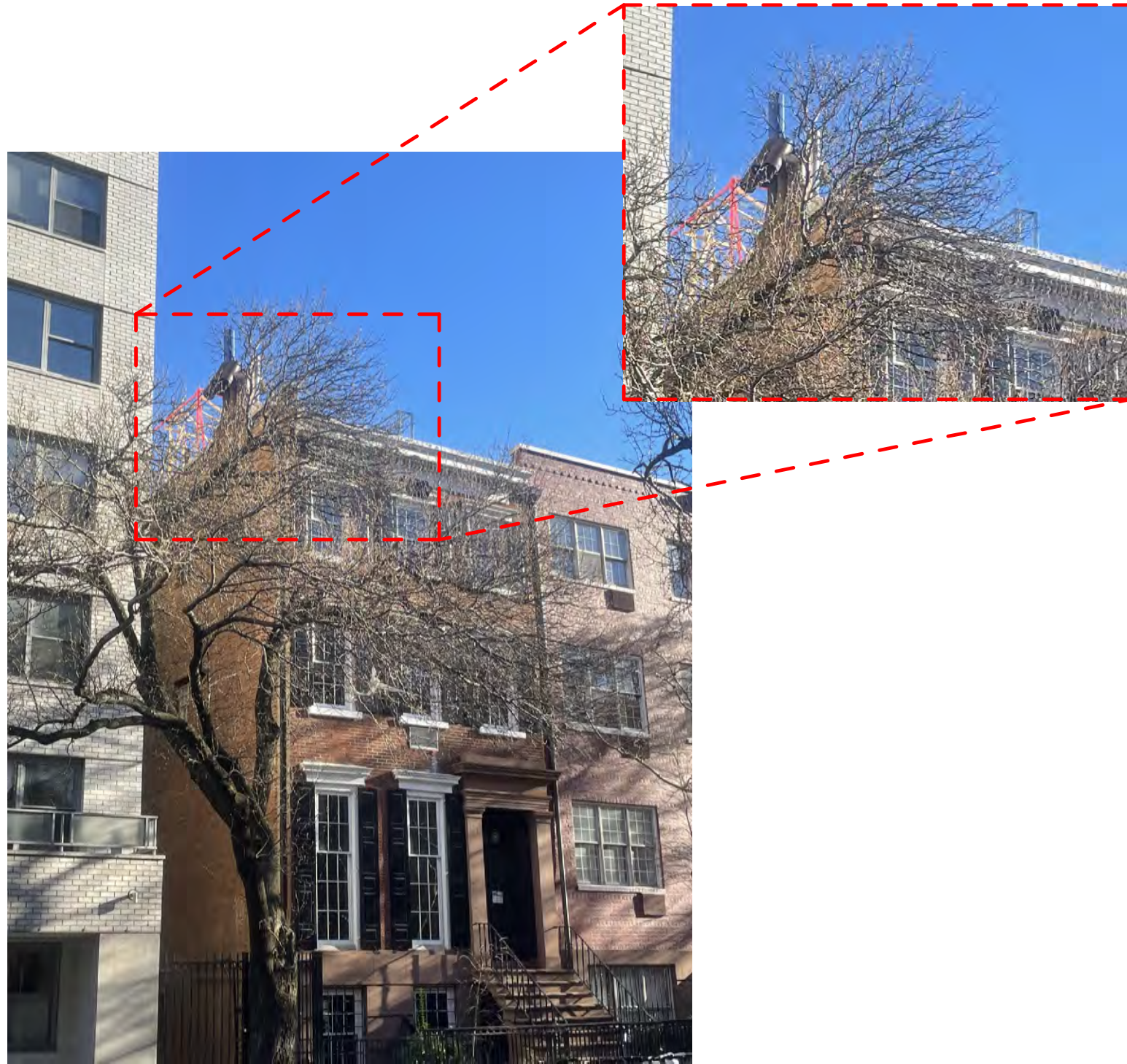
MOCKUP ADDITION VIEWED FROM SOUTHWEST SIDE 13TH STREET
