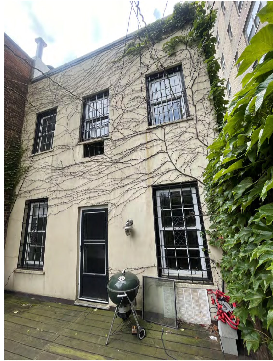
LEVEL 2 AND LEVEL 3 - REAR FACADE CLOSE-UP VIEW
