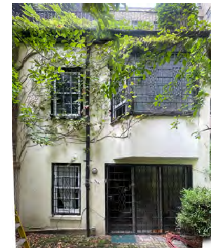
EXISTING REAR VIEW (FROM REAR GRADE)
