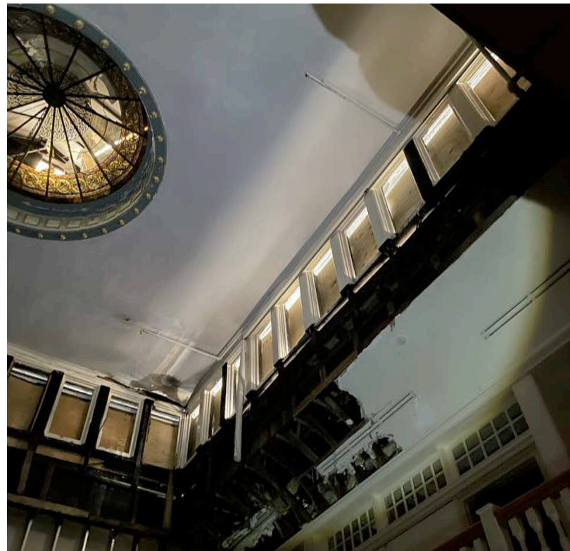
INTERIOR / EXISTING CLERESTORY WINDOWS
