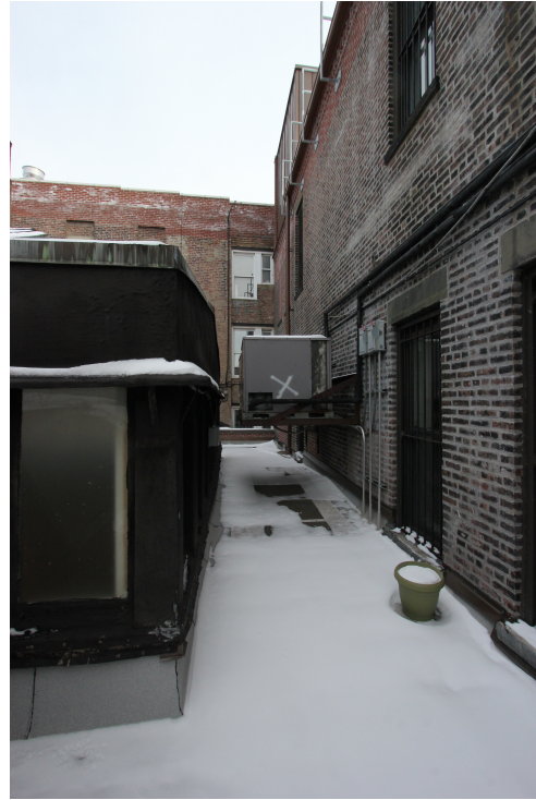
OVERVIEW OF 3RD FLOOR ROOF / EXTERIOR CIRCA 2017
