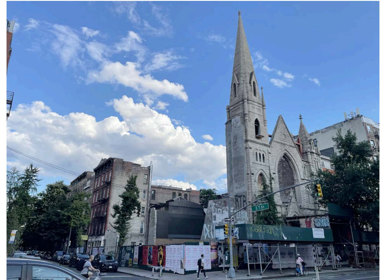
OVERVIEW OF EXISTING BUILDING.
