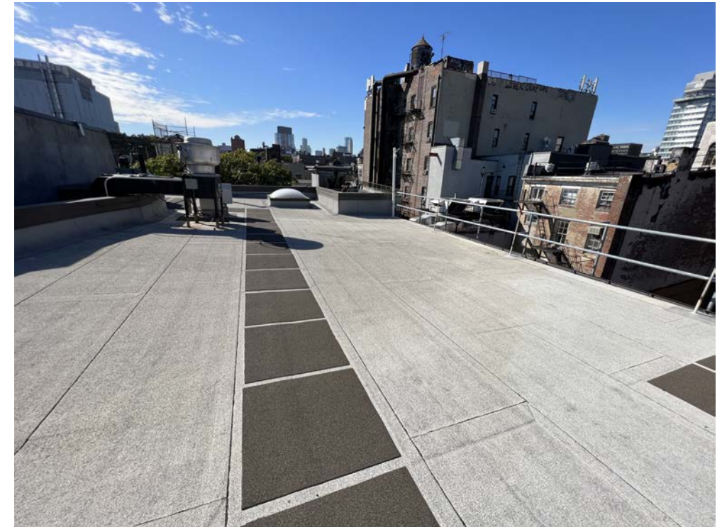
OVERVIEW OF 5TH FLOOR ROOF
