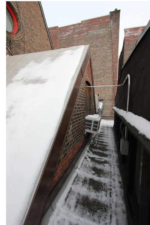
OVERVIEW OF 3RD FLOOR ROOF / EXTERIOR CIRCA 2017
