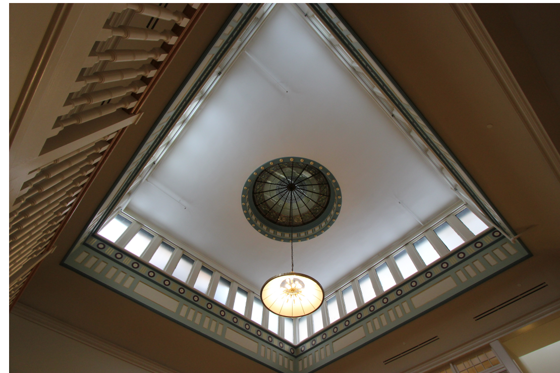
OVERVIEW CLERESTORY / INTERIOR CIRCA 2017
