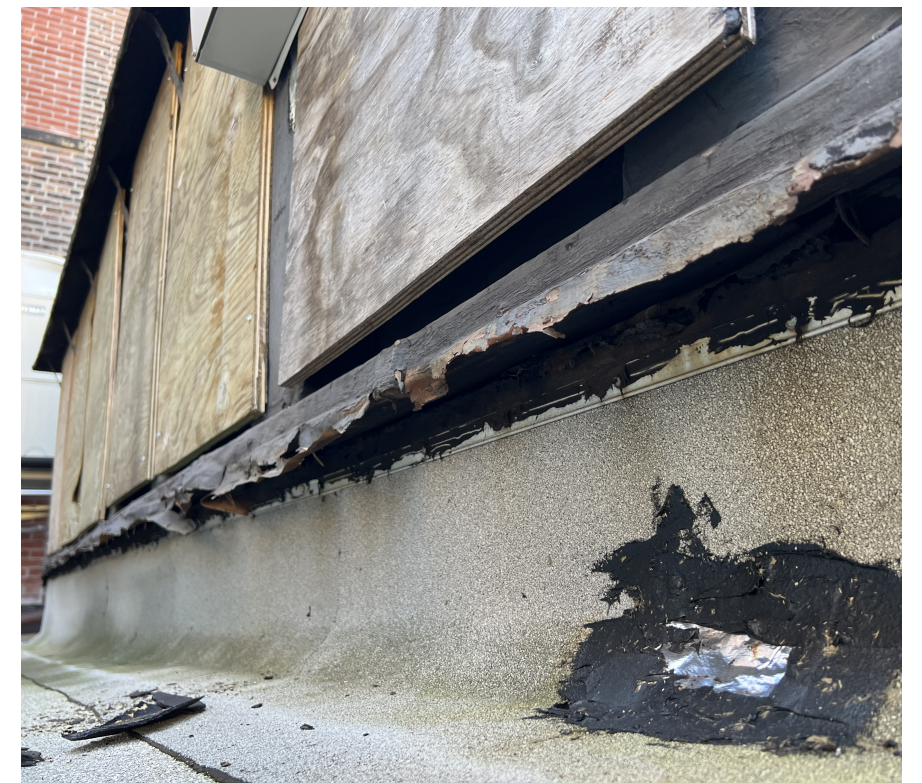
EXISTING EXTERIOR CLERESTORY WINDOWS SIDING
