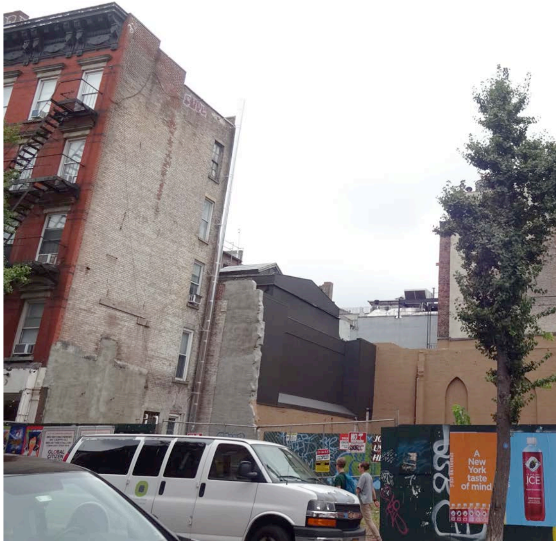
OVERVIEW OF WEST ELEVATION
