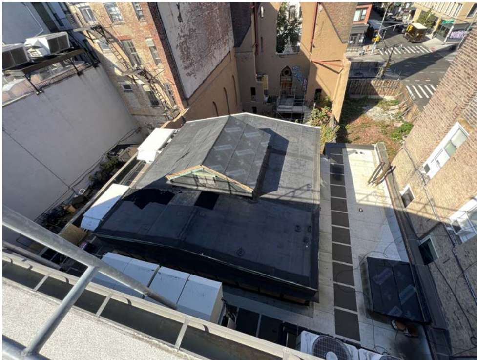
VIEW OF 3RD FLOOR / ROOF BELOW
