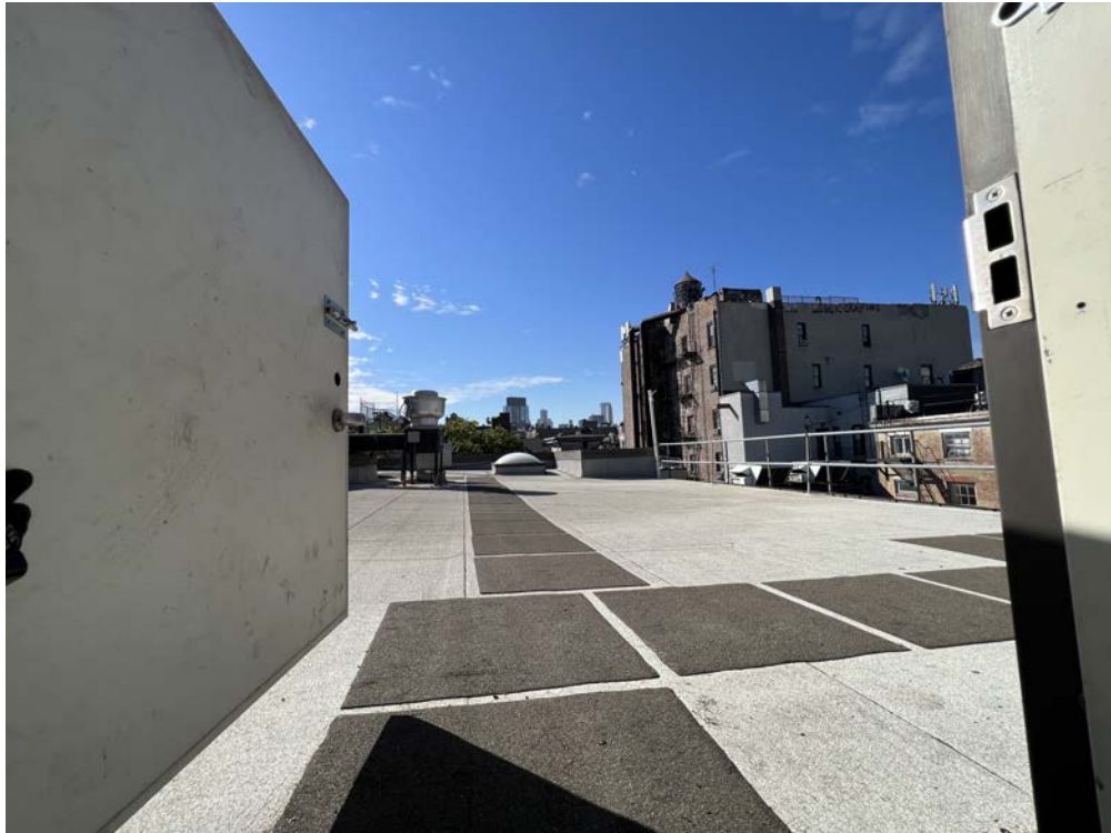
OVERVIEW OF 5TH FLOOR ROOF
