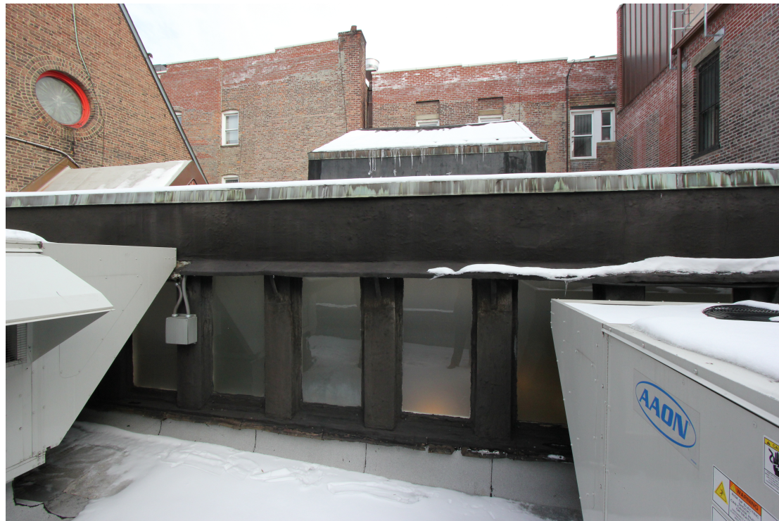
OVERVIEW OF 3RD FLOOR ROOF / EXTERIOR CIRCA 2017
