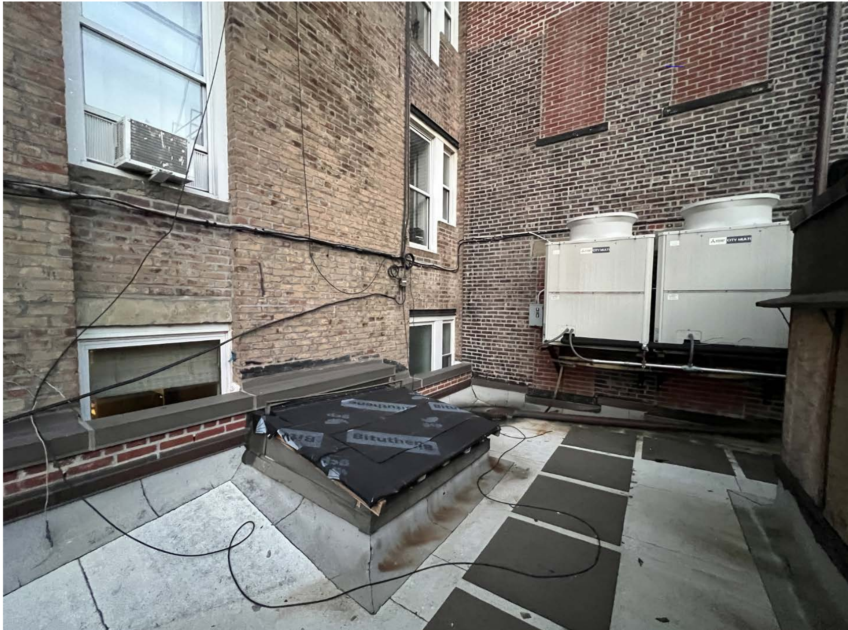
OVERVIEW OF EXISTING SKYLIGHT
