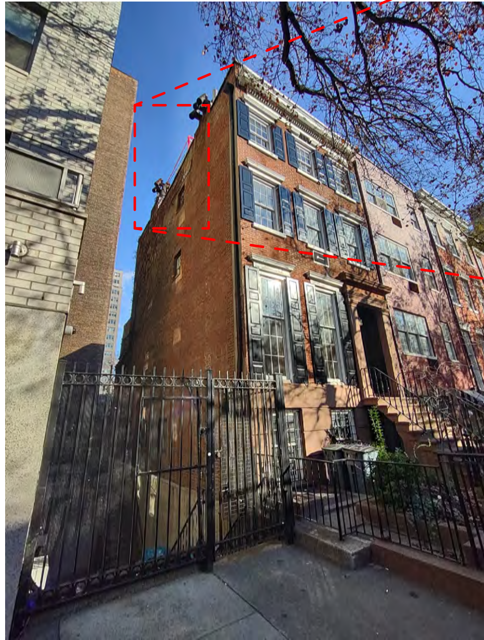
MOCKUP ADDITION VIEWED FROM NORTH SIDE 13TH STREET
