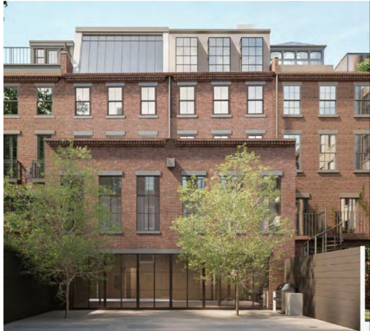
79-81 CHARLES STREET STUDIO WINDOW ADDITION APPROVED IN 2022
