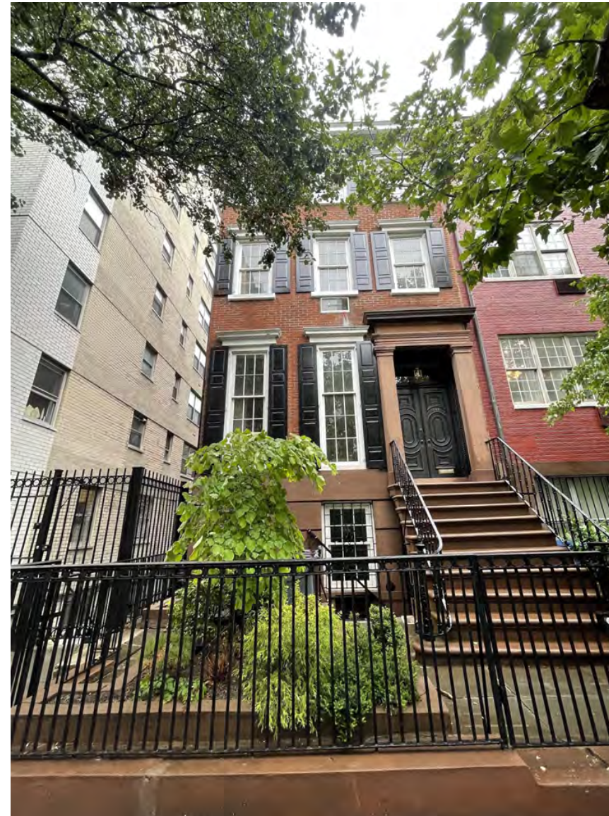
EXISTING FRONT VIEW
