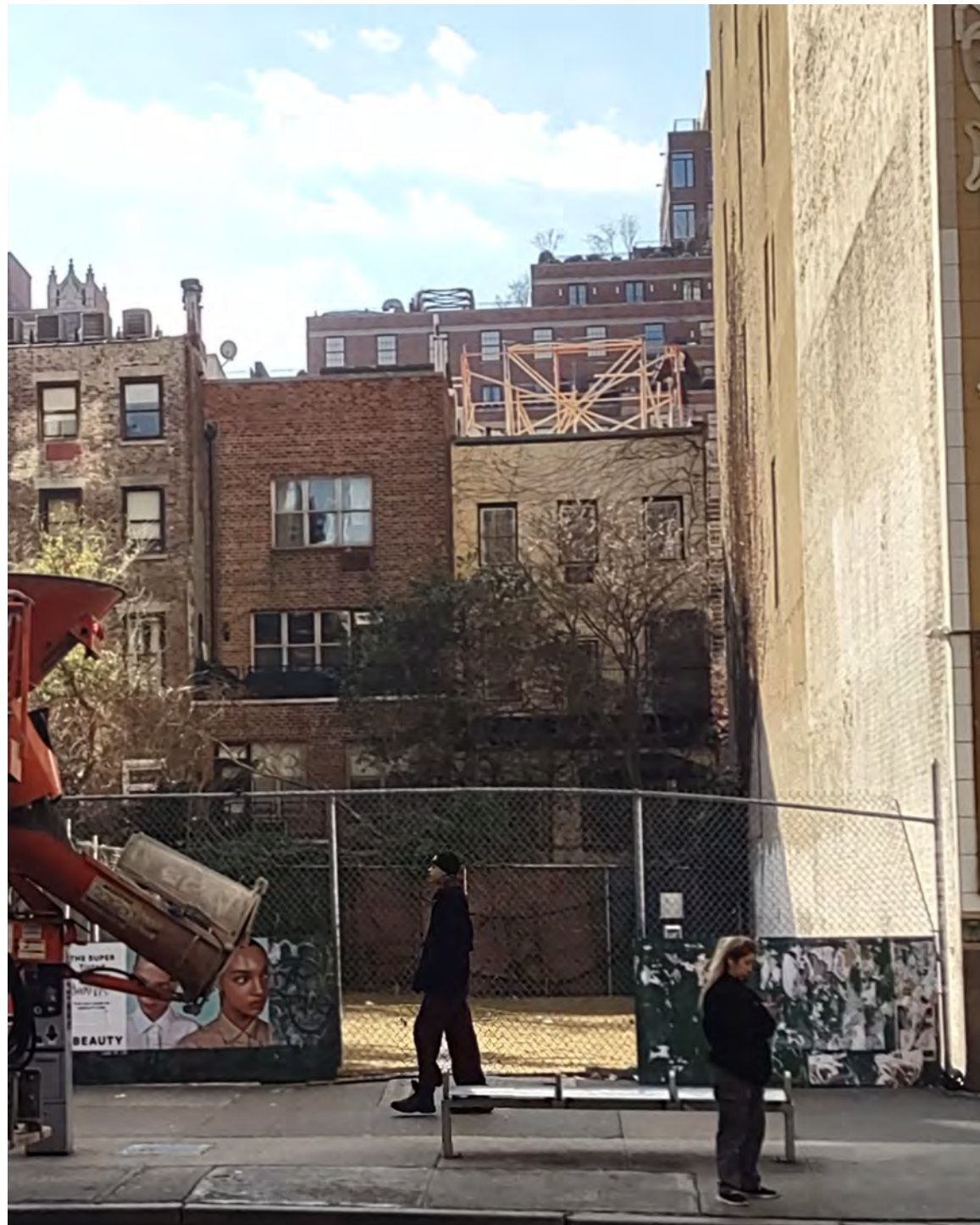
EXISTING REAR VIEW FROM 14TH STREET
