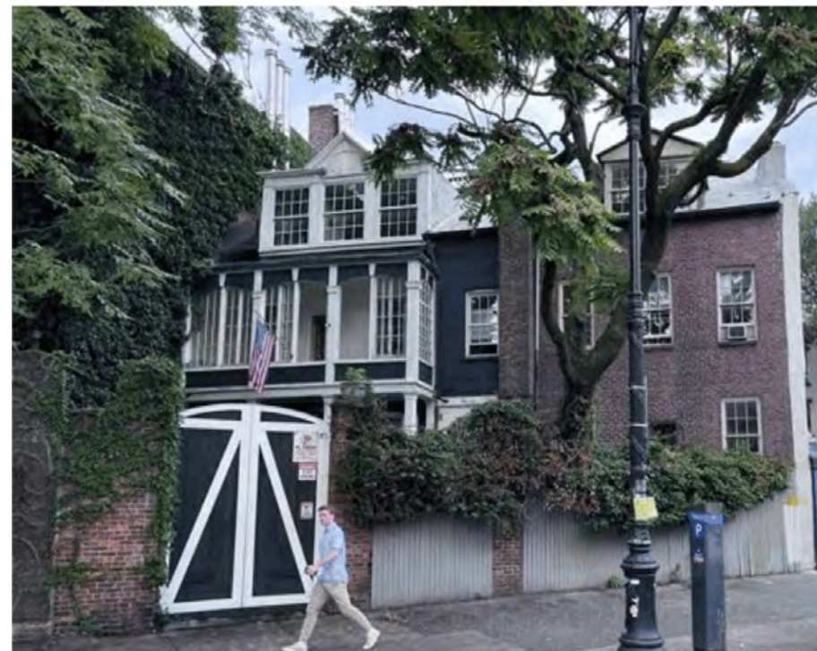
18 COMMERCE STREET REAR TEA PORCH IN 1914 (ABOVE) AND IN 2023 (BELOW) WITH 1920 COLONIAL REVIVAL ALTERATION
