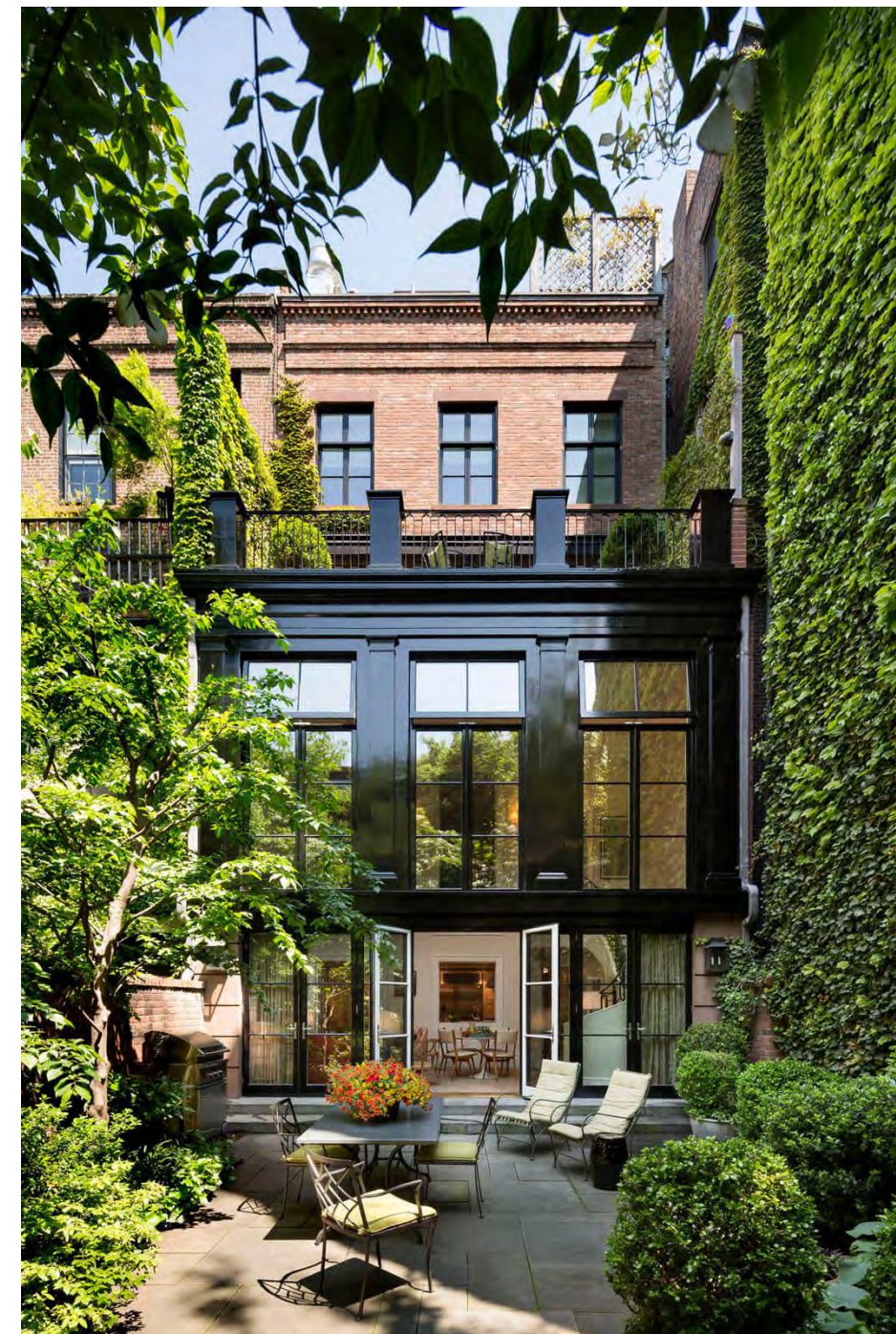
58 MORTON STREET RECONSTRUCTED TEA PORCH
