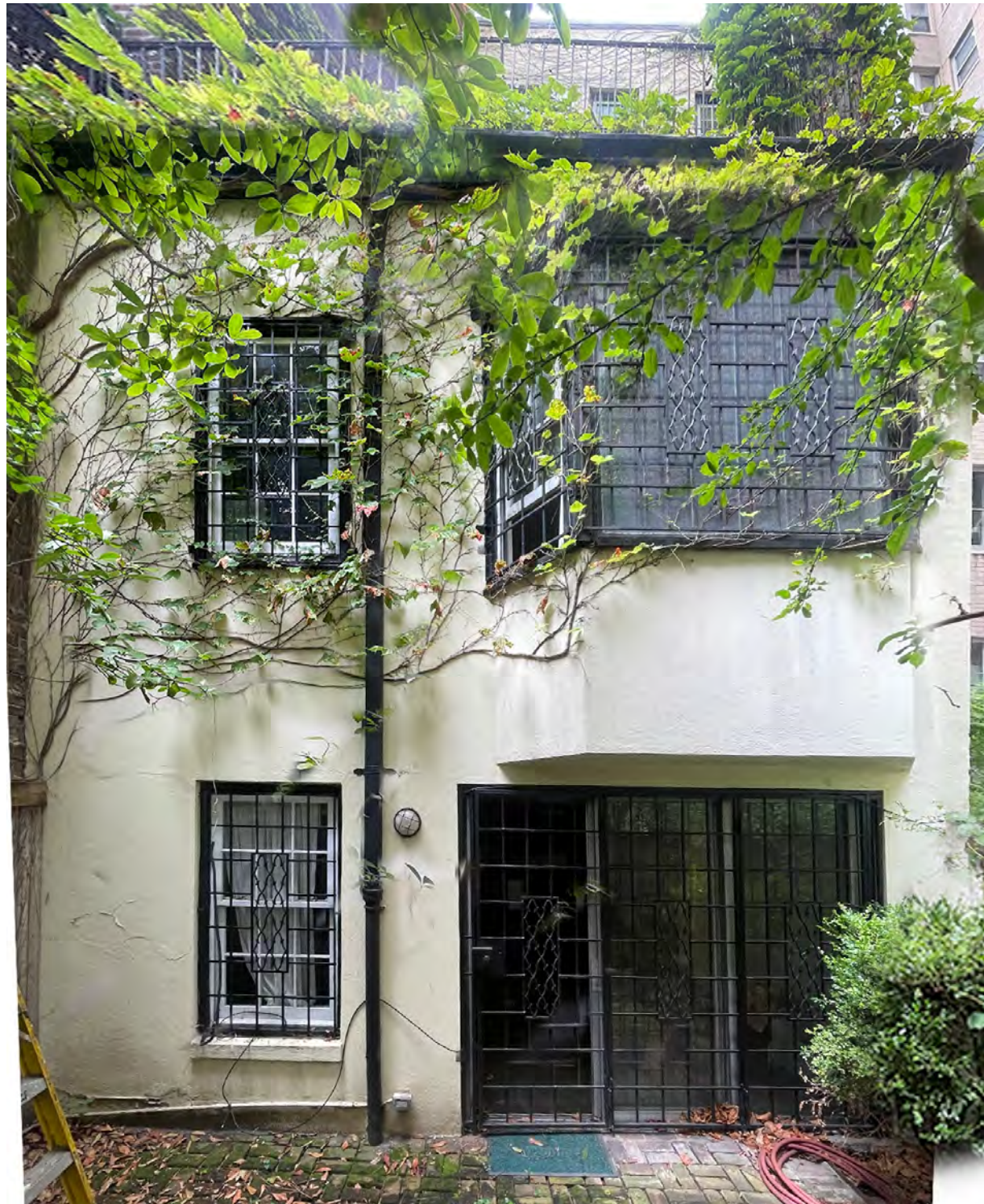
BASEMENT AND LEVEL 1 - REAR FACADE
