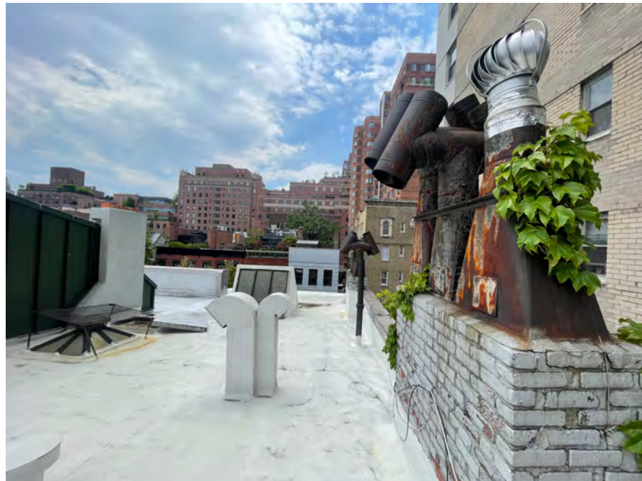
LOOKING SOUTHEAST FROM REAR OF ROOFTOP
