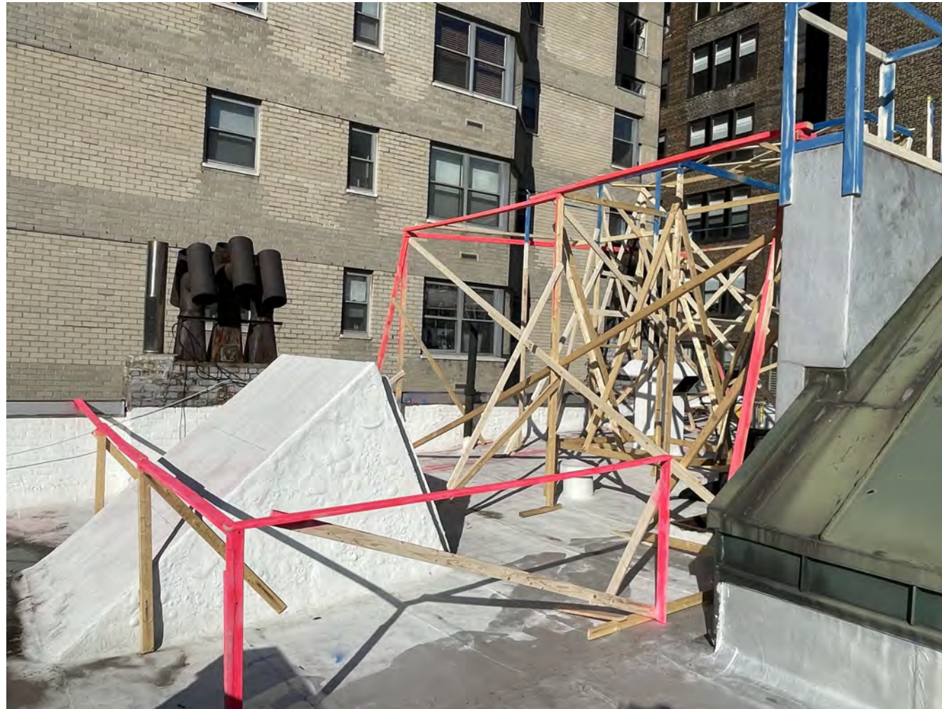
LOOKING NORTHEAST FROM ROOFTOP ADDITION MOCKUP
