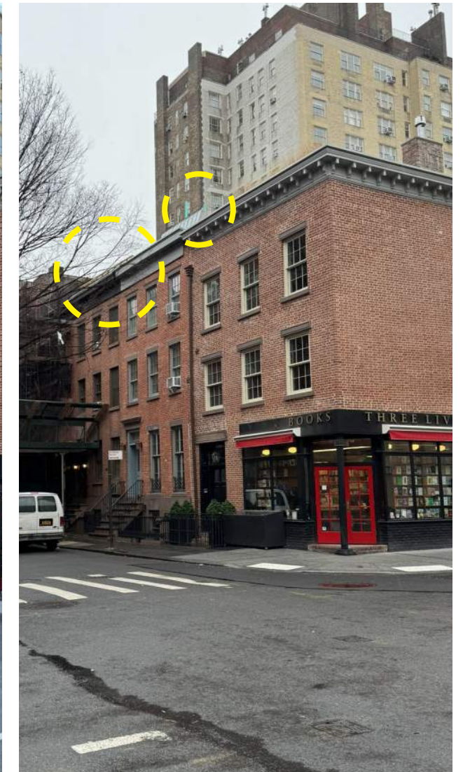
3c Railing seasonally visible through trees, Front Chimney flues partly visible outside of trees
