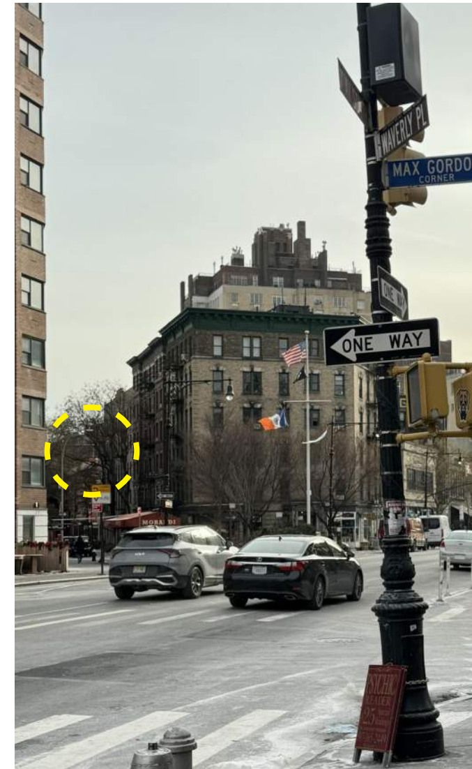
4d Front chimney and flues and railing are seasonally visible through trees
