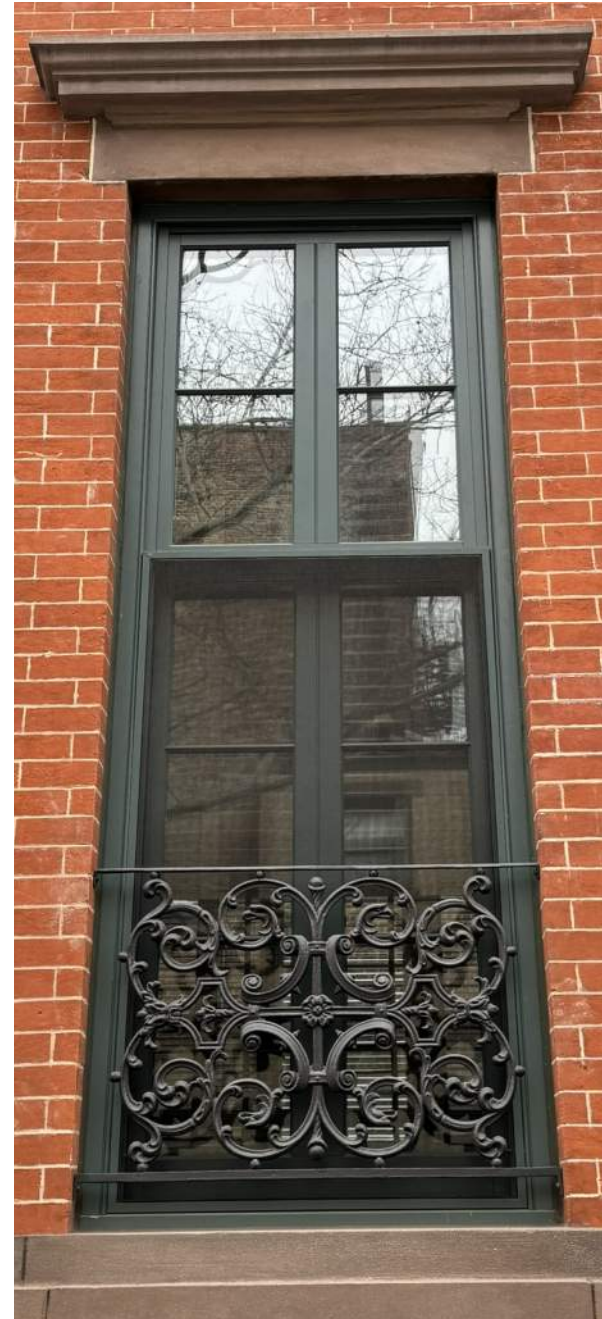
CURRENT 156 AND 158 W. 10TH ST WINDOWS
