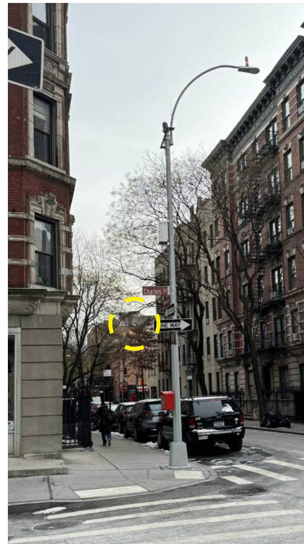
4b Front chimney and flues and railing are seasonally visible through trees
