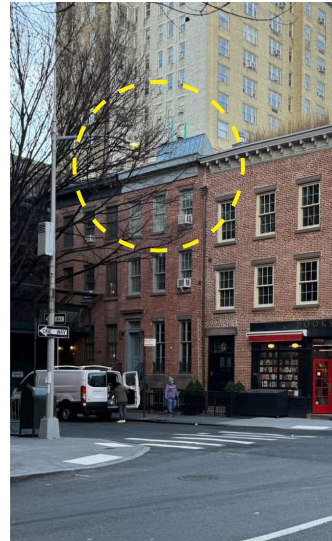
3b Railing and Front Chimney flues seasonally visible; a small portion of the mechanical screen is visible outside of trees
