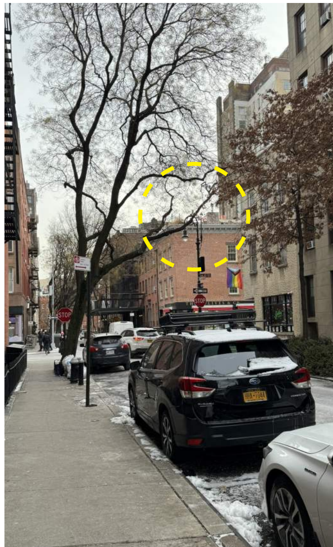
4a Mechanical screen and chimney flues seasonally visible through trees
