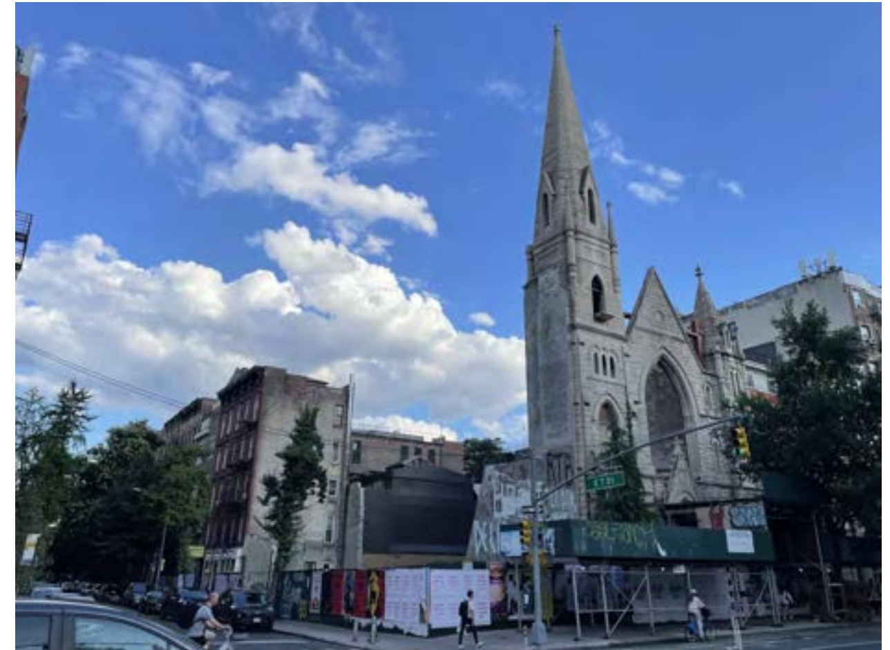
OVERVIEW OF EXISTING BUILDING.
