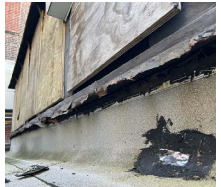
EXISTING EXTERIOR CLERESTORY WINDOWS SIDING
