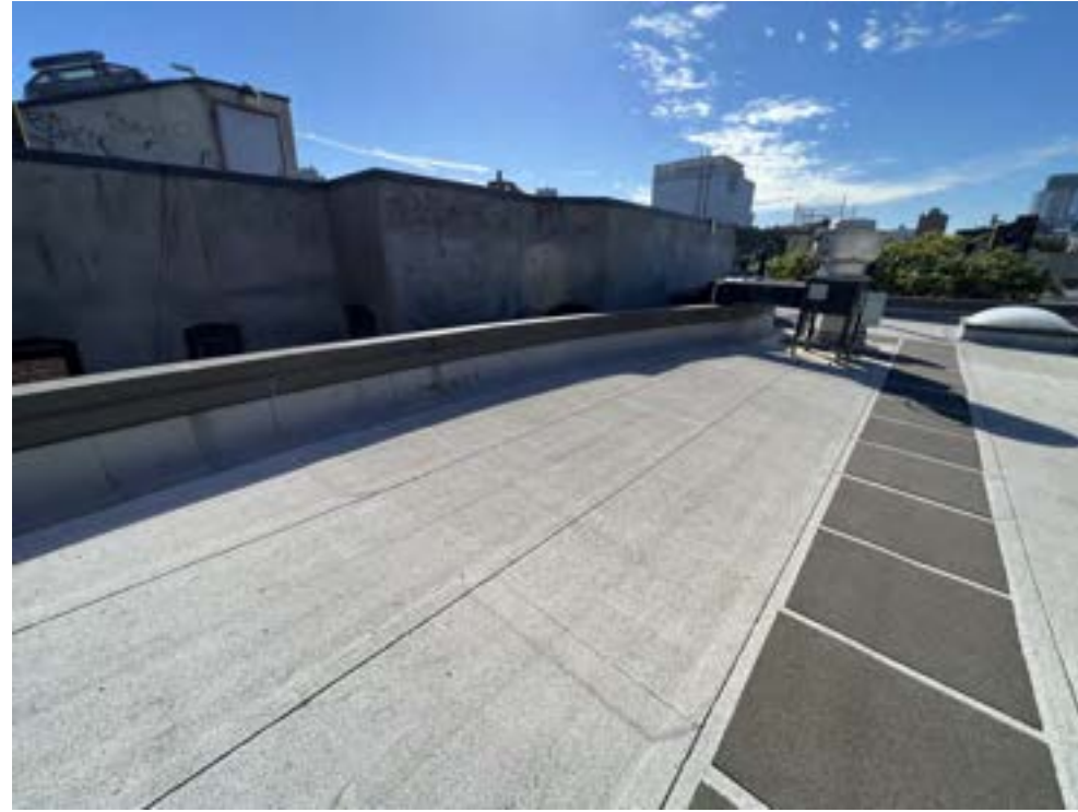
OVERVIEW OF 5TH FLOOR ROOF
