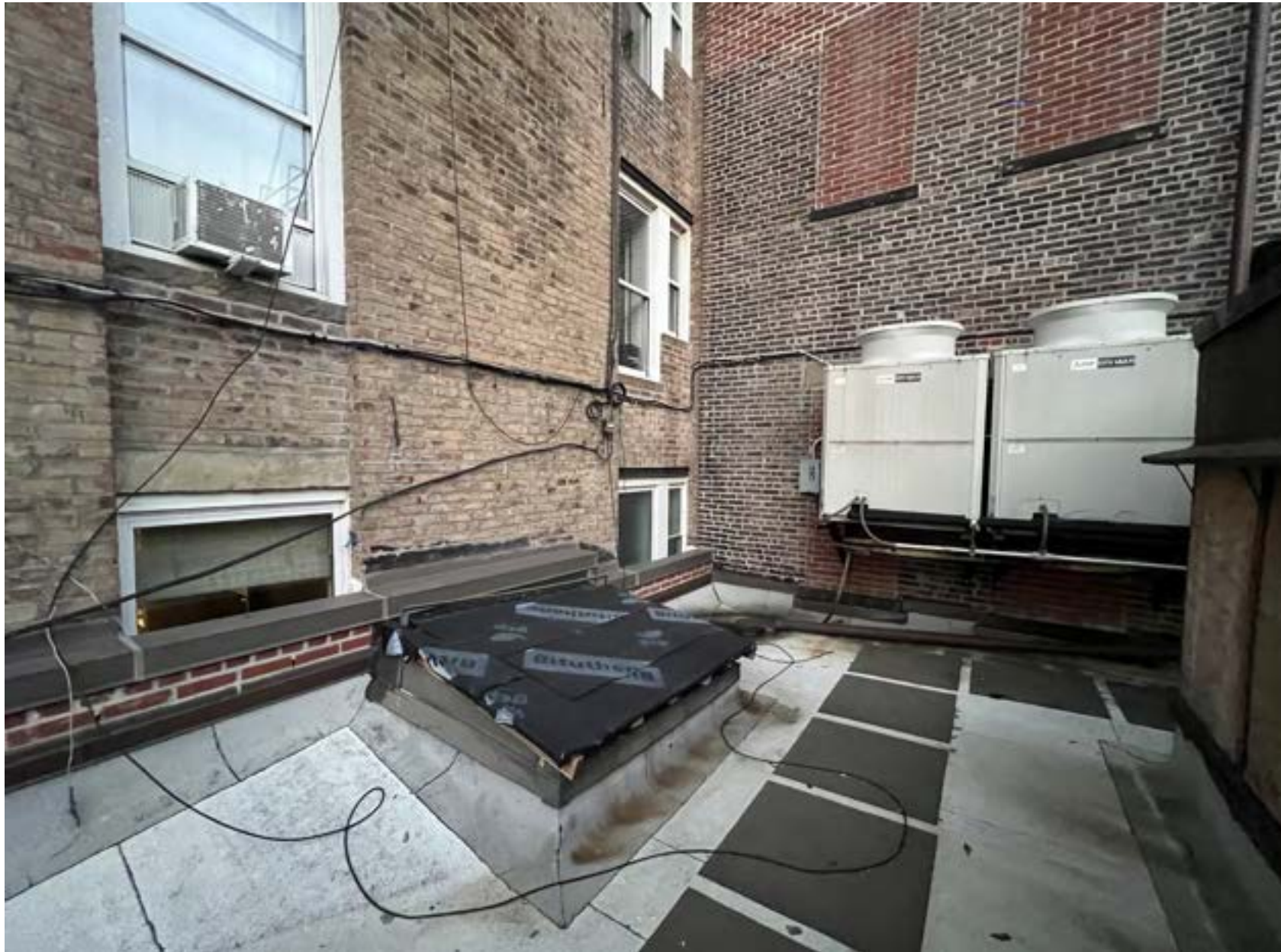
OVERVIEW OF EXISTING SKYLIGHT
