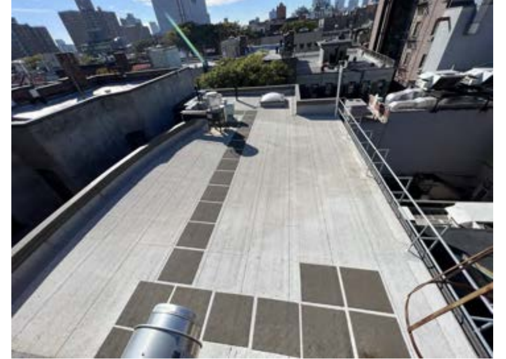
OVERVIEW OF 5TH FLOOR ROOF
