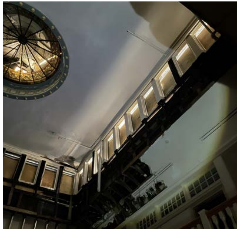
INTERIOR / EXISTING CLERESTORY WINDOWS
