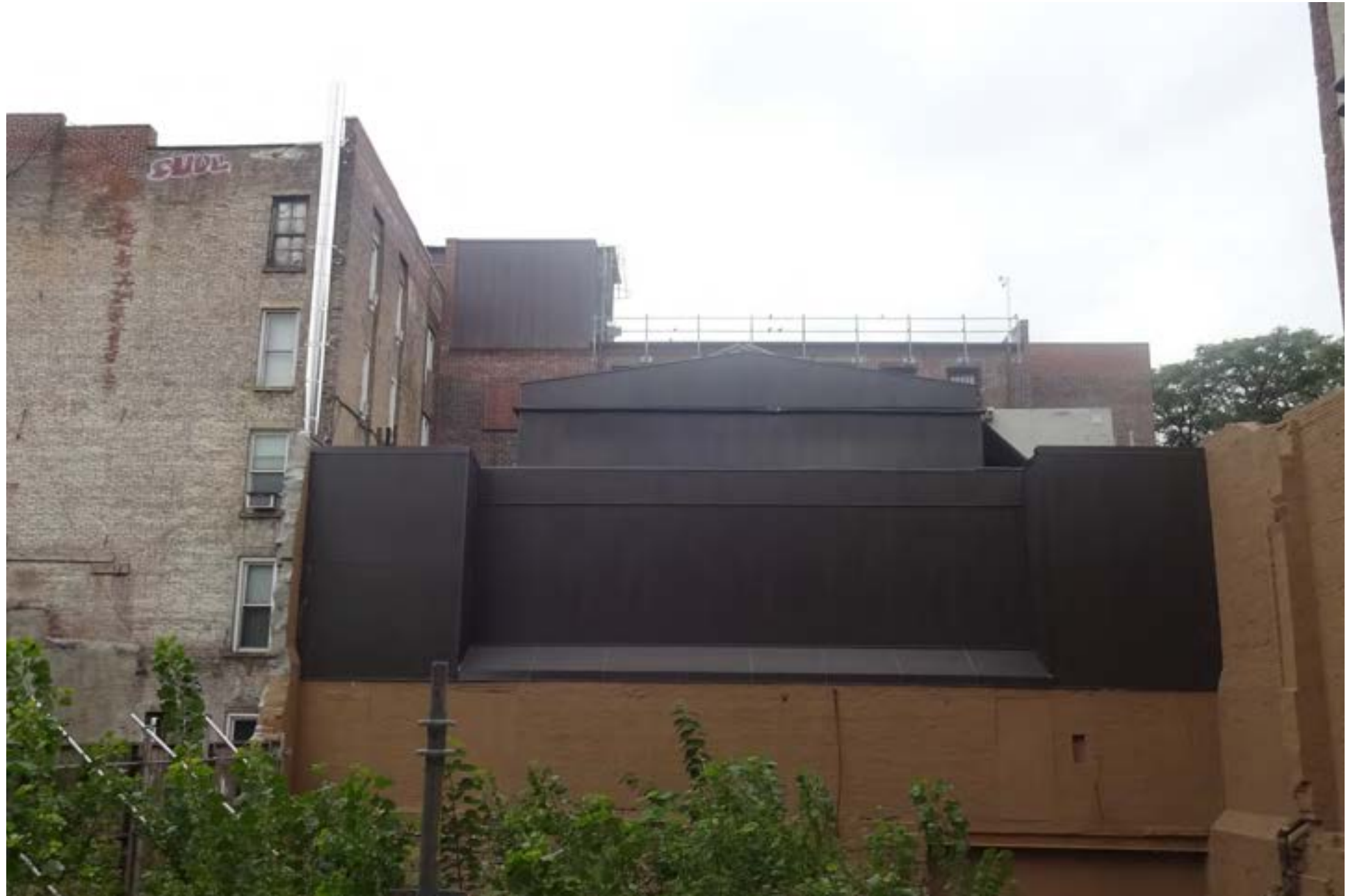
OVERVIEW OF WEST ELEVATION
