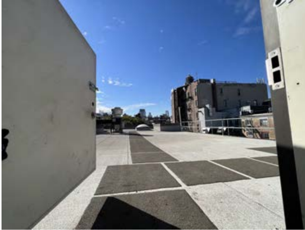
OVERVIEW OF 5TH FLOOR ROOF
