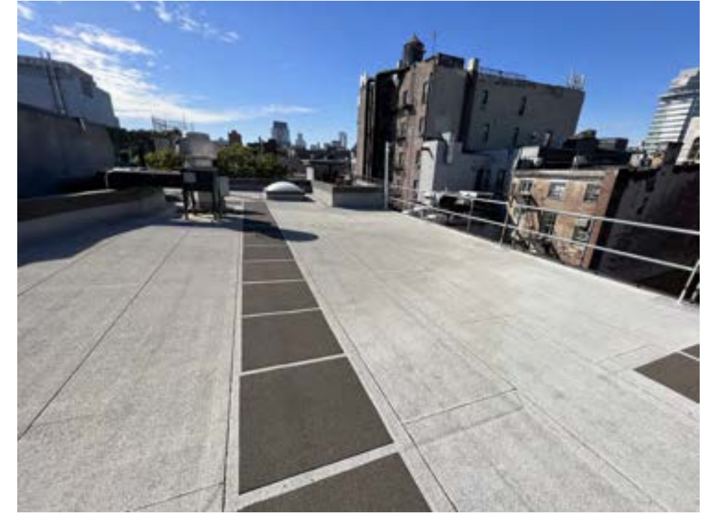
OVERVIEW OF 5TH FLOOR ROOF
