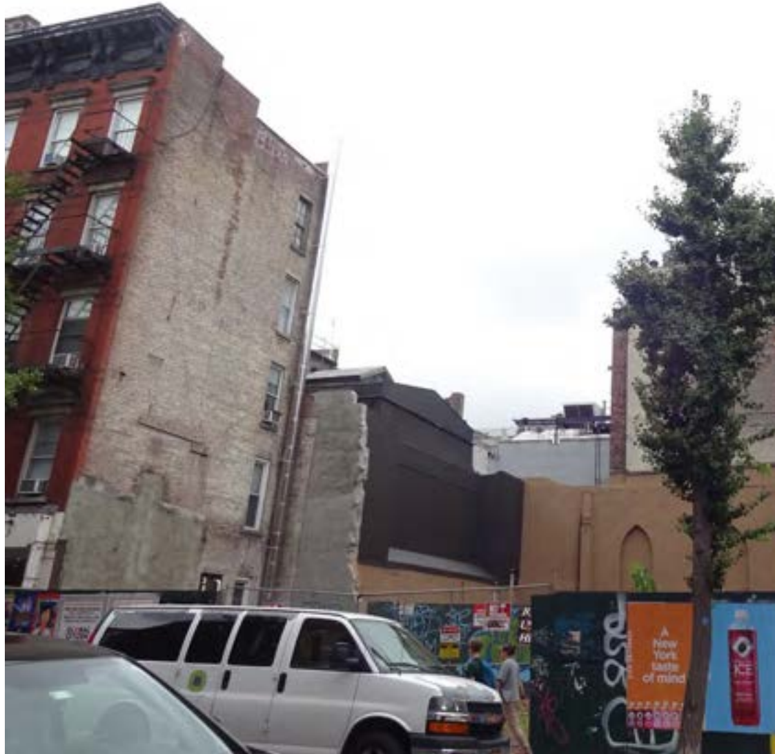
OVERVIEW OF WEST ELEVATION
