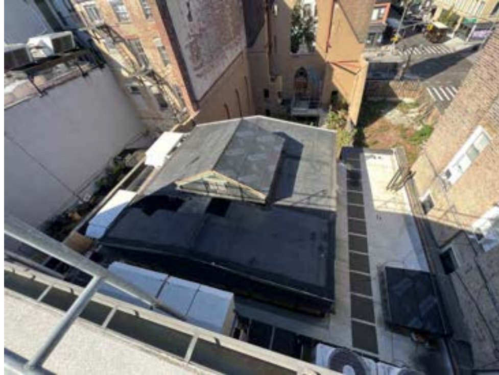
VIEW OF 3RD FLOOR / ROOF BELOW
