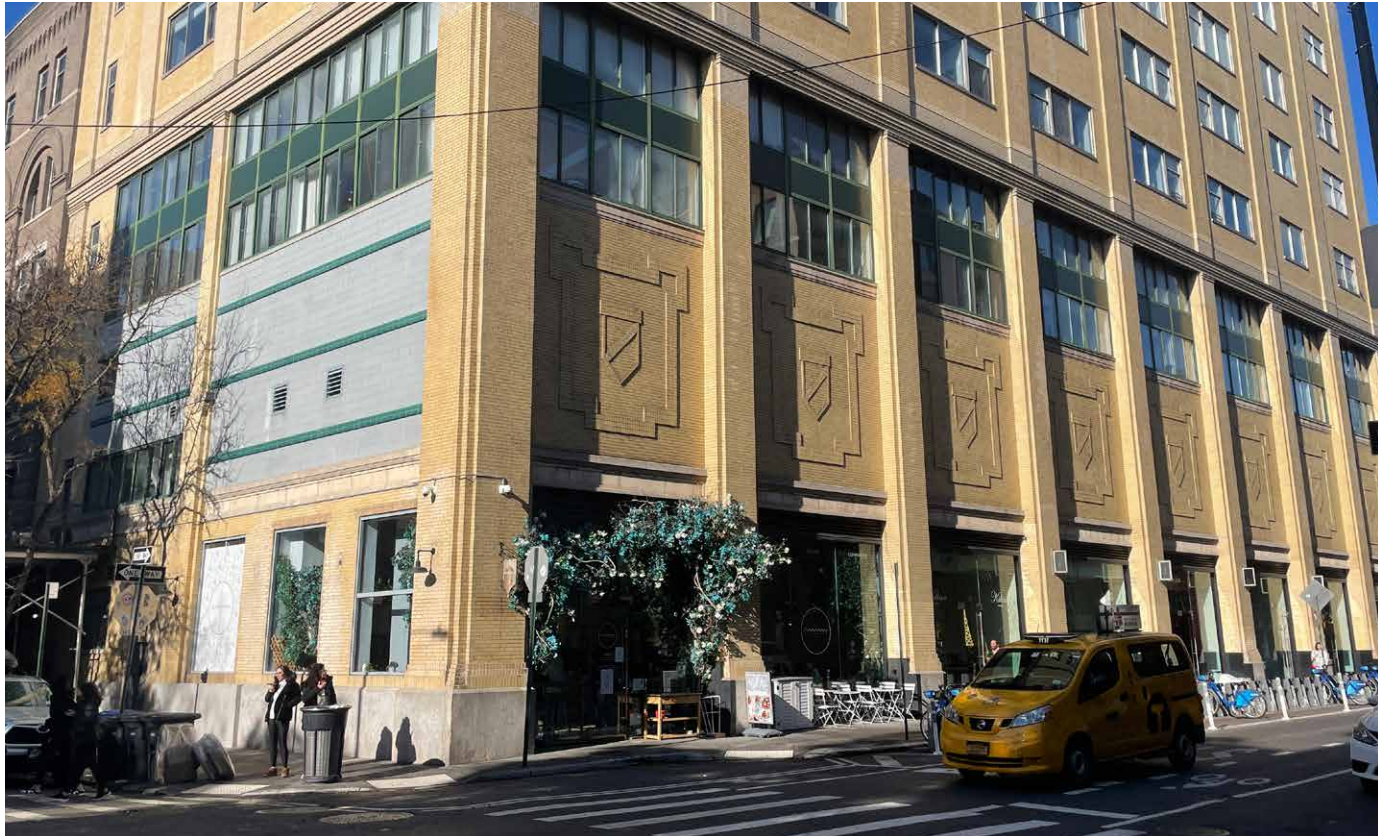
2. 808 WASHINGTON ST. (DIRECTLY NORTH WEST)
