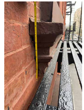
Existing Stone Header and Sill Profiles
