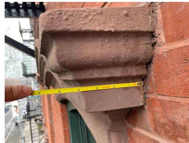
Existing Stone Header and Sill Profiles
