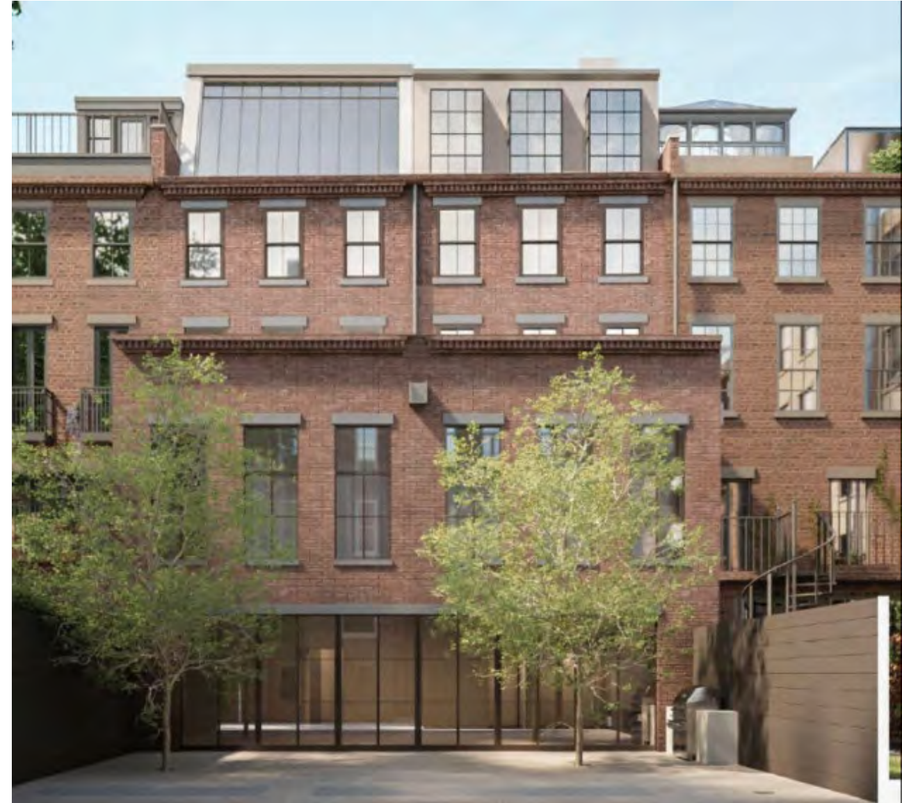
79-81 CHARLES STREET STUDIO WINDOW ADDITION APPROVED IN 2022
