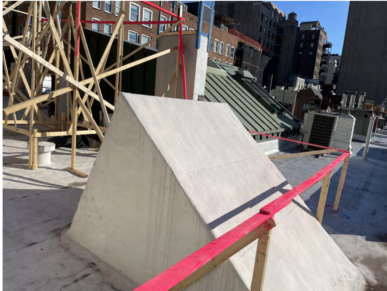
LOOKING EAST FROM FRONT GUARDRAIL MOCKUP
