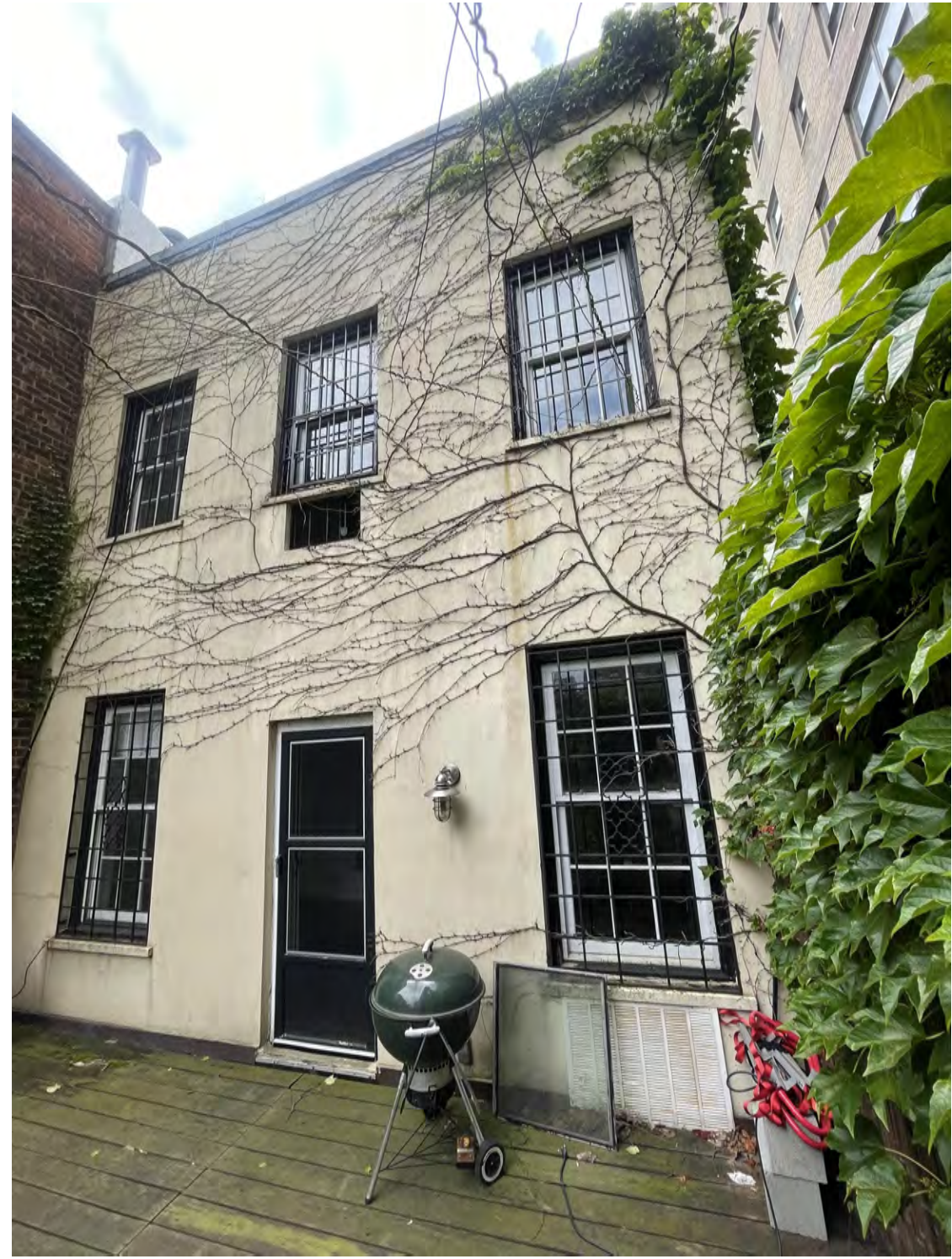
LEVEL 2 AND LEVEL 3 - REAR FACADE
