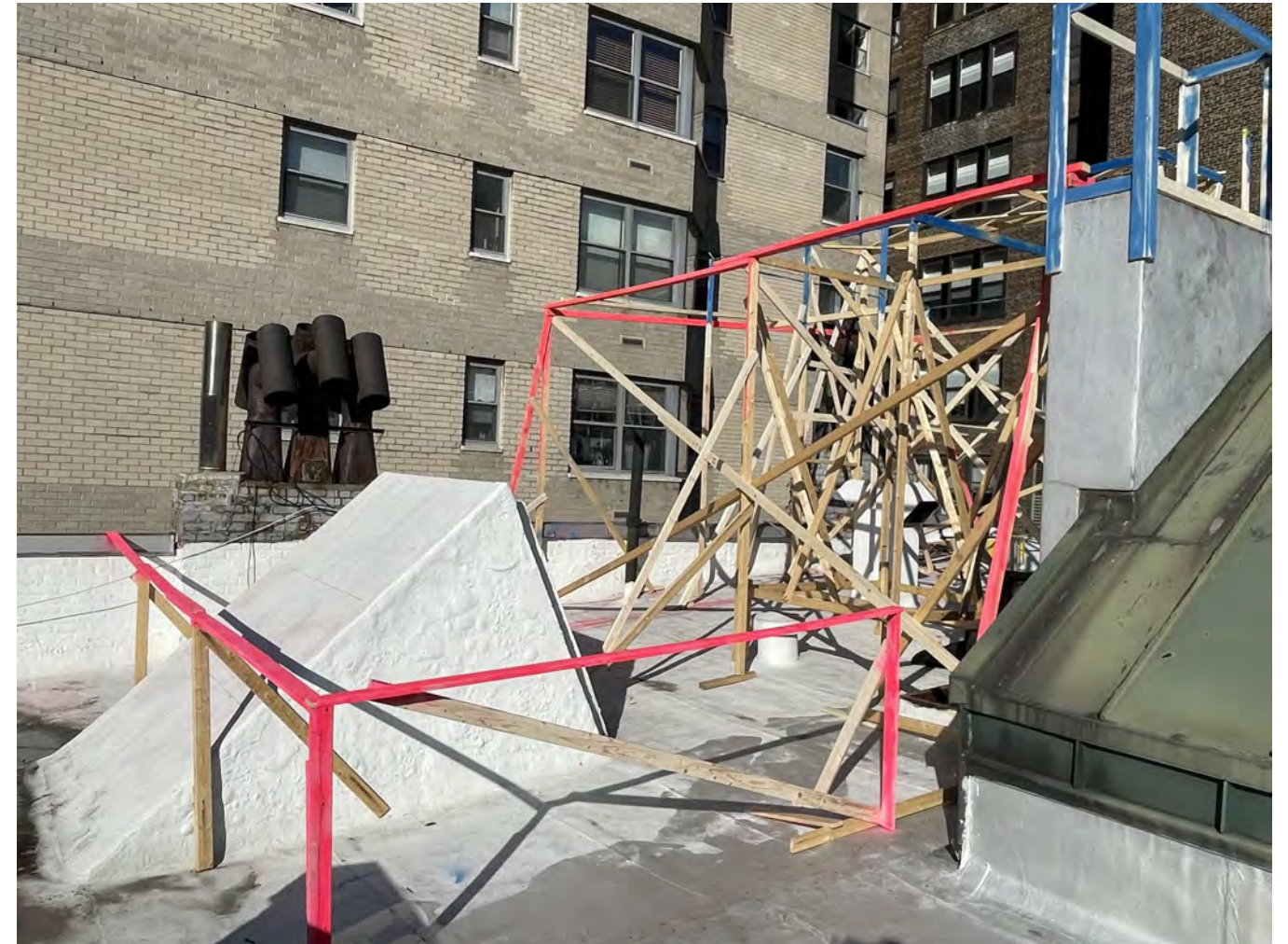
LOOKING WEST FROM FRONT GUARDRAIL MOCKUP
