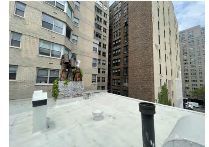
LOOKING WEST FROM PROPERTY LINE
