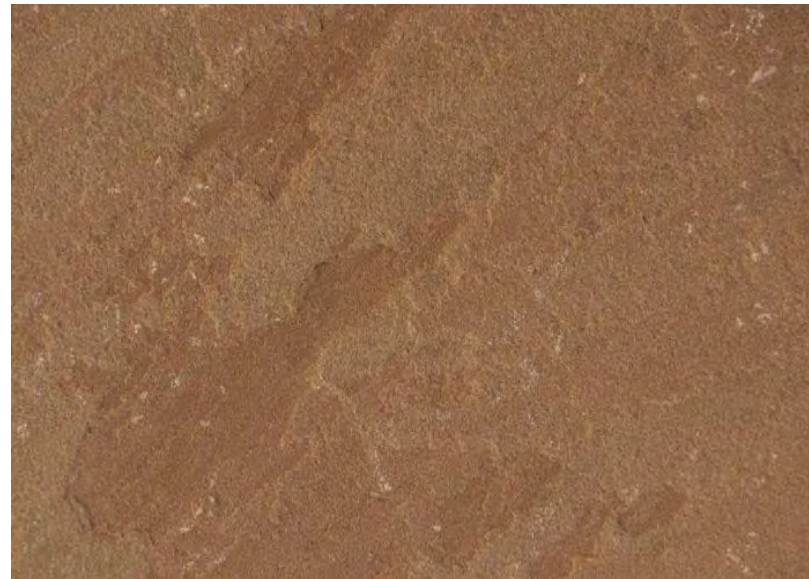
(EXISTING) BROWNSTONE EXTERIOR STONE; MATCHING BROWNSTONE STUCCO TO BE USED FOR PATCHING LOCATIONS
