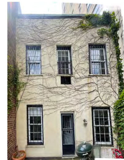
EXISTING REAR VIEW (FROM REAR TERRACE)
