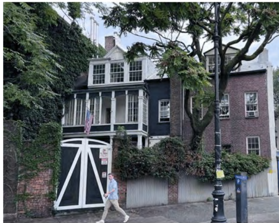
18 COMMERCE STREET REAR TEA PORCH IN 1914 (ABOVE) AND IN 2023 (BELOW) WITH 1920 COLONIAL REVIVAL ALTERATION
