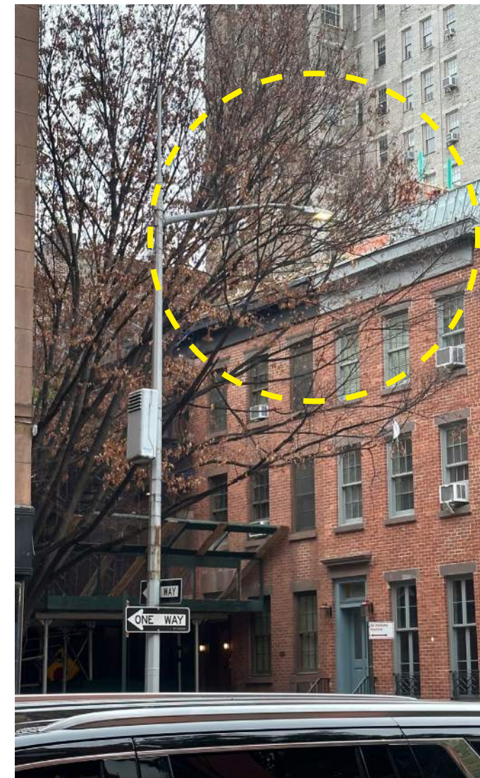
3b Railing and Bulkhead seasonally visible Front Chimney flues visible outside of trees
