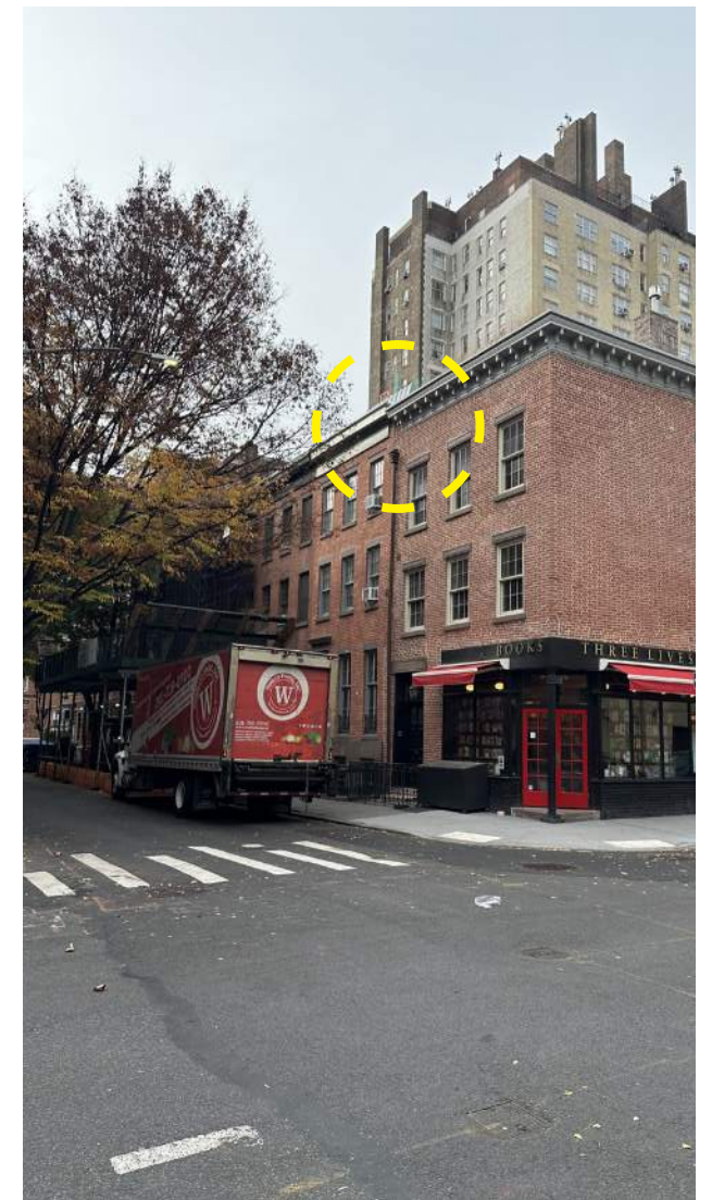
3c Front Chimney and flues partly visible
