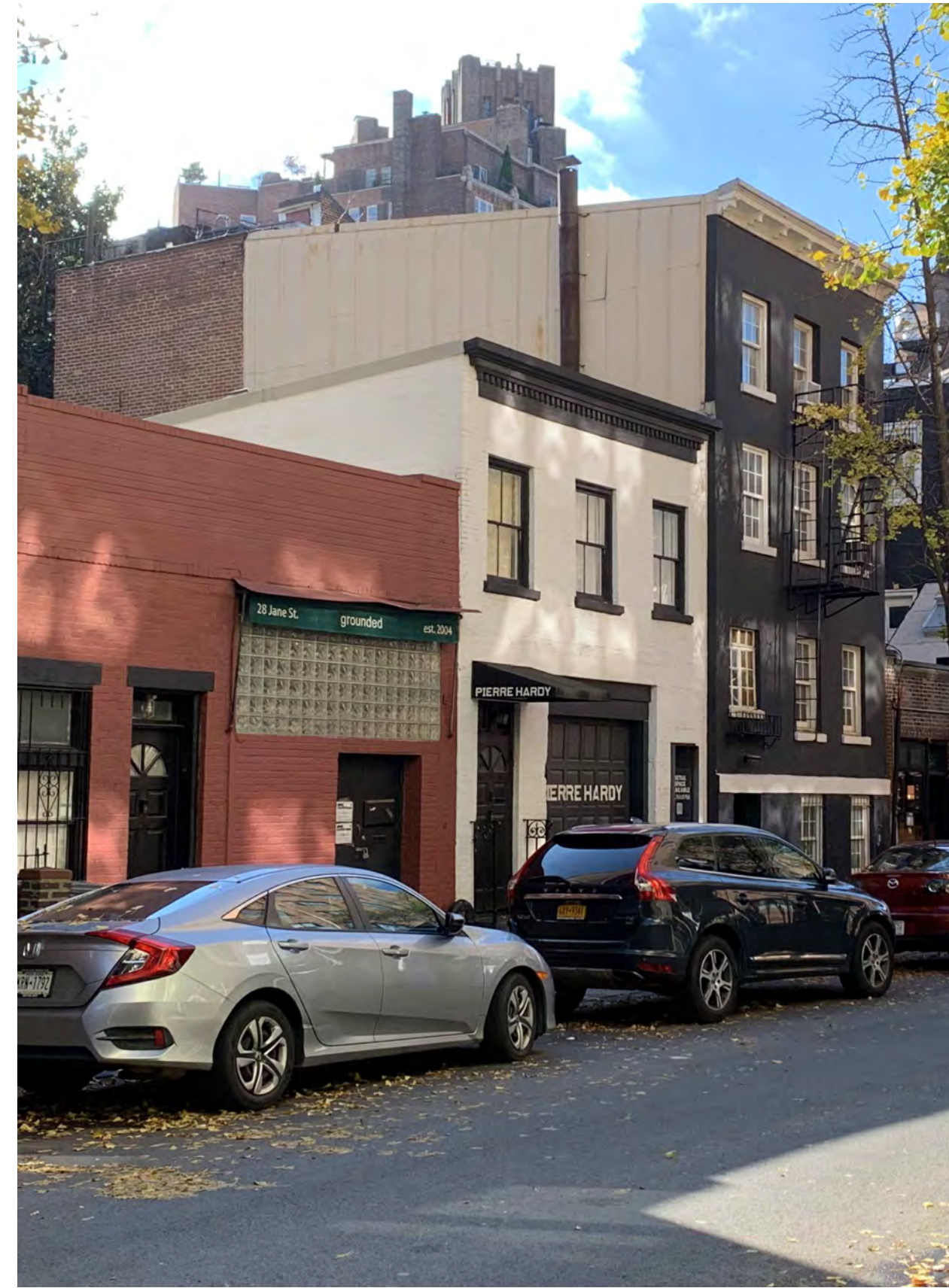
PHOTO 32 JANE ST. EAST FACADE N.T.S.
