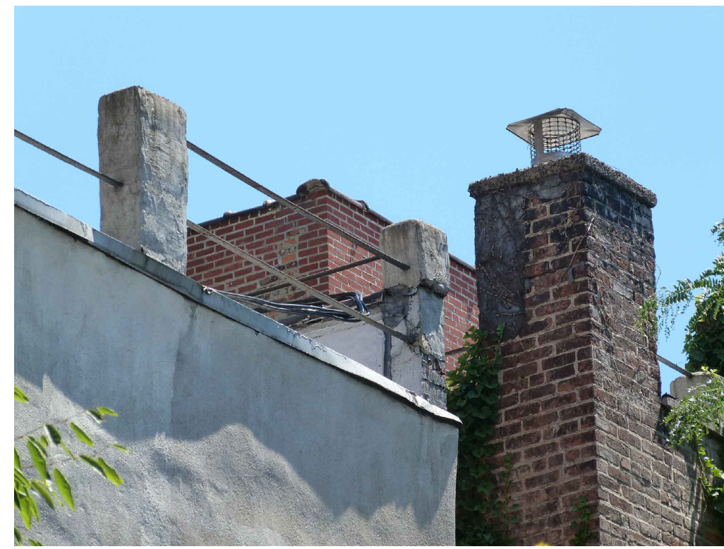
PHOTO 32 JANE ST. WEST FACADE CHIMNEY DETL. N.T.S.
