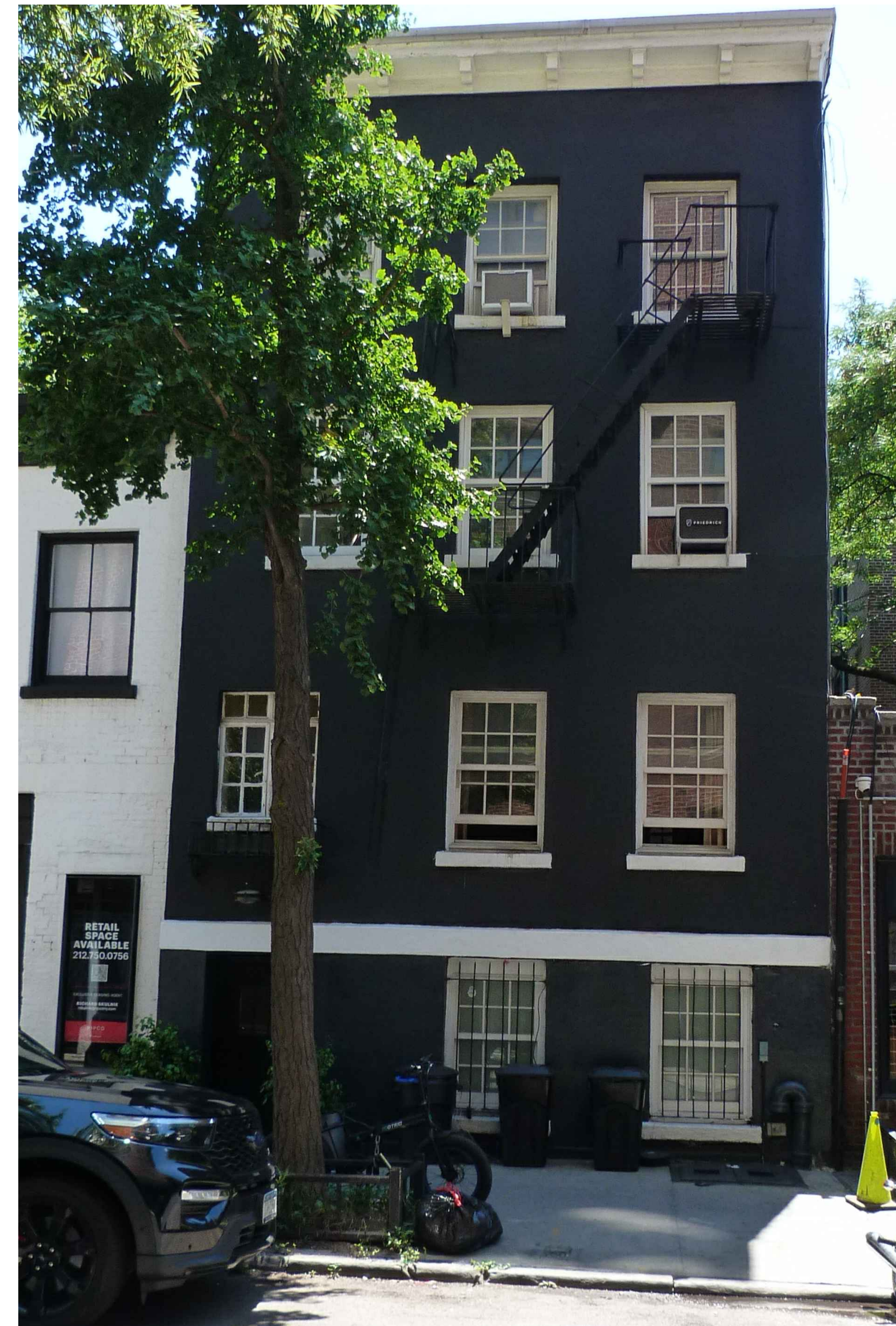
PHOTO EXISTING FACADE 32 JANE ST. N.T.S.
