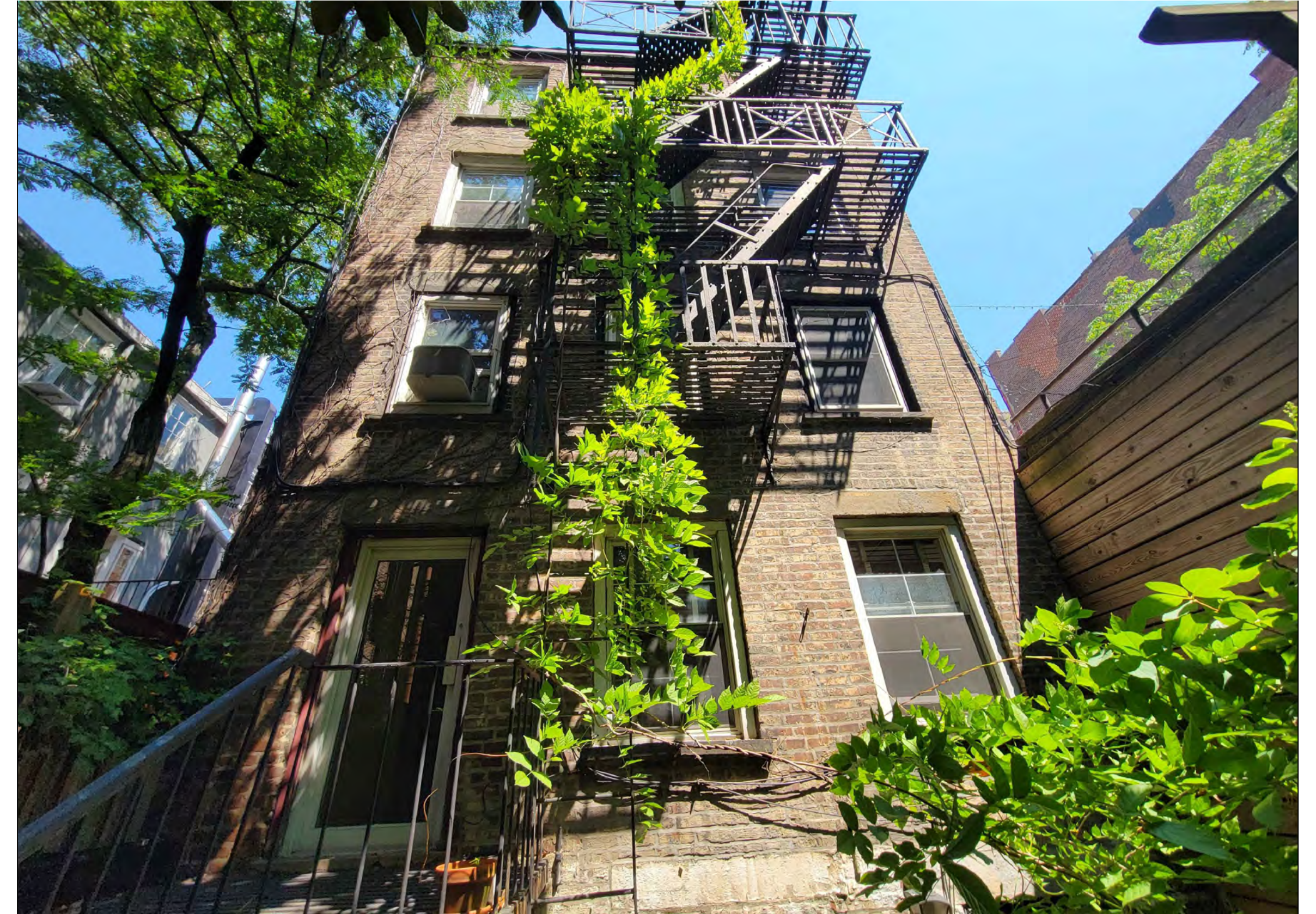
3 PHOTO: EXISTING REAR FACADE N.T.S.
