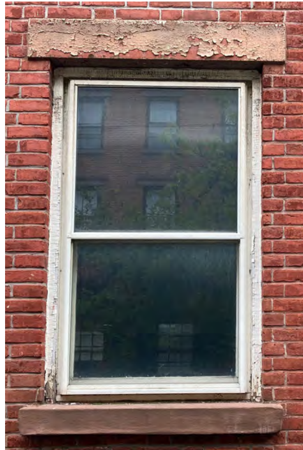
front and rear existing windows replace existing to match (white finish) Restore existing window sills and headers
