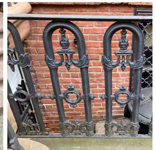
restore original railing, paint black
