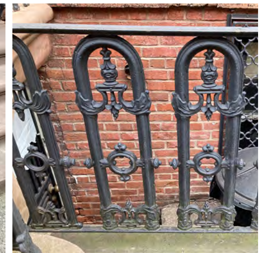
restore original railing, paint black
