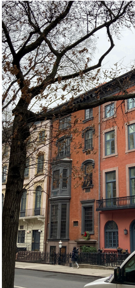
Location 4 Taken from 12 West 9th Street
