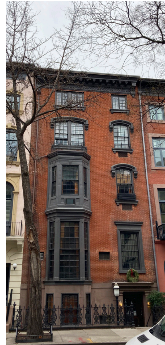
Location 3 Taken from 18 West 9th Street
