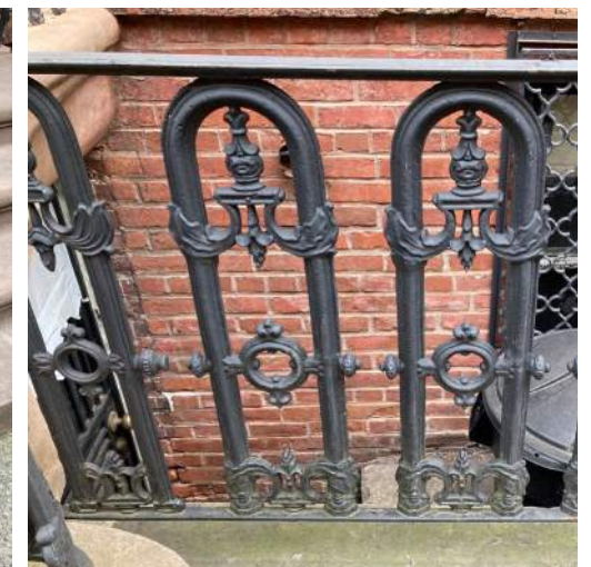
restore original railing, paint black
