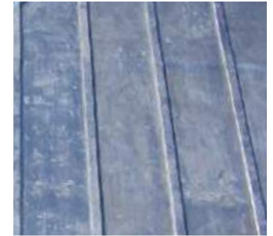
penthouse facade lead coated copper standing seam
