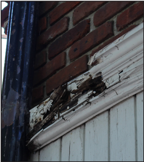
DETERIORATED FIRST FLOOR WOOD PANELING
