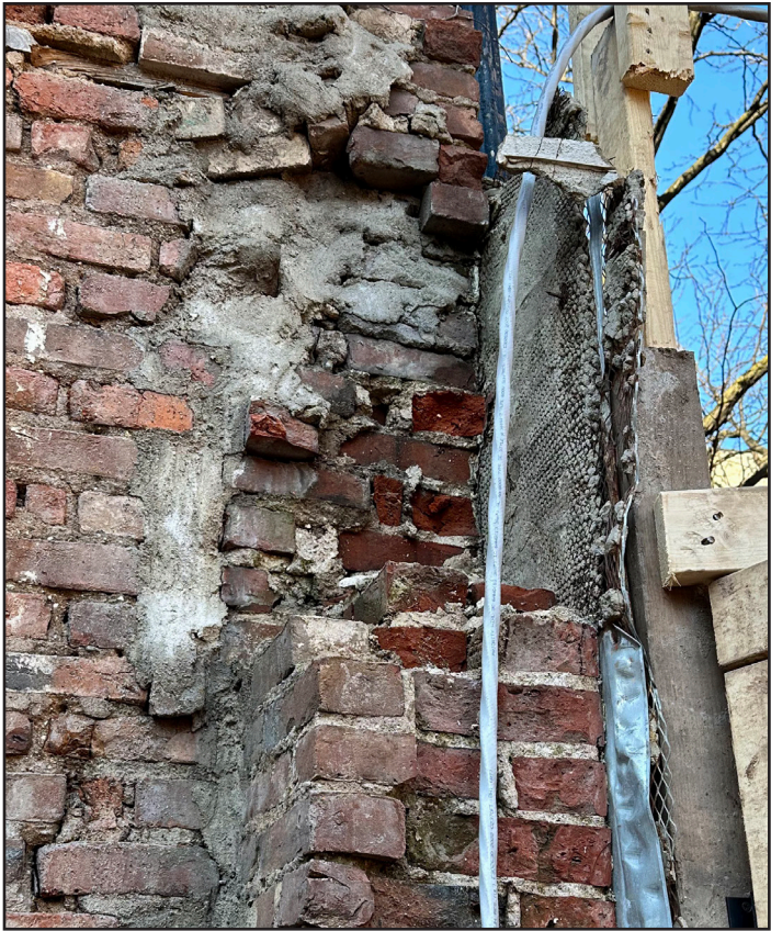
SIDE PROBE SHOWING REPLACED BRICK FACADE
