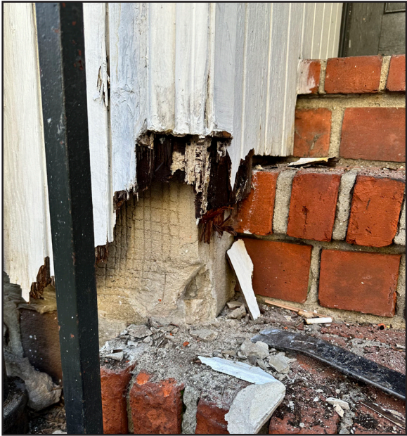
WOOD CLADDING PROBE REVEALING CEMENT INFILL
