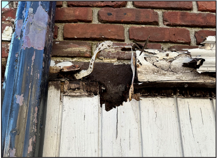
WOOD CLADDING PROBE REVEALING ORIGINAL BROWNSTONE LINTEL
