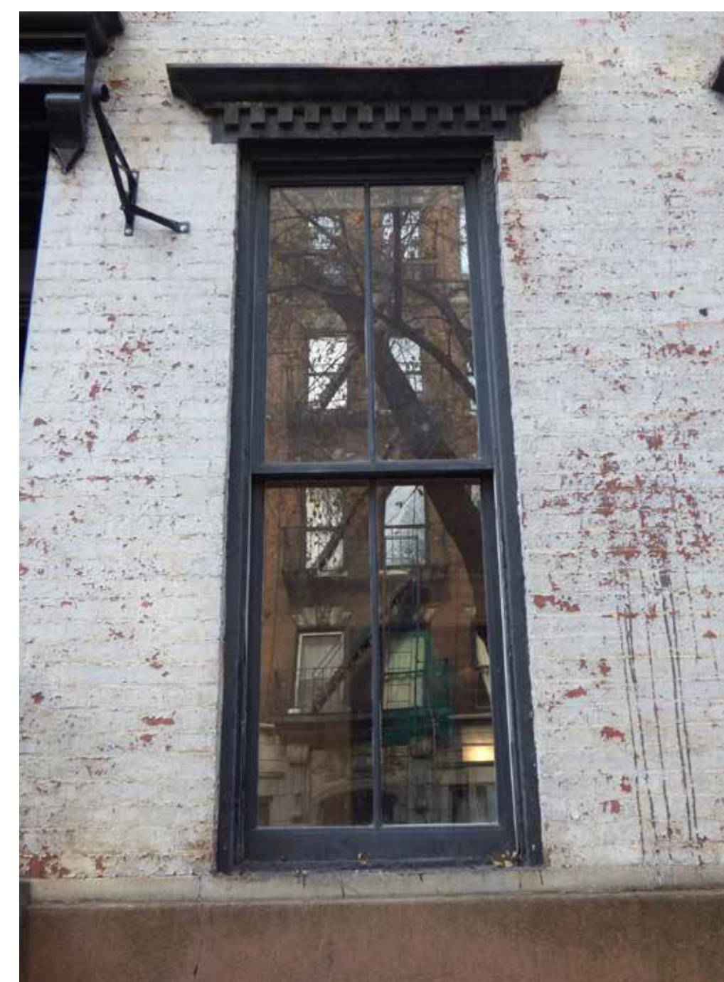
PARLOR-FLOOR WOOD, TWO-OVER-TWO WINDOWS. SHEET-METAL LINTELS AND PAINTED BROWNSTONE SILL COURSE.
