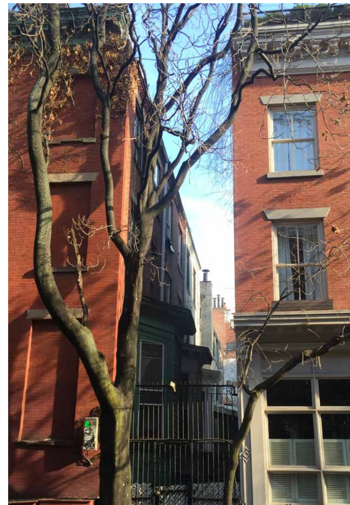
VIEW FROM WEST 4TH STREET, LOOKING EAST
