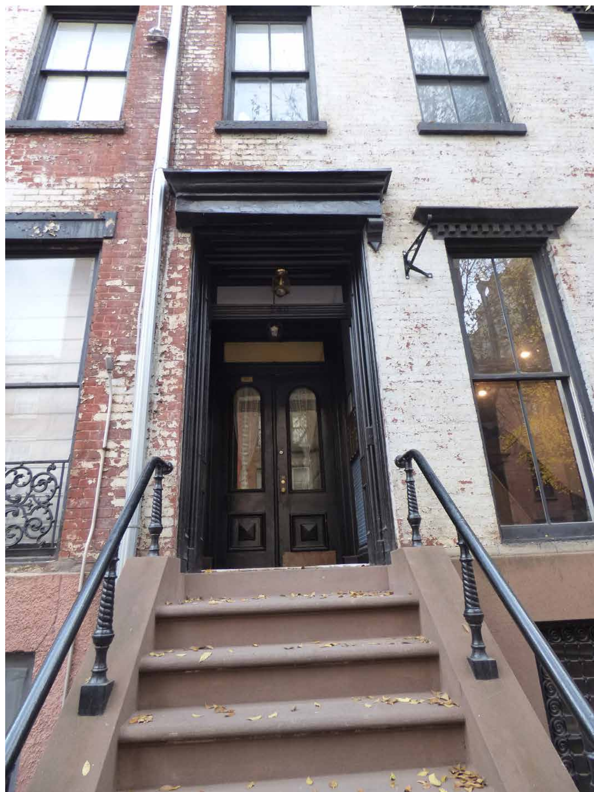
FRONT ENTRANCE WITH RECESSED DOORS. STOOP RAILING LIKELY DATES TO LATE 19TH CENTURY.
