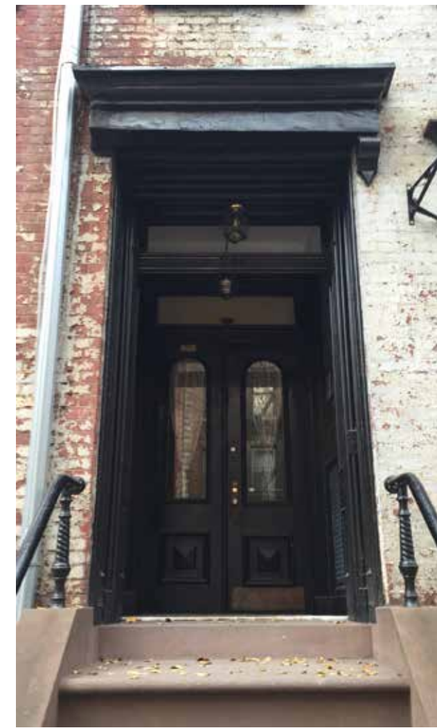
EXISTING FRONT DOOR AT 246 WEST 11TH STREET
