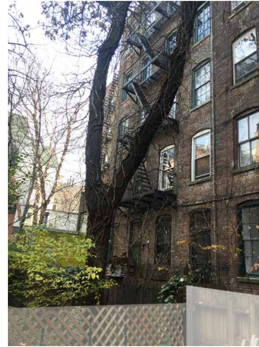
REAR COURTYARD - VIEW SOUTH
