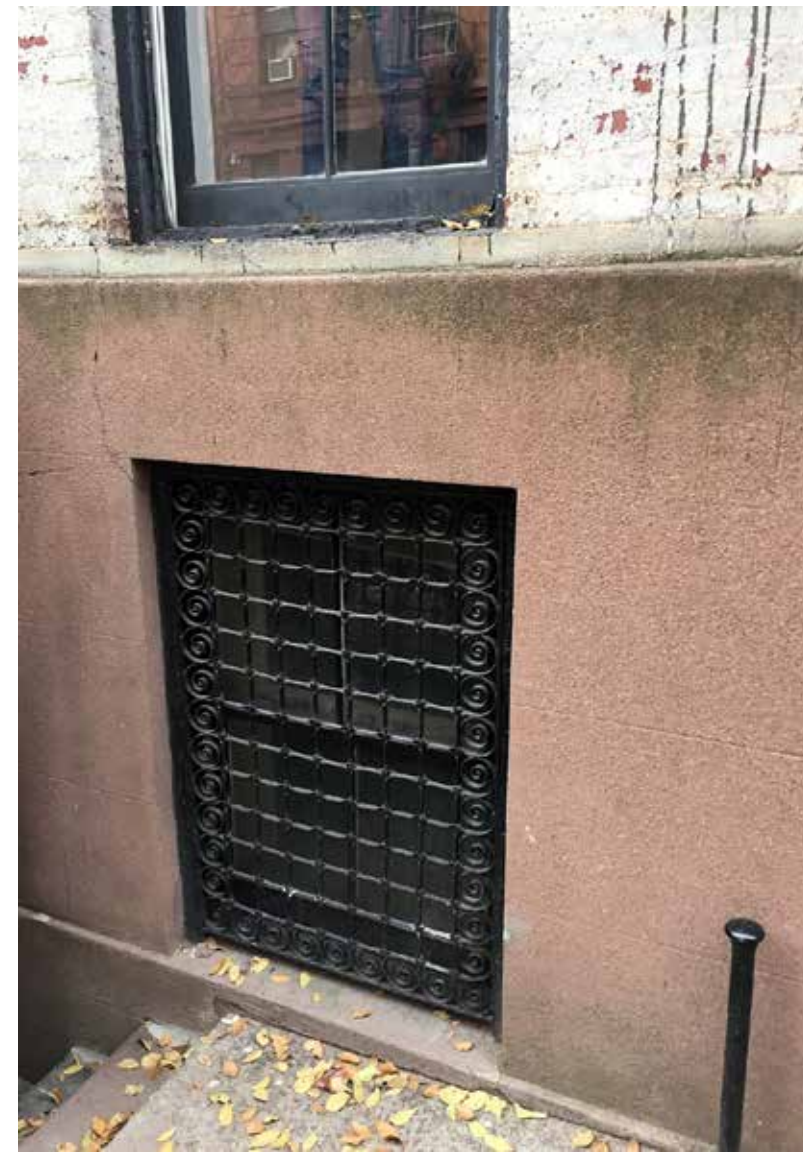
EXISTING GARDEN LEVEL WINDOW GRATES AT 246 WEST 11TH STREET TO BE REMOVED AND WINDOW SILLS TO BE LOWERED
