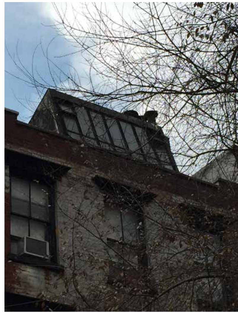
EXISTING PARAPET CAP AND SKYLIGHT AT 246 WEST 11TH STREET
