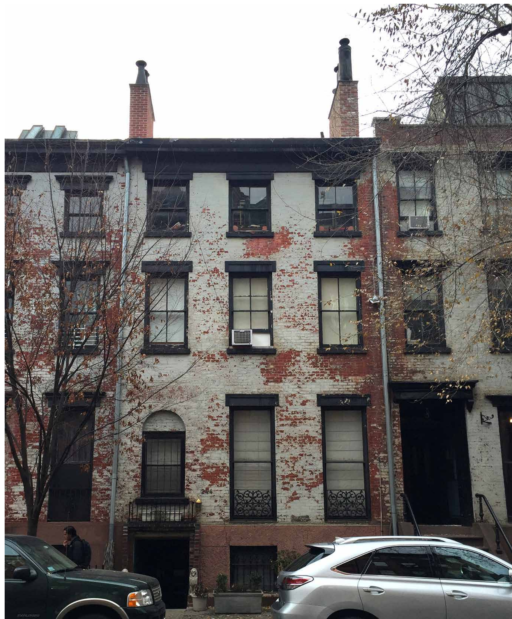
NEIGHBORING FACADE AT 244 WEST 11TH STREET
