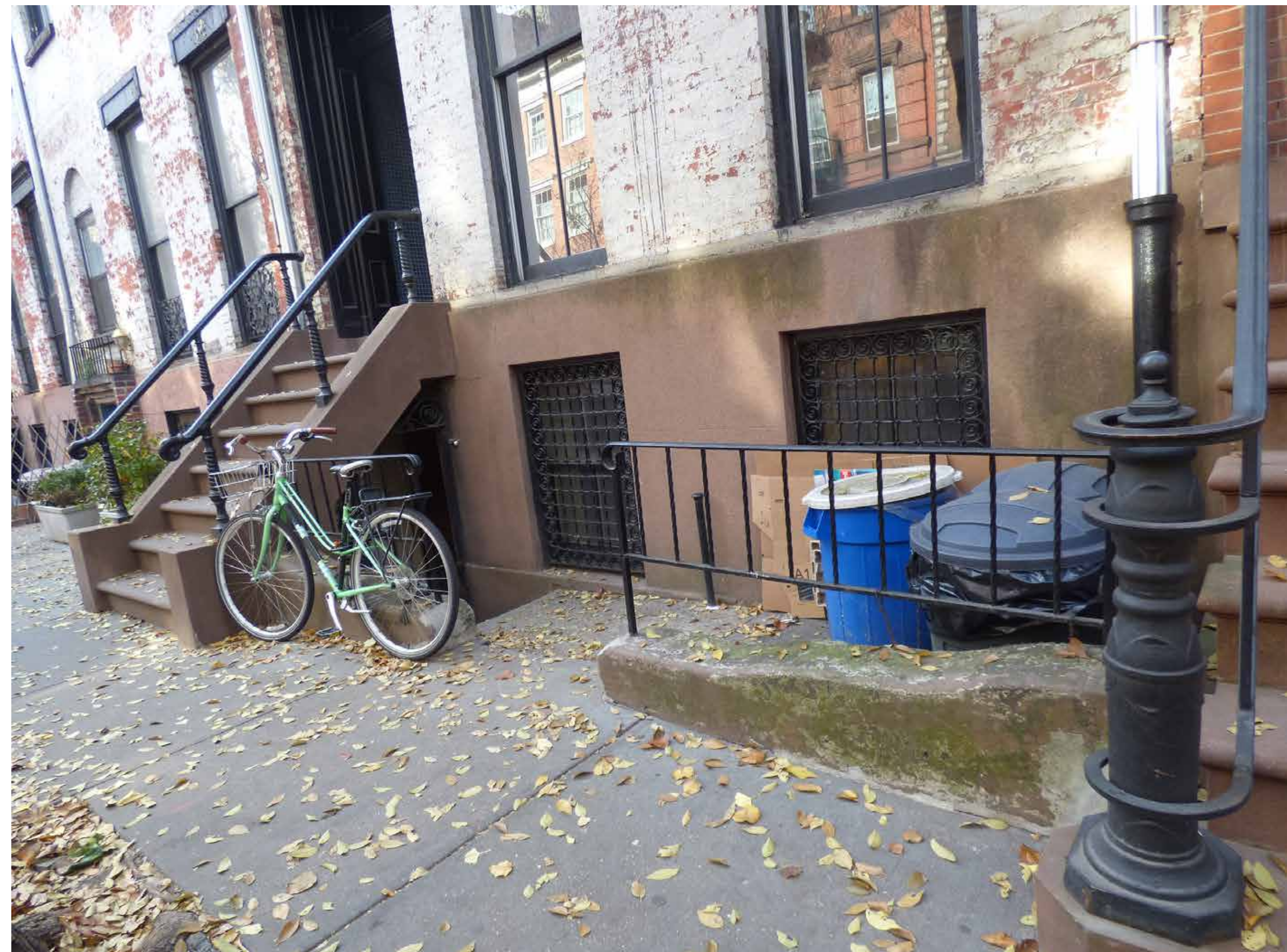
STUCCO-COVERED BROWNSTONE STOOP AND BASE. ALTERED AREAWAY.
