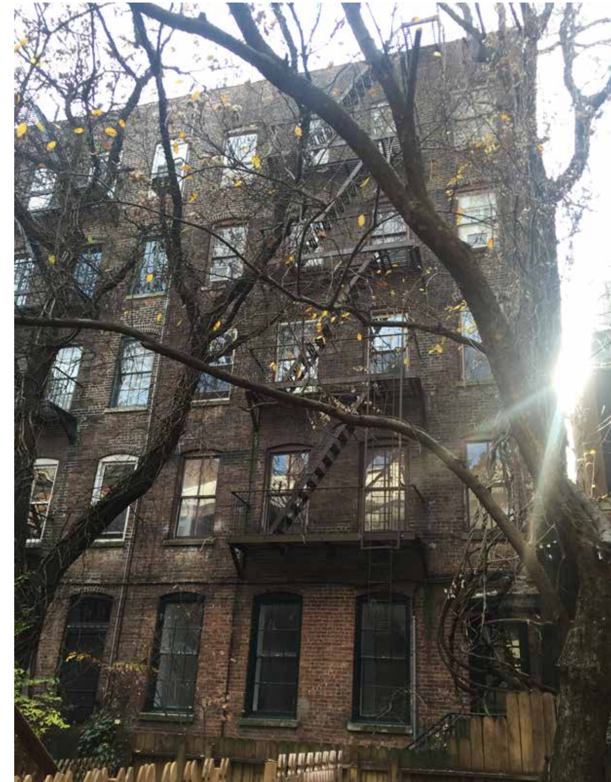
REAR YARD AT 244 WEST 11TH STREET, LOOKING SOUTH
