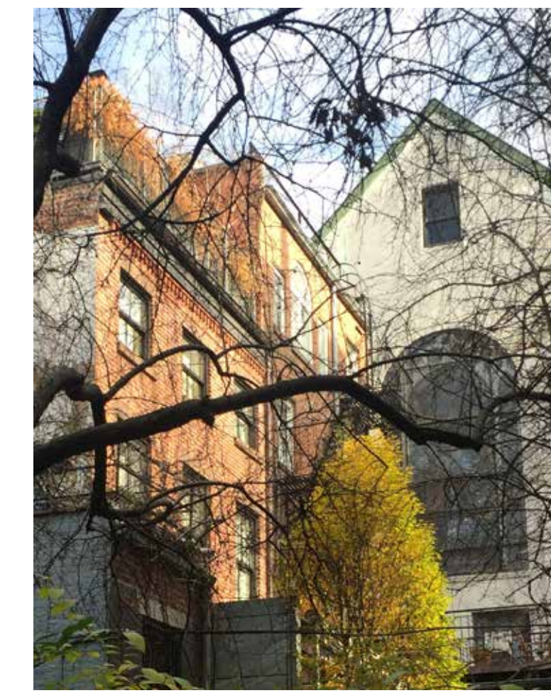
PRECEDENT OF REAR BRICK FACADE AT 240 WEST 11TH STREET
