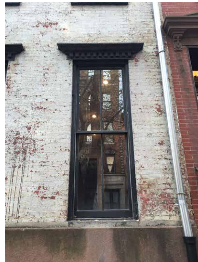
EXISTING WINDOW SILLS AND LINTELS AT 246 WEST 11TH STREET
