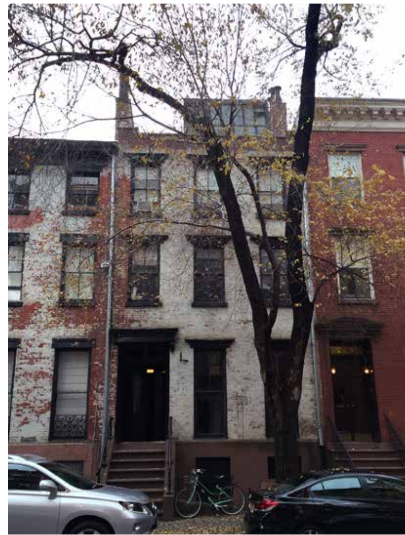
EXISTING FACADE AT 246 WEST 11TH STREET
