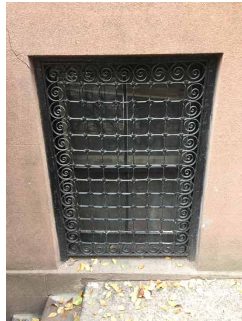
EXISTING WINDOW GRATE AT 246 WEST 11TH STREET
