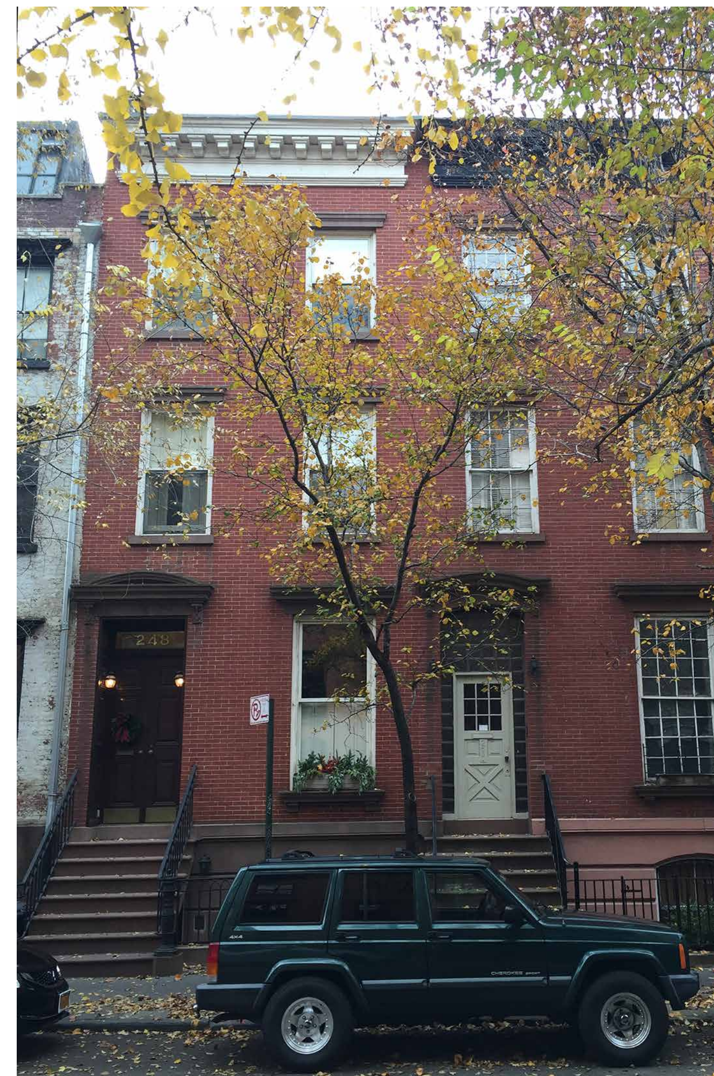
NEIGHBORING FACADE AT 248 WEST 11TH STREET
