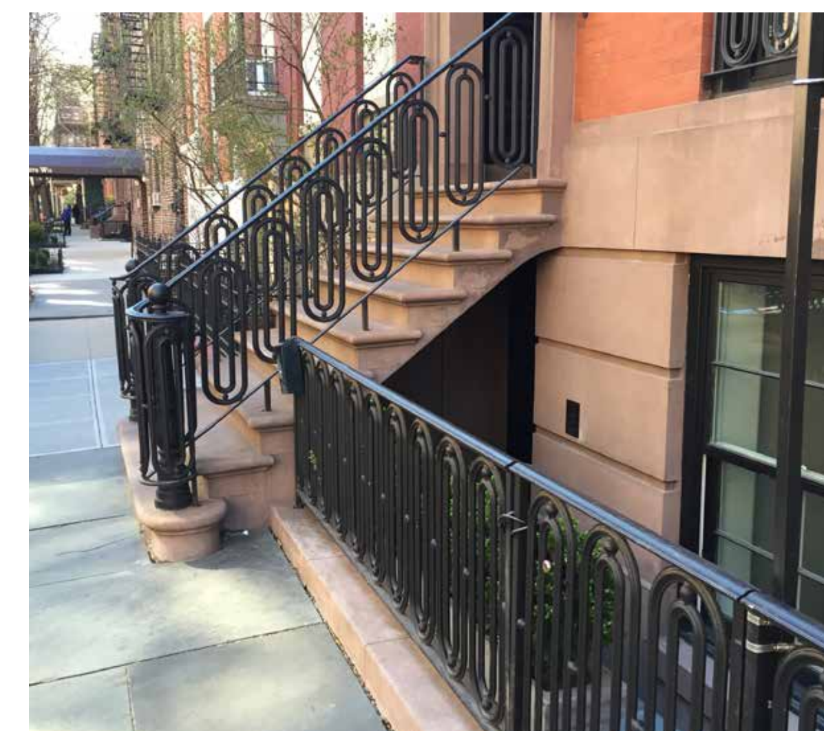
RAILING PRECEDENT AT 278 WEST 11TH STREET
