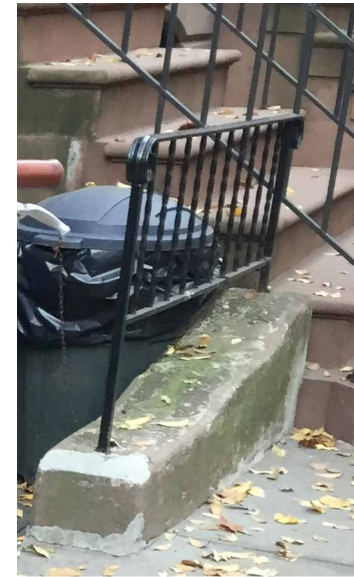
EXISTING RAILING AT 246 WEST 11TH STREET TO BE REPLACED
